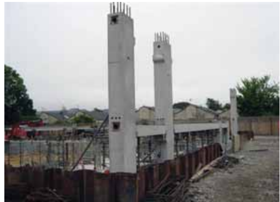
(b) PRESSS frame under construction
