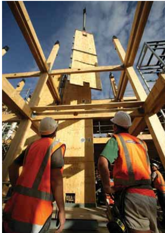
(b) Installation of prefabricated wall elements
