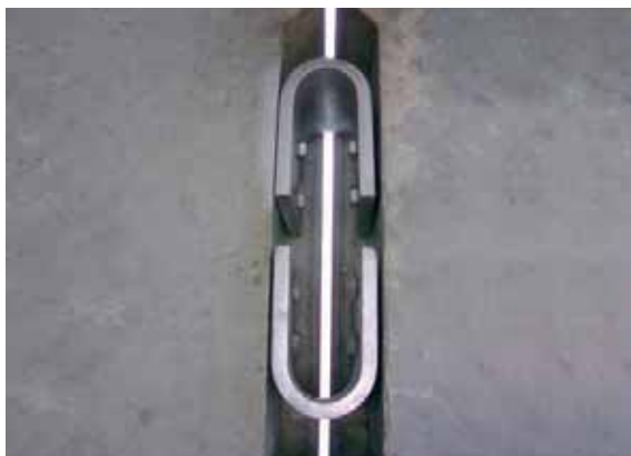
(c) U-shaped flexural plates between coupled walls
