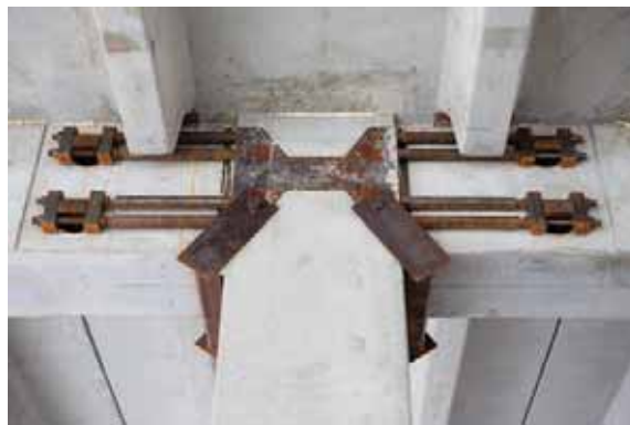
(b) Beam-column connection detail during construction
