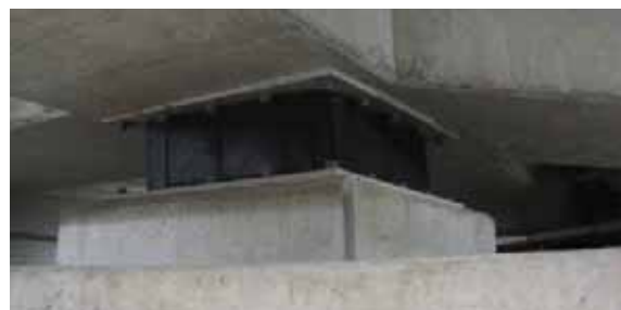
(b) Lead rubber bearing (source: Buchanan report)
