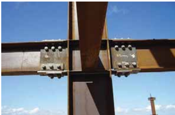
(c) Sliding hinge joints in a moment resisting frame
