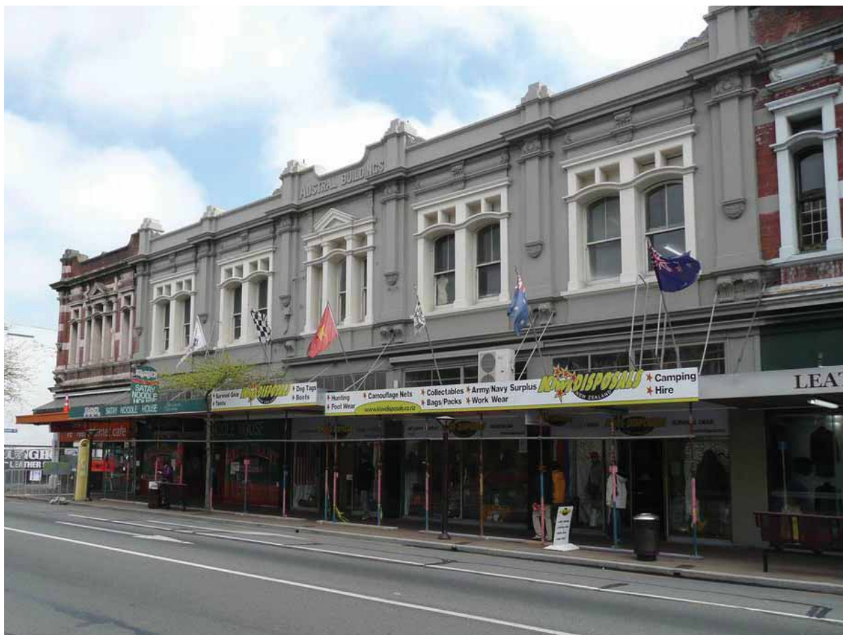
Figure 12: Former Austral Buildings, 603, 605–613 Colombo Street before the February earthquake
