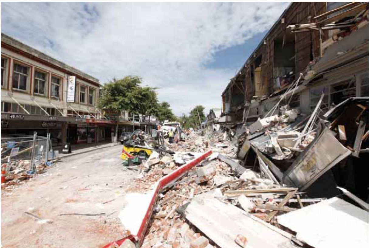
Figure 13: Former Austral Buildings, 603, 605–613 Colombo Street after the February earthquake
