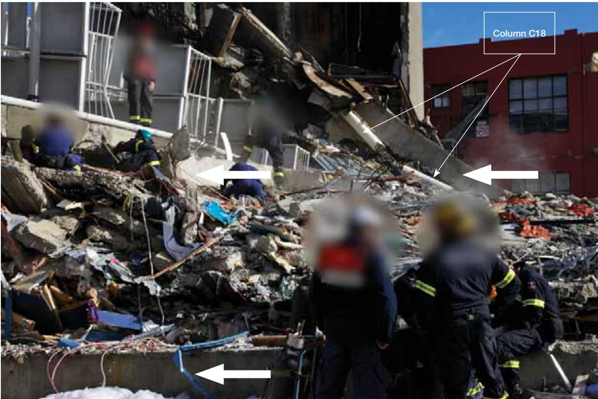
Figure 62(g): View towards the north wall complex from the south-east showing two storey-long segments of column C18 (source: Robert Heywood)
