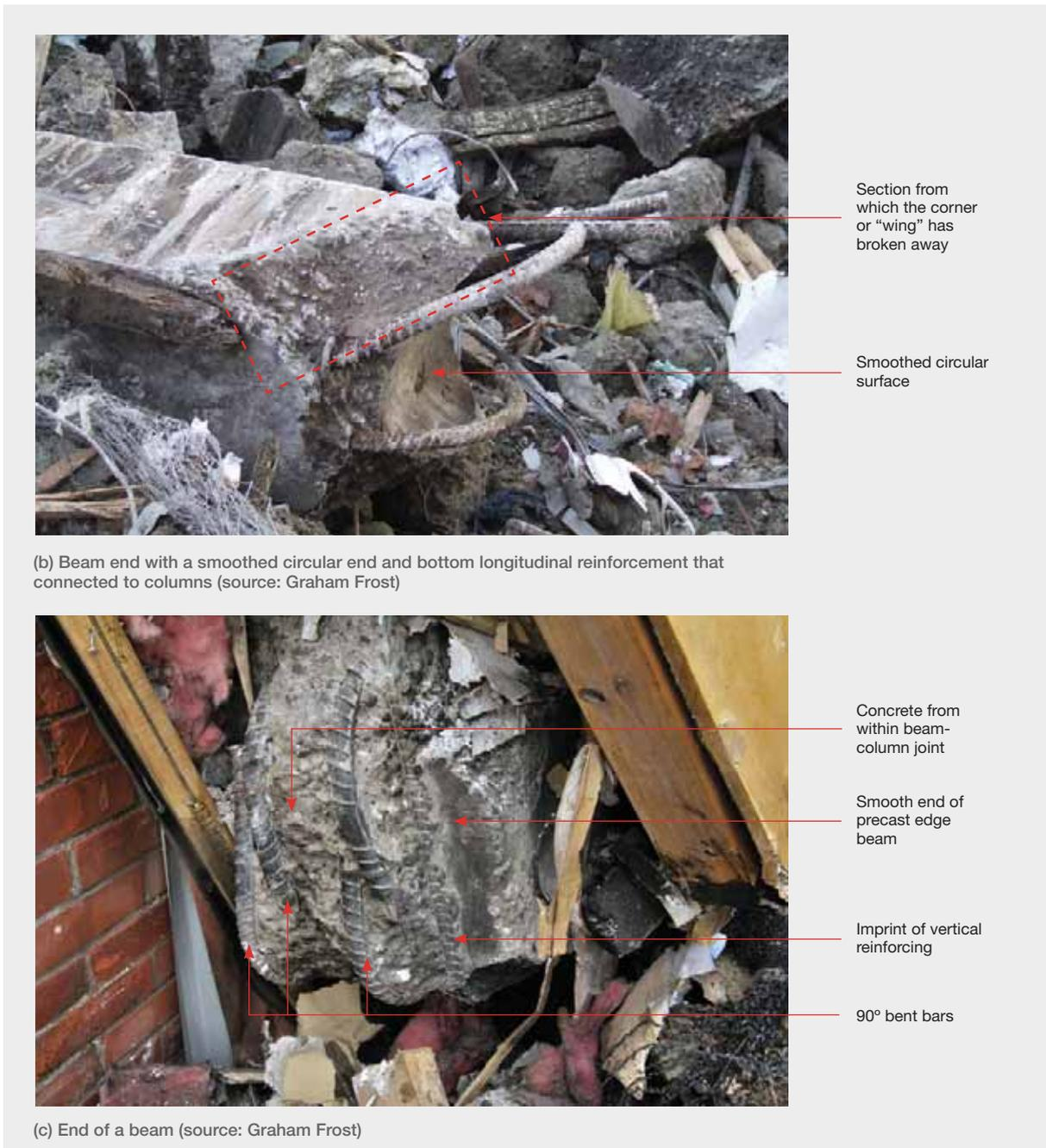
**Figure 64: Beam-column joint details**
