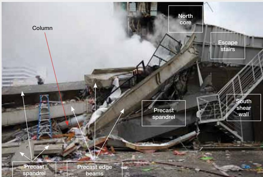
Figure 59(b): Spandrel panels and edge beams to the west of the south shear wall (source: Robert Heywood)
