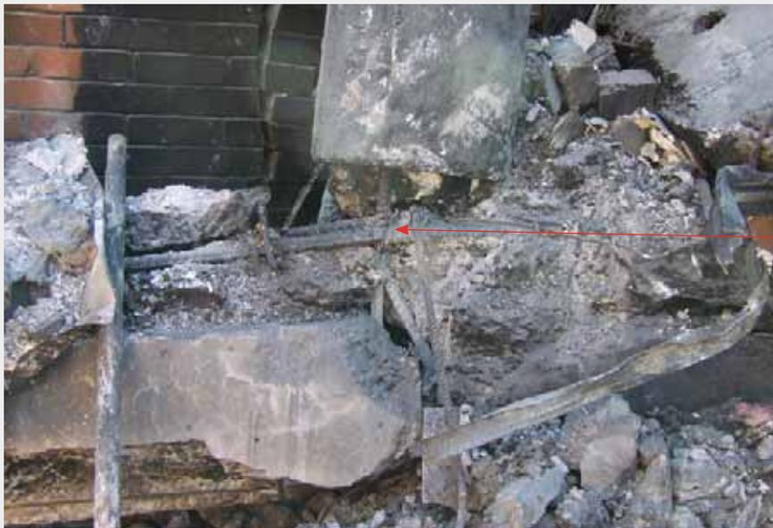
Figure 64(a): Disintegrated beam-column joint (source: Graham Frost)
