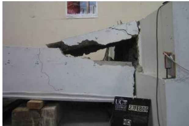
Figure 5-9: Positive moment failure of hollow-core unit (Photo from reference 7)
