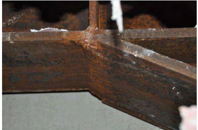
L6, Grid C2, brace weld
