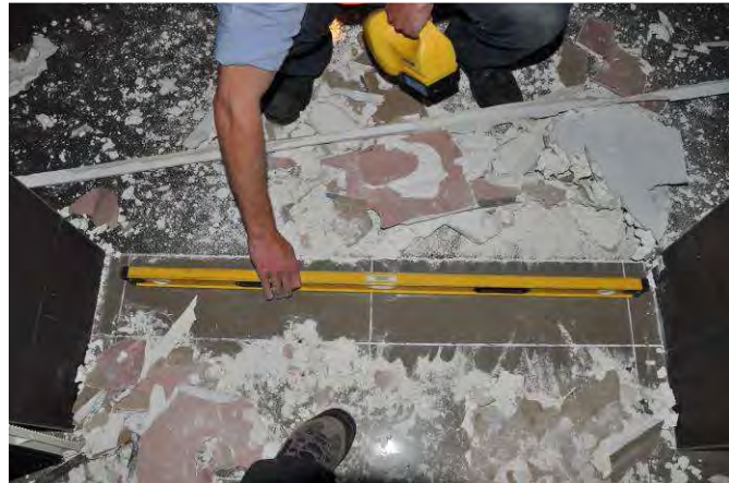
L7 floor at Grid C1/26, essentially level
