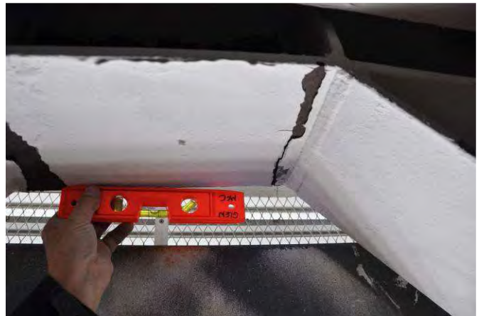
L2, Grid E½1, active link, permanent offset
