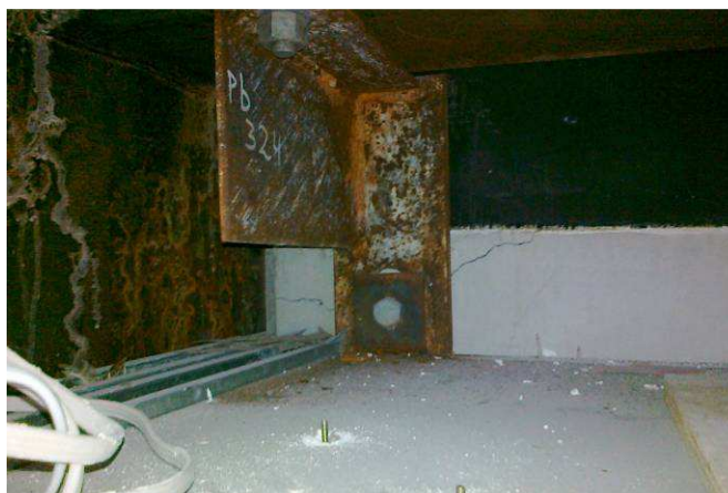
L11, Grid C2, damaged panel fixing
