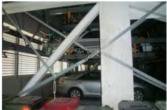
L2 Carstacker crossbraces "unhooked"
