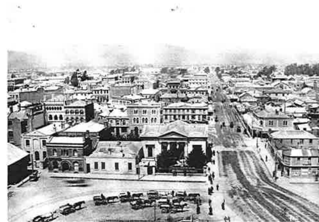
Figure 37. Christchurch in transition from wood to masonry, looking south from cathedral.
