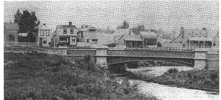
Figure 16. The second Victoria Street bridge, 1865. Probably the earliest iron-and-stone bridge in New Zealand, it is now preserved as the Hamish Hay Bridge in Victoria Square. Dr A.C. Barker photograph, CM41
