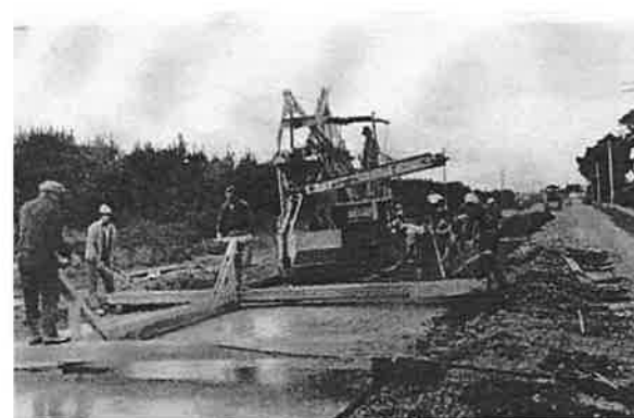
Figure 13. Road construction, Sockburn, 1930s. ATL collection
