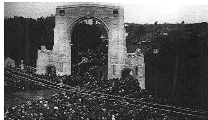
Figure 127. Opening of the Bridge of Remembrance, 11 November 1924. CMI 4572
