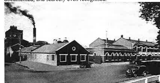
Figure 55. Brewing began on this site, on the corner of Kilmore shed and Fitzgerald Avenue, in the 1890s and continued until 1954. The buildings remain, in other uses. John Wilson private collection.
