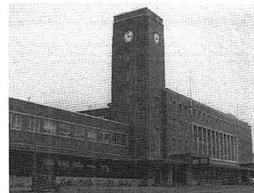
Figure 11. New Railway Station, Moorhouse Avenue, 1960. It was designed in the thirties but construction was delayed by the war. The well-proportioned brick building was obsolete within a decade, as passengers deserted the railways for motor cars and air travel. It now houses Science Alive and a cinema complex. Rice GW, p13, Christchurch Star
