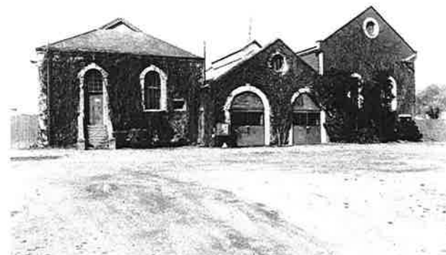
Figure 27. Old Drainage Board No.1 pumping station, now a recycling yard. J. Wilson Private collection.
