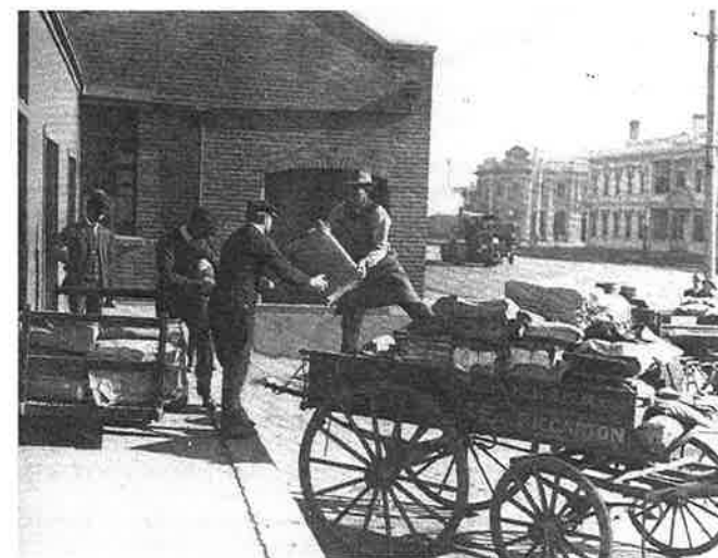
Figure 105. The Press being unloaded at the Christchurch station for rail delivery. Alexander Turnbull 40900 1/2 (press)
