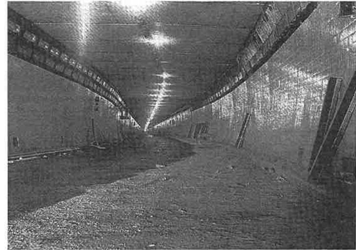
Figure 8. Road tunnel to Lyttelton nearing completion. Opened on 27 February 1964, it was designed as a toll tunnel (New Zealand's longest) but became toll-free in 1979. Christchurch Star
