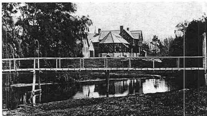
Figure 119. Antigua Street suspension bridge and a section of the original Public Hospital buildings, 1872. Lamb RC, p108, Brittenden Collection CHAC/CM
