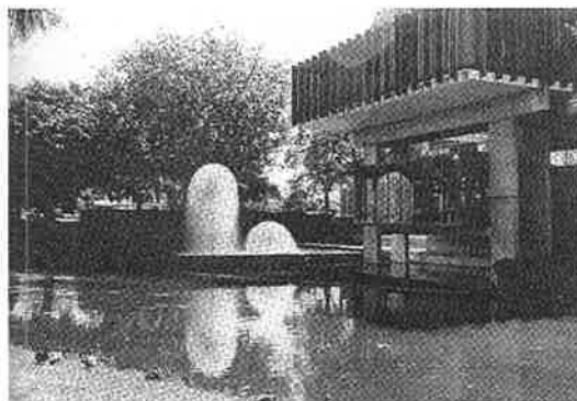
Figure 101. Part of the Christchurch Town Hall (1972) and the Ferrier fountain, viewed across the Avon from Victoria Square. Designed by Warren and Mahoney, this award-winning group of buildings has become a Christchurch icon. CM 16276
