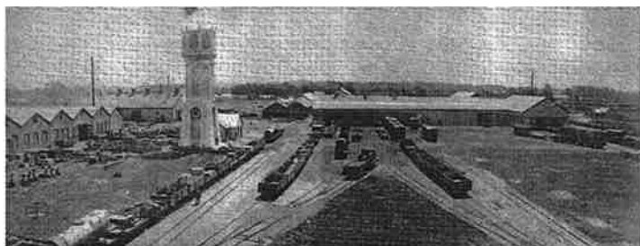
Figure 12. Addington Railway Workshops, soon after completion of the water tower (1883), one of New Zealand's earliest reinforced concrete structures. The workshops became one of the city's biggest employers in the late nineteenth century, and produced New Zealand's first locally designed steam locomotive (W192) in 1889. French collection, CHAC/CM 931
