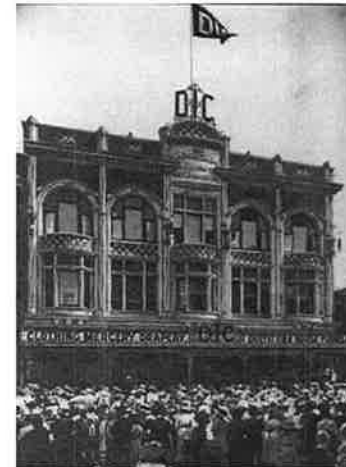
Figure 65. DIC, one of a number of departments on Cashel Street. Canterbury Museum 2495 1/4
