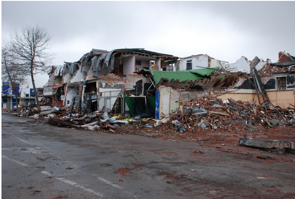
Figure 2-10 An example of the concentration of damaged URM buildings in the CBD.
