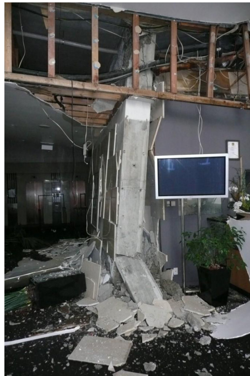
Figure 2-9 Shear wall failure in the Grand Chancellor. Failure of this wall caused the entire building to lean. (Source: Dunning Thornton, 2011)
