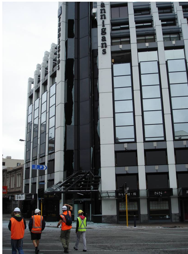
Figure 1-6 Safety assessment personnel in the Central Business District. Note the broken windows and canopy glazing. (Source: Ken Elwood)
