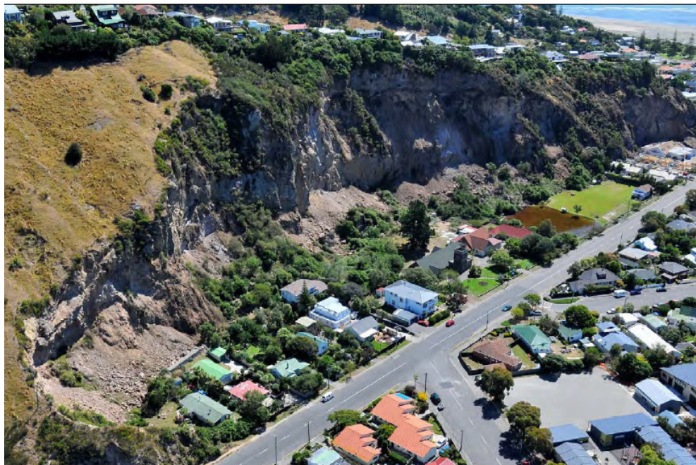
Figure 3-6 One of the cliffs in the Sumner District that experienced slides and rock falls. Note debris at bottom of cliff. (Source: GNS Science, 2011a)
