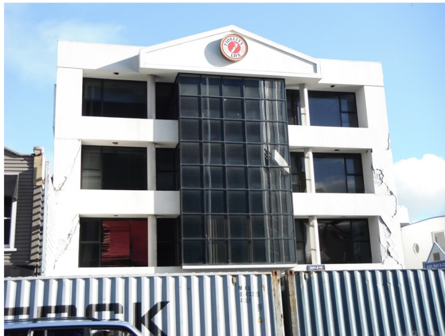
Figure 3-2 Close-up of the indicator building of Figure 3-1.
