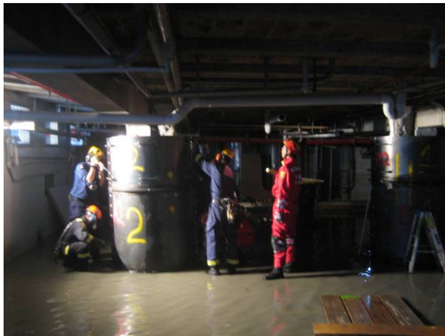
Figure 3-4 Emergency stabilization of columns. (Source: Holmes Consulting Group)
