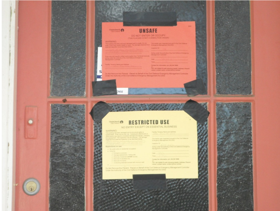
Figure 4-1 A building with two different placards. Often the older placard was not removed.
