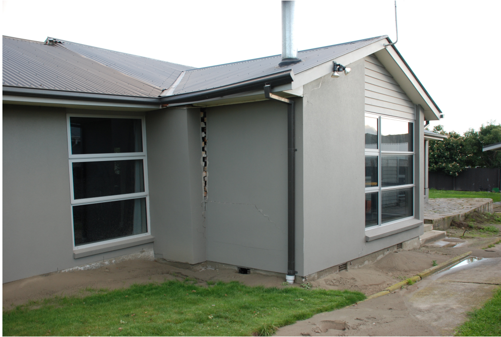
Figure 2-1 Home damaged by liquefaction. Note sand boil under window at right.
