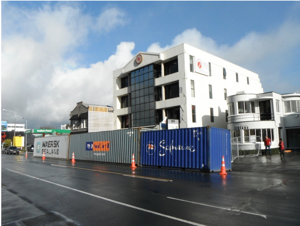
Figure 3-1 This building was used as an “indicator building” by Christchurch officials. Note the shipping containers used as barricades at the front of the building.
