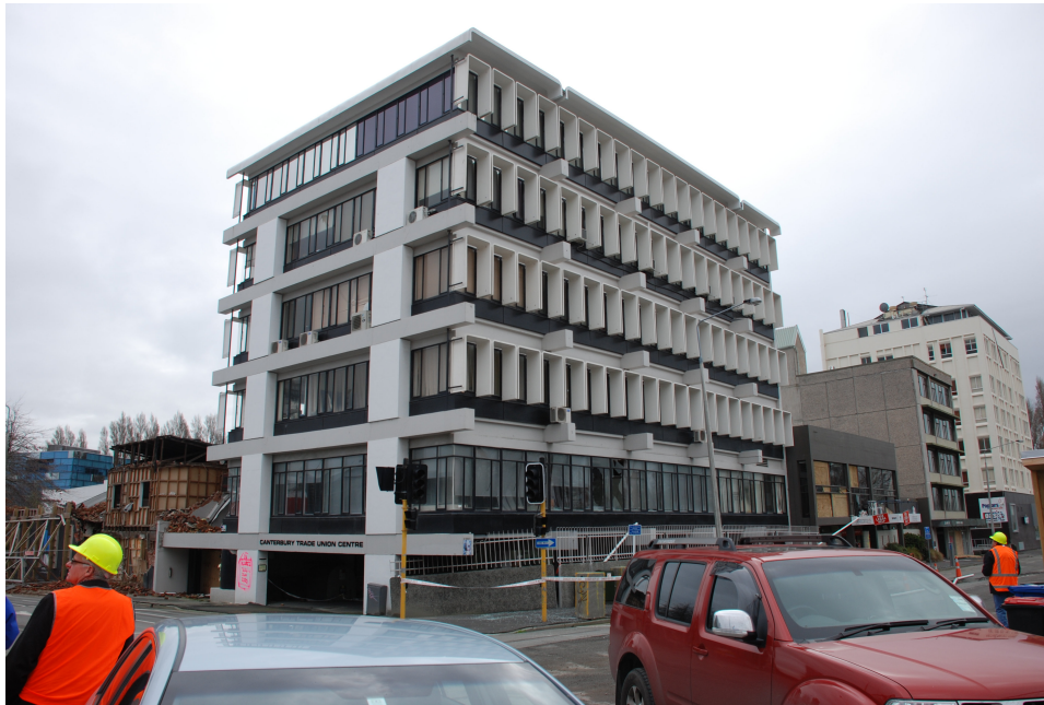
Figure 2-3 The Trade Union building was damaged by both ground shaking and differential settlement caused by liquefaction. This building was later demolished.
