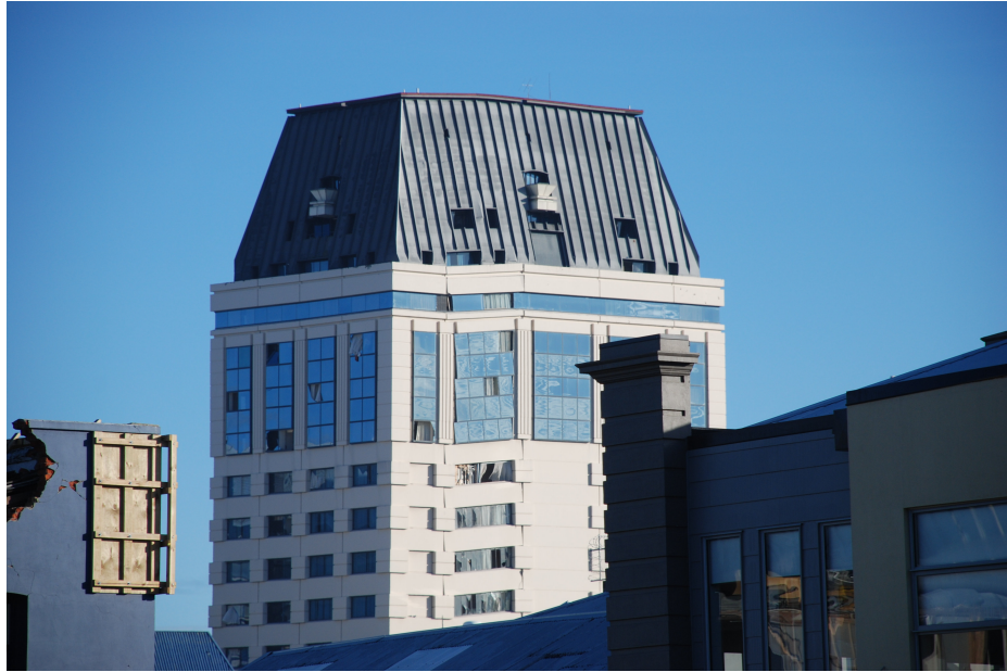
Figure 2-8 The severely damaged Grand Chancellor Hotel in the CBD. This 22-story building was one of a number of high-rise buildings to be demolished.
