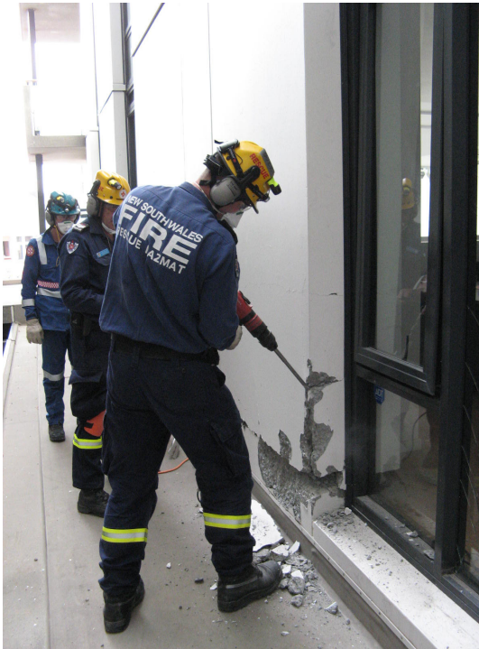
Figure 2-15 Exploration work in concrete shear wall for possible fractured bars. (Source: Des Bull)
