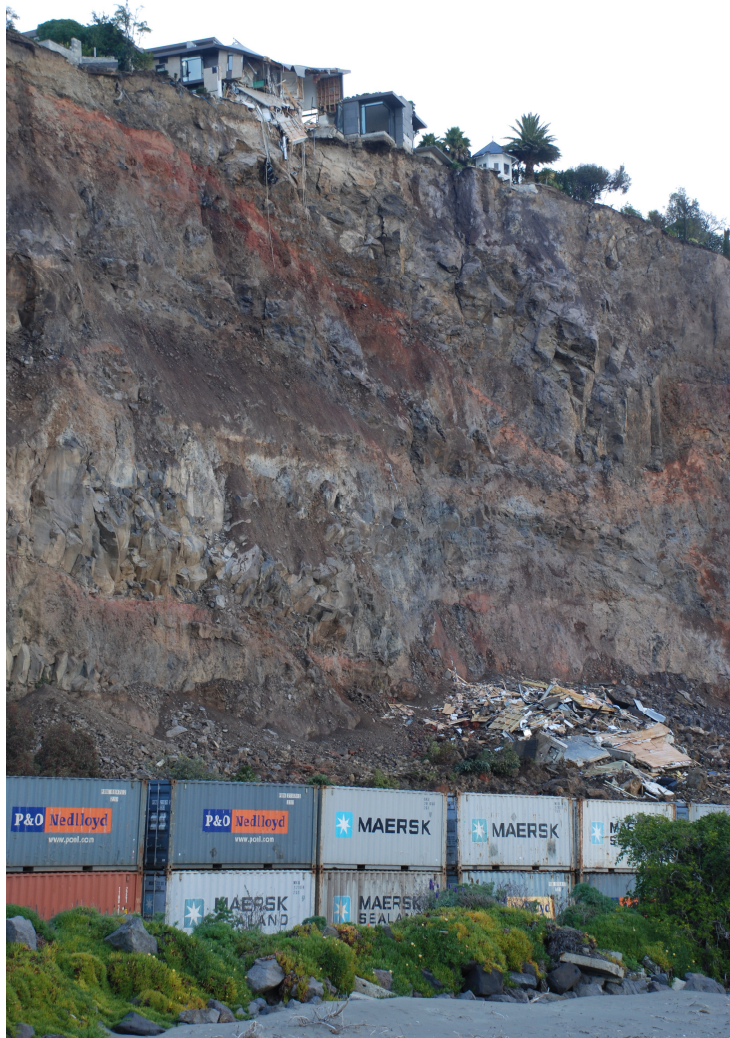
Figure 2-13 A home destroyed by slope failure in the Sumner area. Part of the home is at the top of the cliff and the other part at the bottom (just above the shipping containers on the right).
