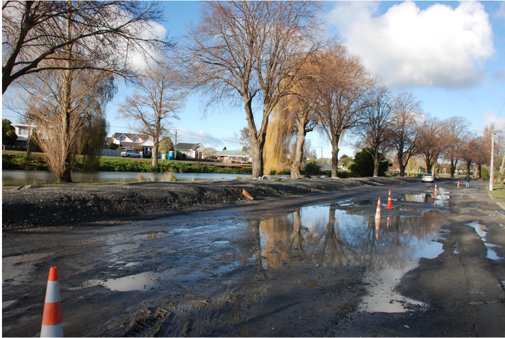
Figure 2-5 New built-up berm on the banks of the Avon River.
