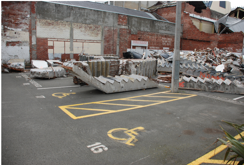
Figure 6-2 Failed precast concrete stairs from the 19-story Forsyth Barr building.
