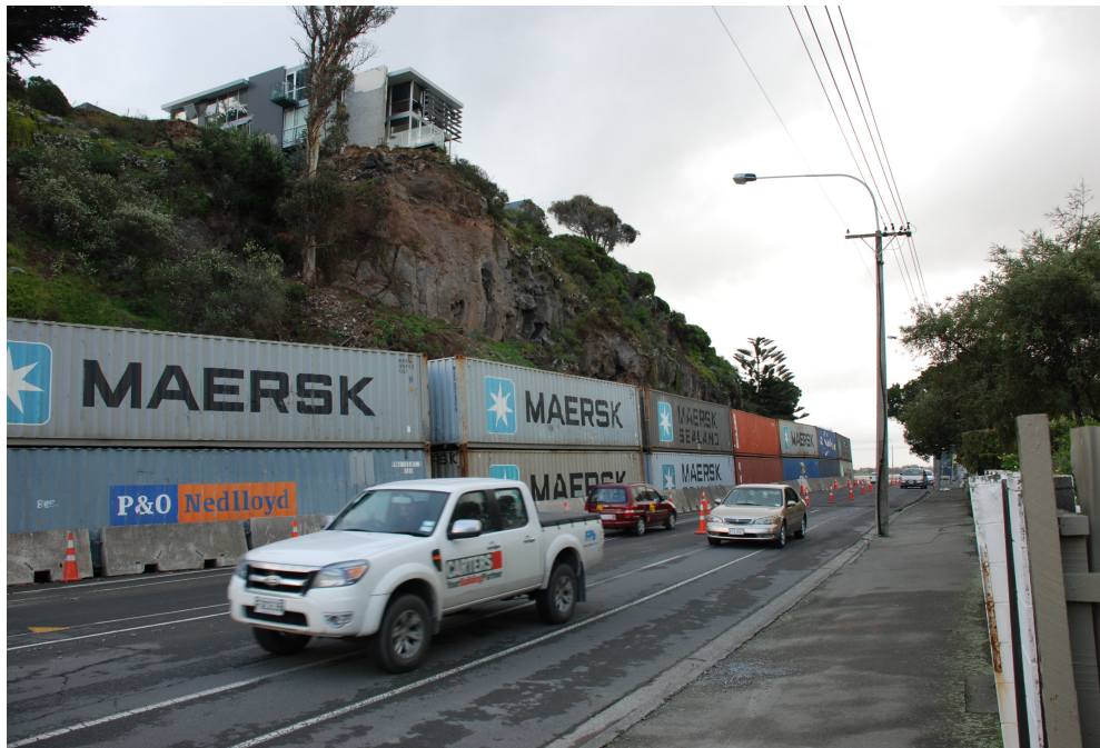
Figure 3-9 Shipping containers were frequently used to barricade roads from slides and rock falls.
