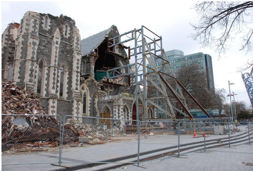
Figure 2-12 Failure of temporary wall shoring at the famous Christchurch Anglican Cathedral intended to allow removal of the Rose Window. The picture at top shows the wall and Rose Window after the February 22, 2011 earthquake, and the picture at the bottom shows the wall, and loss of the Rose Window, after the June 13, 2011 aftershock. (Source: Top picture, Christchurch City Council)
