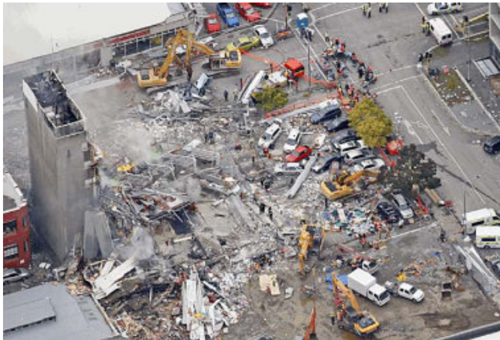
Figure 2-6 CTV building before and after collapse. One hundred and fifteen people were killed in this building. (Source: Hyland and Smith, 2011)
