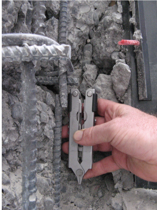
Figure 2-14 An example of a fractured vertical reinforcing bar in a concrete shear wall. (Source: Des Bull)
