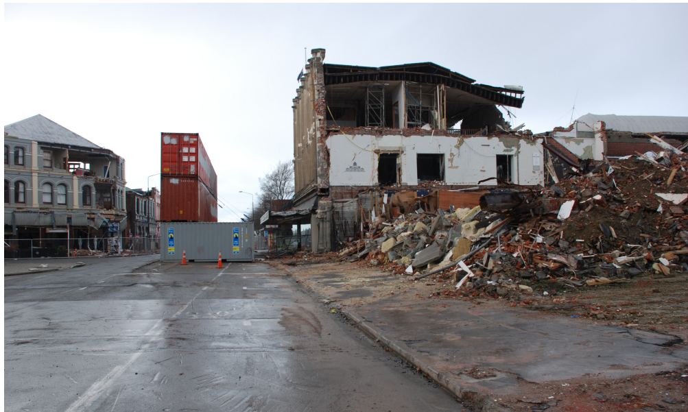
Figure 3-8 Shipping containers were used to keep possible falling debris from damaged buildings from blocking streets. The red containers protect the building to the left and the portion of the street adjacent to it from the URM building on the right.
