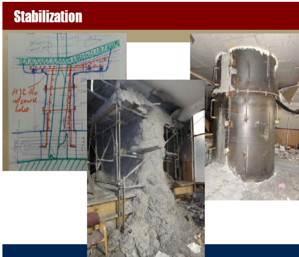
Figure 3-3 Examples of emergency stabilization measures. (Source: Prof. Sri Sritharan, Iowa State University)
