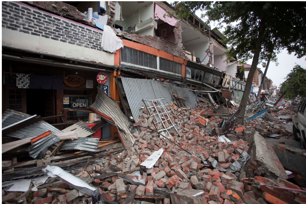
Figure 2-11 Damage in the Christchurch CBD immediately after the February 2011 earthquake. (Source: Christchurch City Council)
