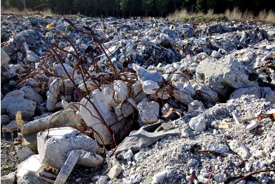
Figure 1 Remains of CTV Building at Burwood
