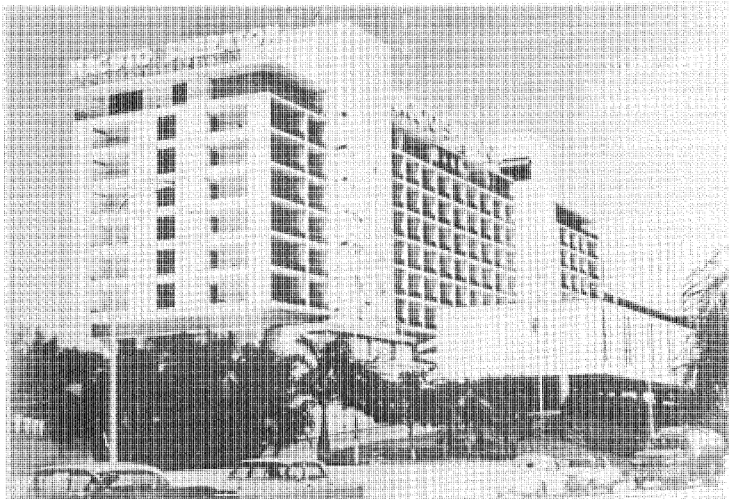
(a) The hotel building after the earthquake
