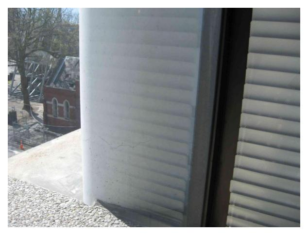
Figure 5 - Photo of Column F4 (249 Madras Street 068C.jpg) at the northeast corner of the CTV Building at Level 4 taken by David Coatsworth during his inspection after the September Earthquake. It is the only column that was found to be cracked below Level 6. See review of Statement of Evidence by damage observer Pagan on page 53. See also the review of the Statement of Evidence by eyewitness Smith on page 55.
