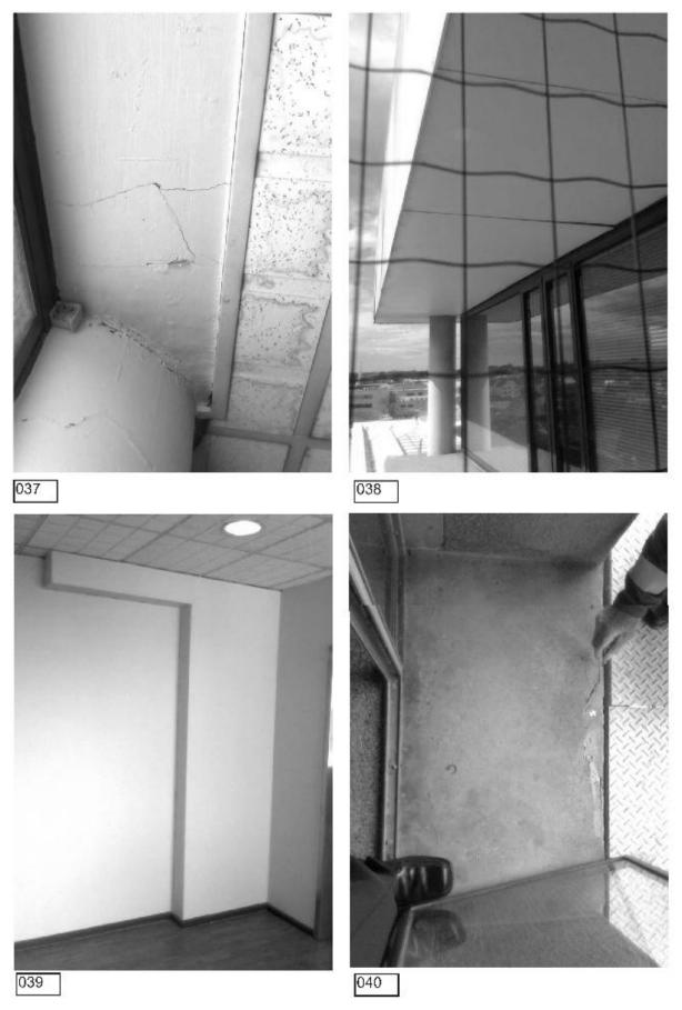
Figure 22 - Collection as photographed by Pagan. Photo 37 shows the damage to the connection of the Column C18 into the North Core overhead wing wall on Line D/E.
