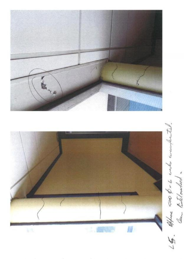
Figure 21 - Photos from Peter Higgins (BUI.MAD249.0454) showing damage to column C18 and connection to overhead North Core wing wall on Line D/E.
