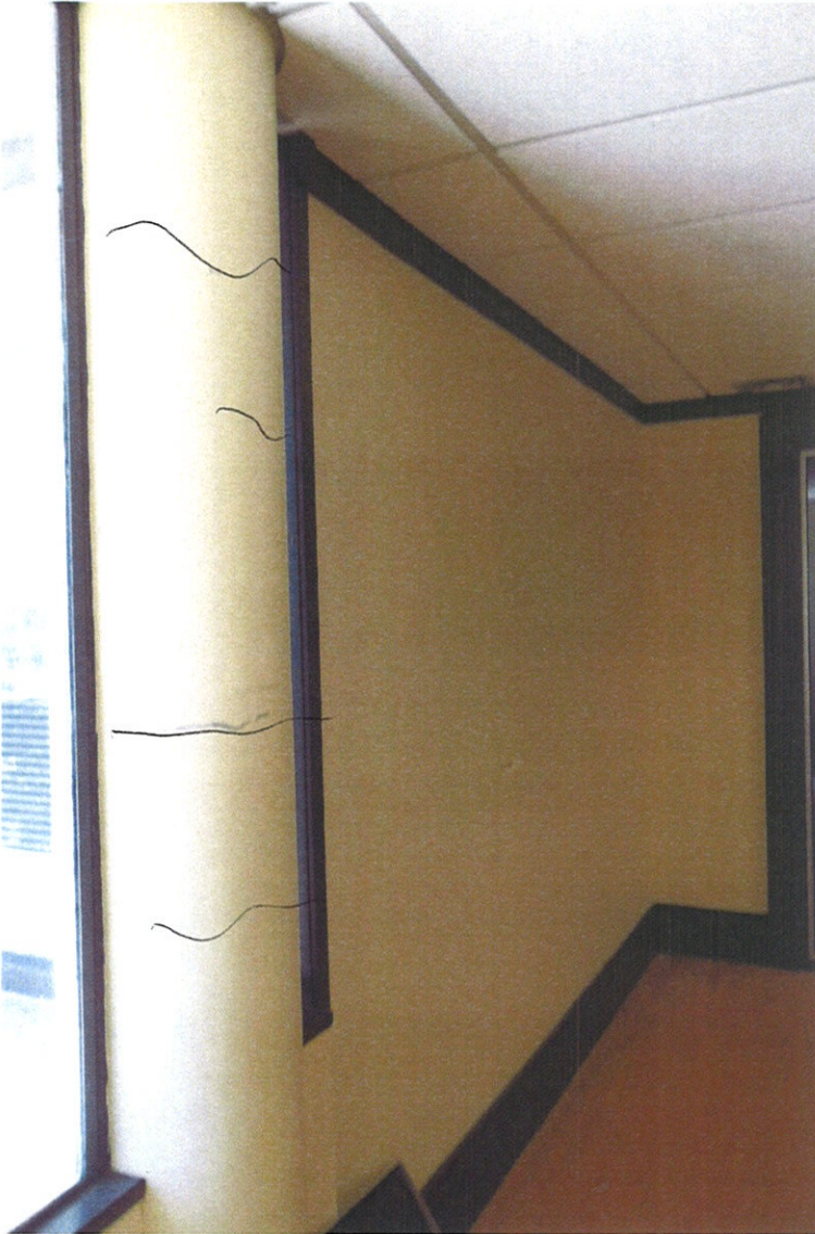
25. Approx 500 \phi \times 6 cracks circumferential. Beam lintel overhead.
