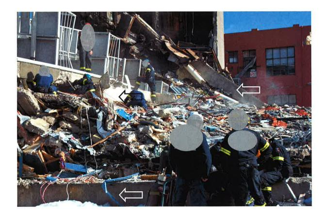
View of South Wall and fire escape stair collapsed onto the Building. The wall "hinged" about a line parallel to its base at about Level 2. The edge beams are no longer attached to the lower levels on the eastern side of the South Wall (4:30 AM 24 Apr 2011).
