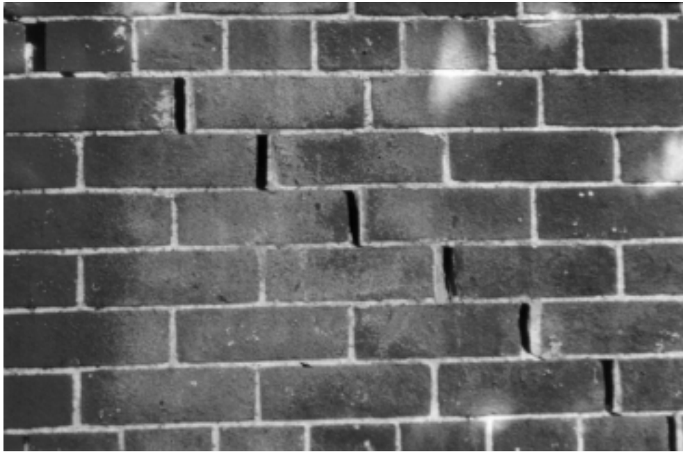
Figure 7-10 Photo of Bed Joint Sliding
