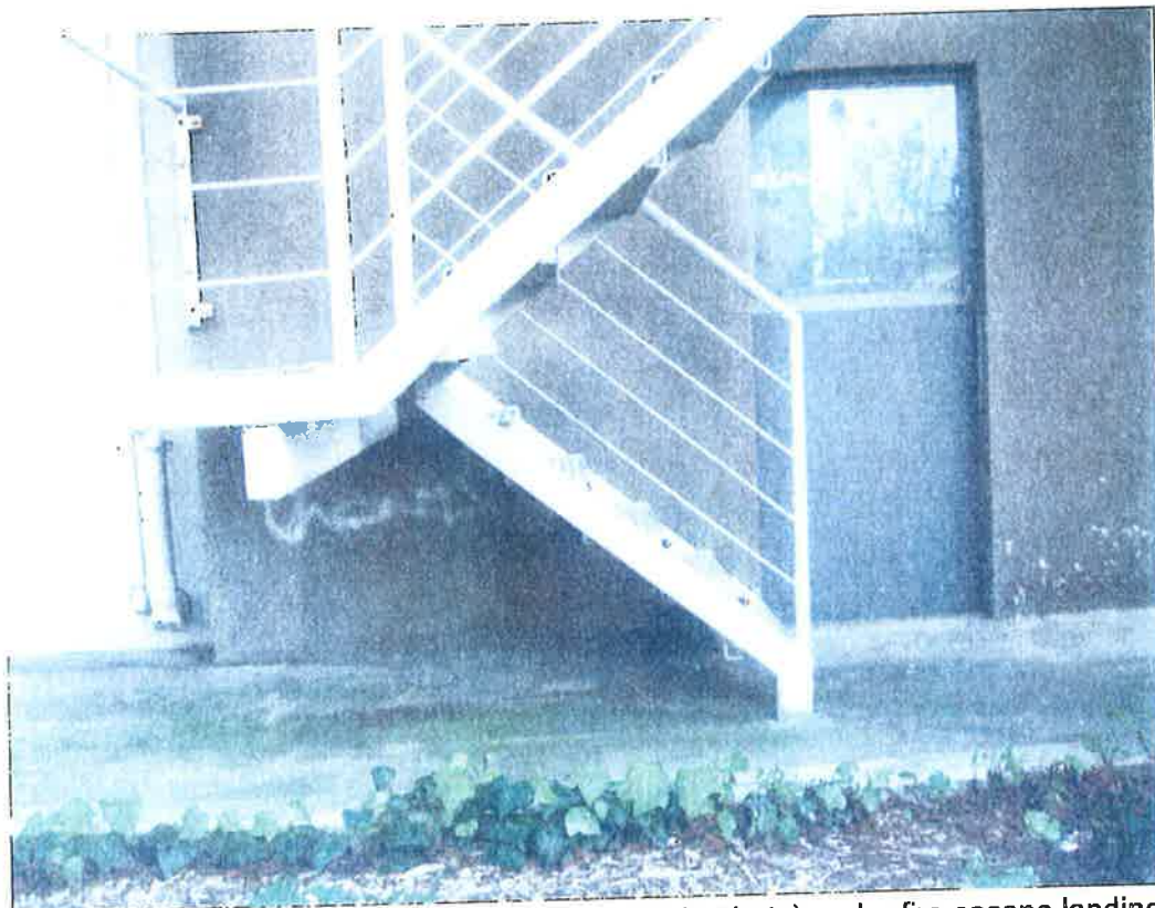
Photo 2 Cracking in south shear wall (not visible in photo) under fire escape landing
