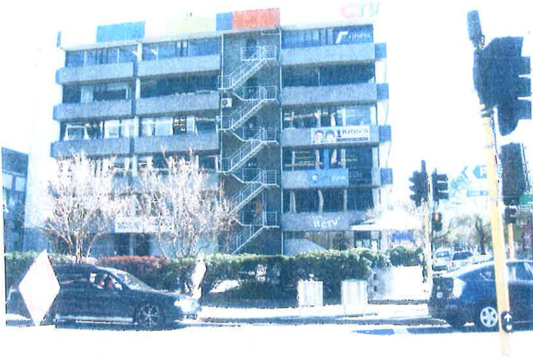
Photo 1 South Elevation of Building
