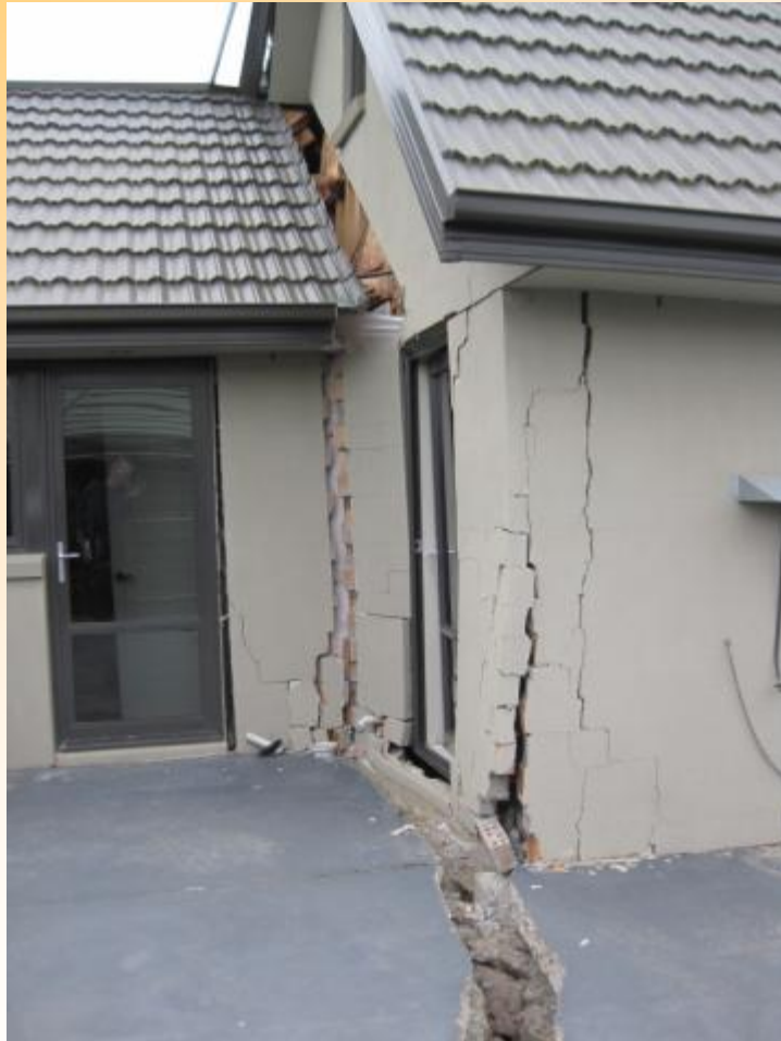
Lateral spreading
