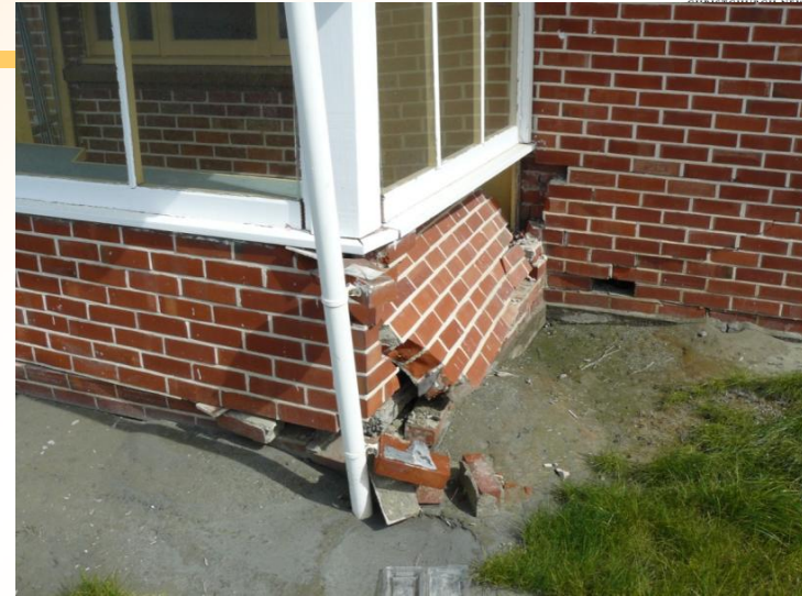
Differential sinking
