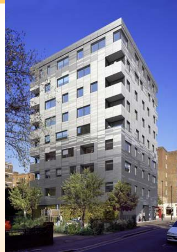
9 storeys – London (CLT panels)
