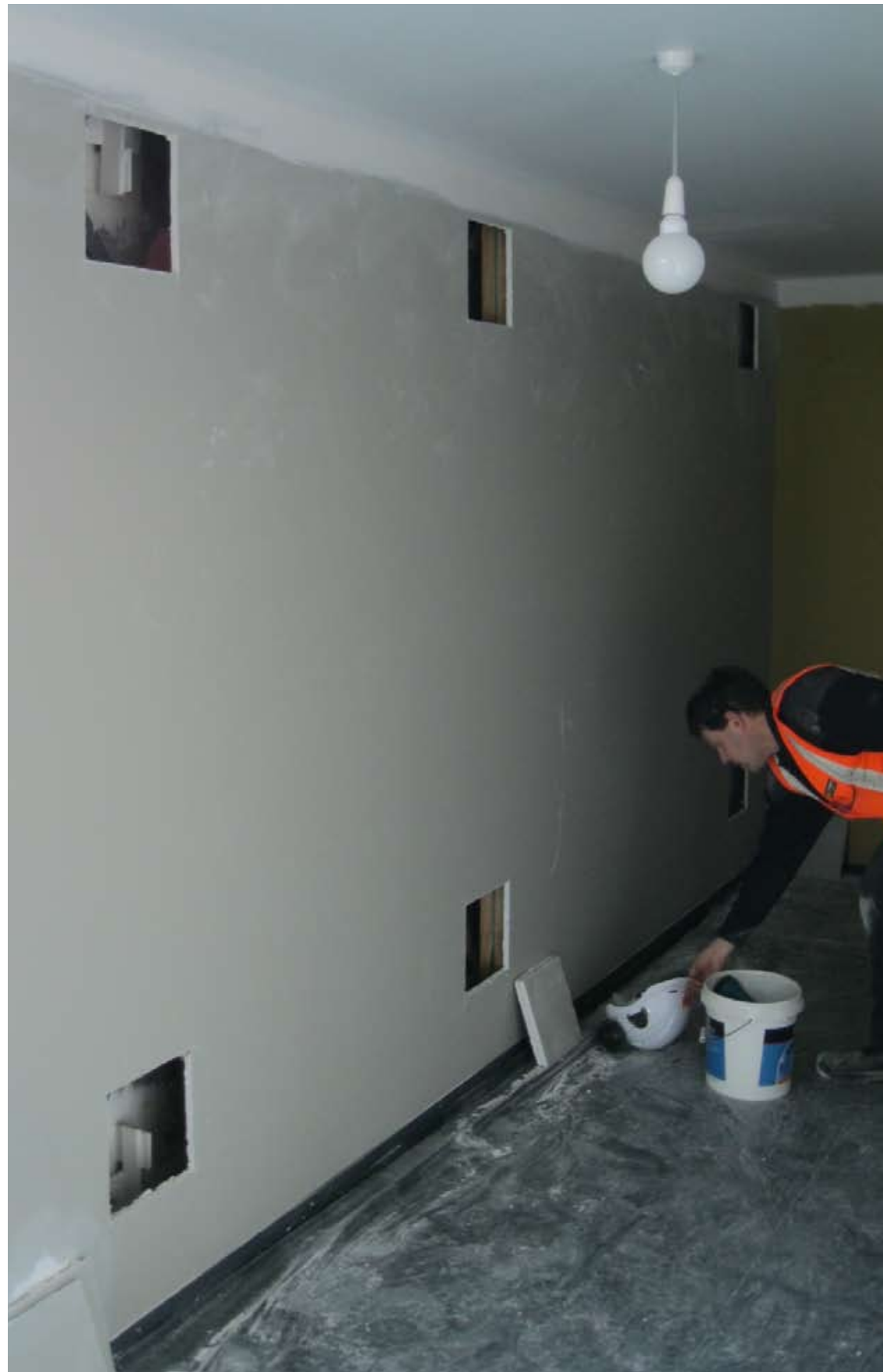
ease of inspections of structural connections
