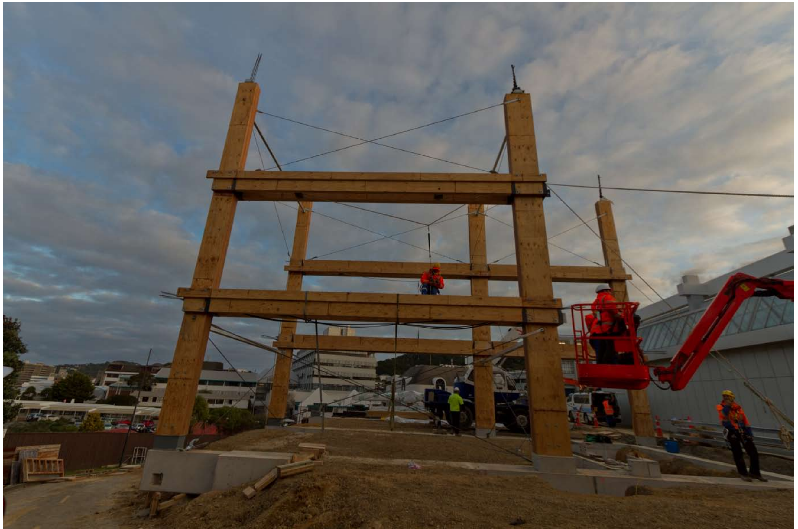
LVL timber post tensioned frame - a world first for multi-storey construction
