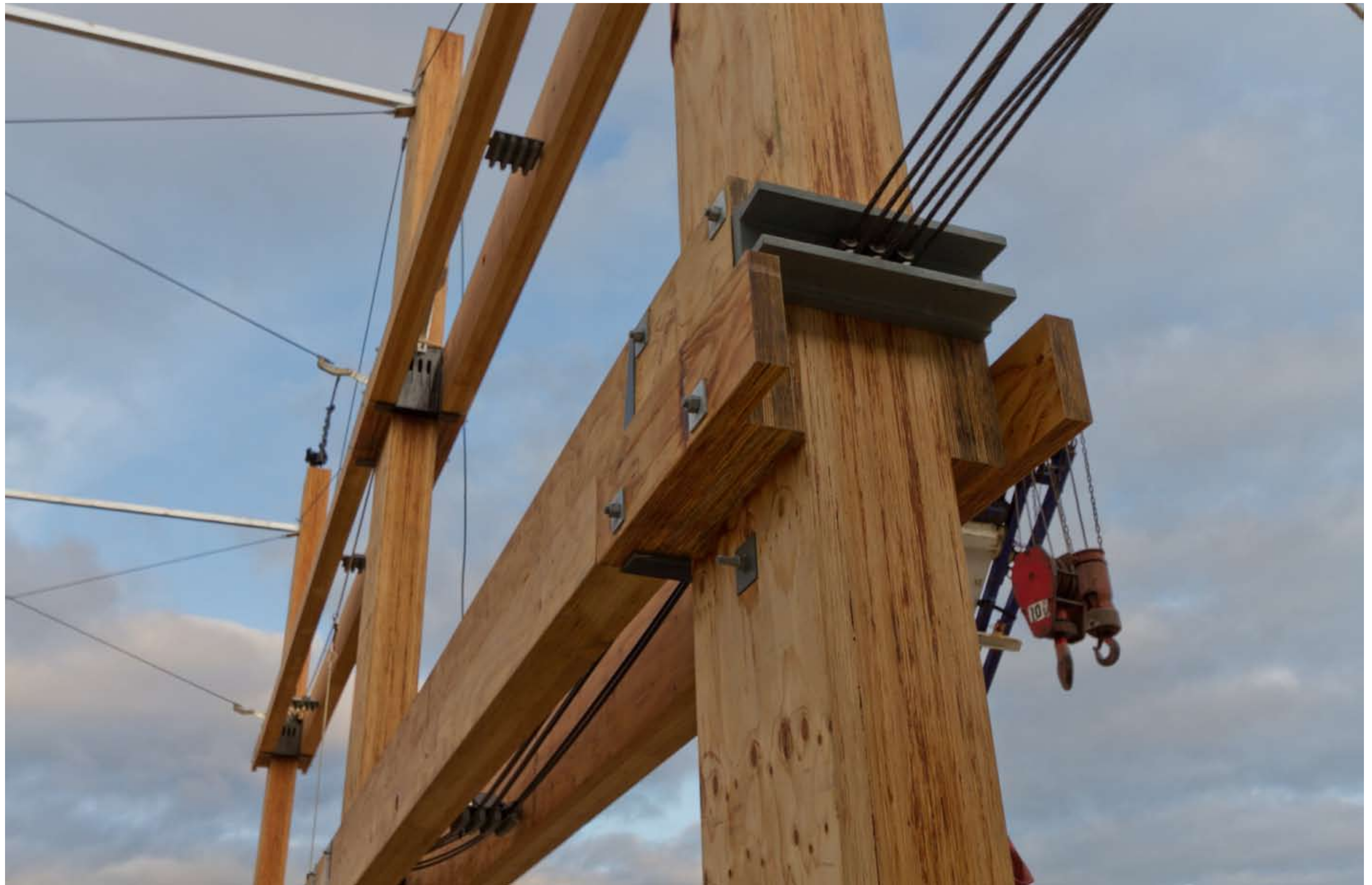
LVL timber post tensioned frame - a world first for multi-storey construction
