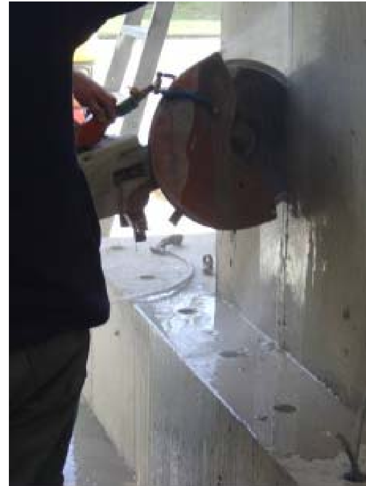
Vertical saw-cutting
