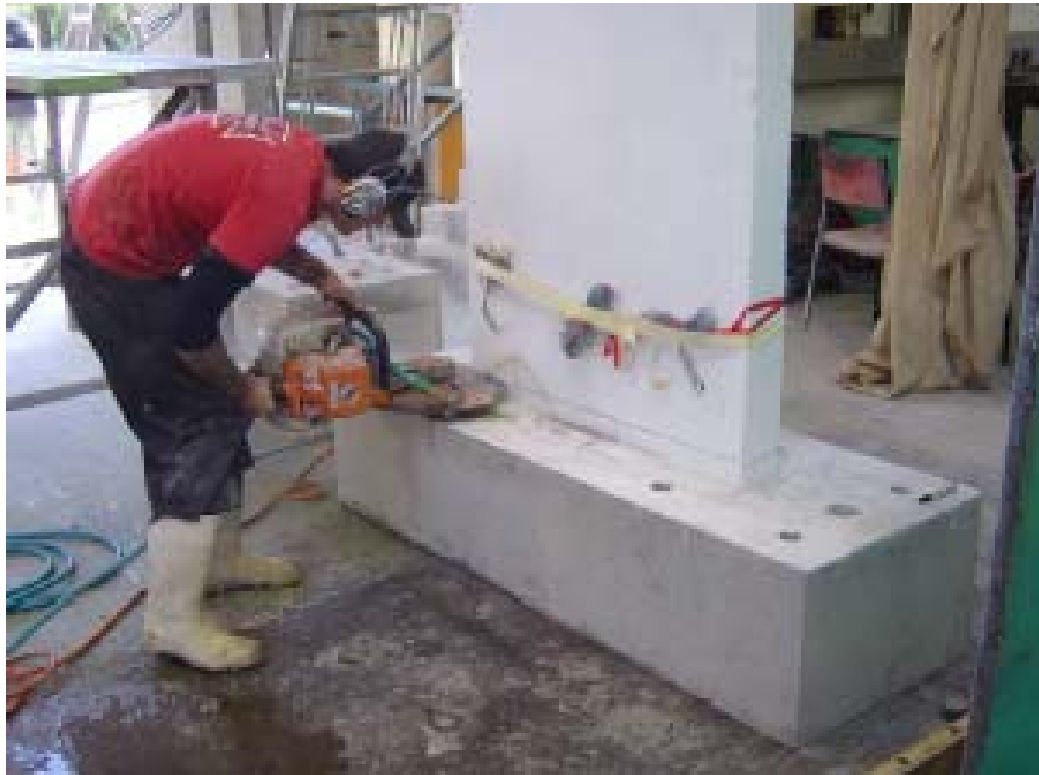
Horizontal saw cutting at the wall base (Acknowledgments to Contech)
