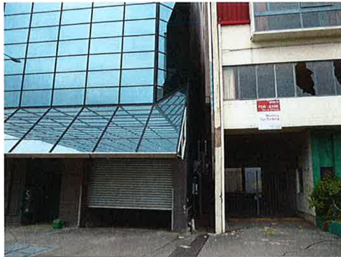
Separation to building to the south
