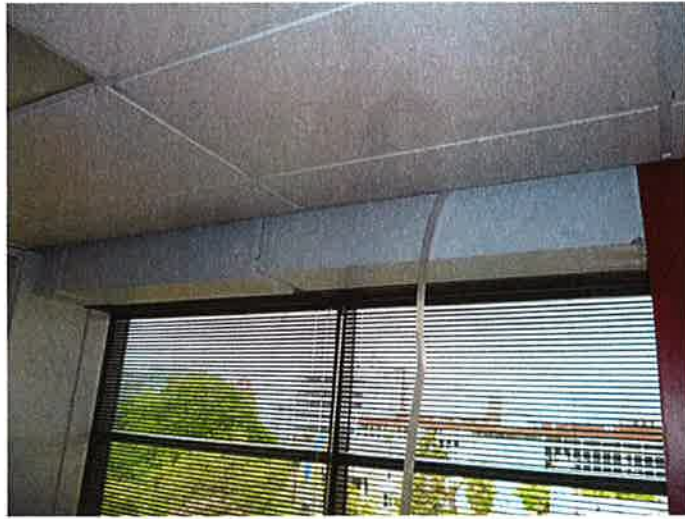
General view of splice to beam
