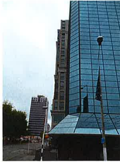
View of building tilting to south
