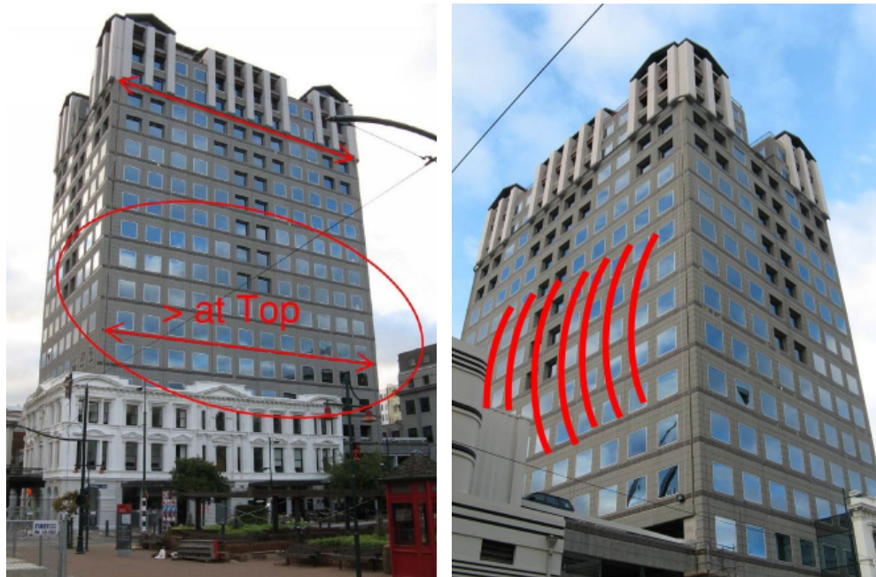
Figure 9: Frame Elongation (left) and Bulging at levels 5 to 11 (right) [31]
