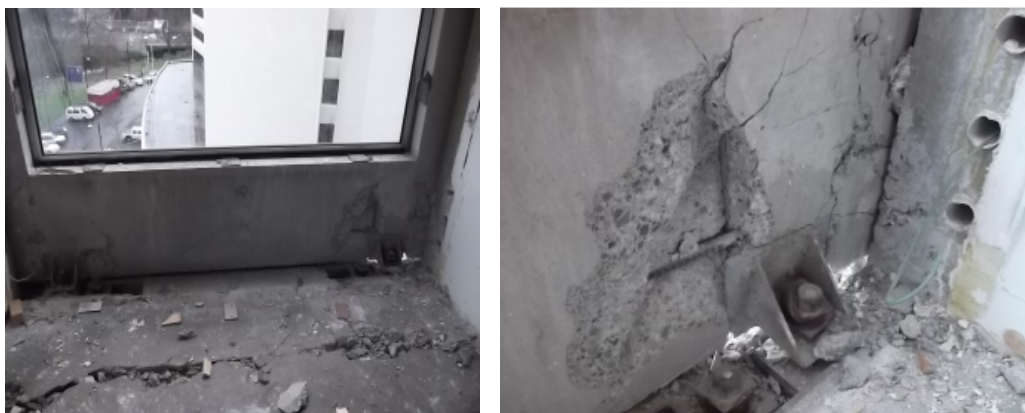
Figure 15: Precast Panel Connection Damage [31]
