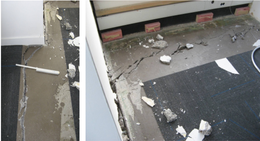
Figure 10: Diaphragm Cracking [31]
