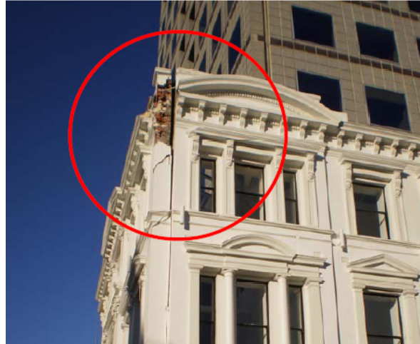
Figure 16: Historic Facade Damage [31]
