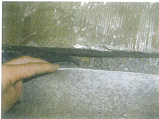
Photo 3. Debris in Seismic separation
