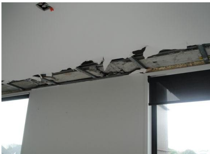
Severe spalling of insitu concrete edge beam along 'un-bonded' section adjacent to panels
