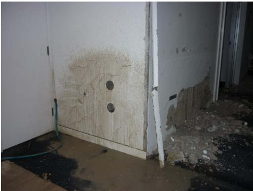
Figure 7 Core location on Wall element
