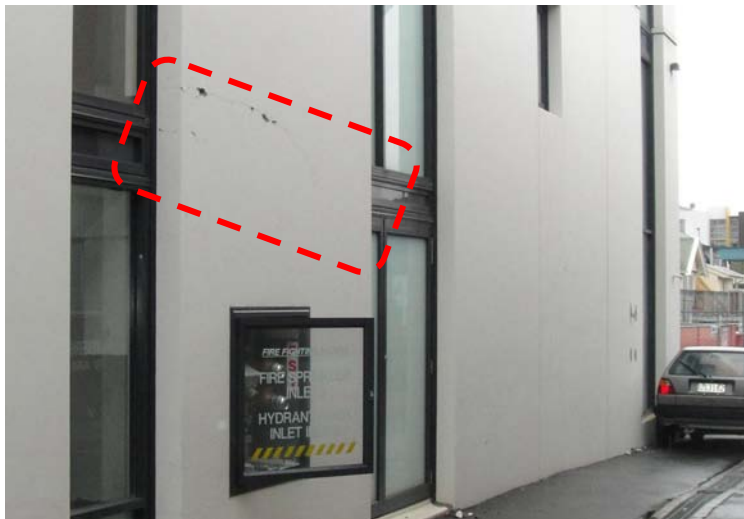
Cracking to grid F external panel on east side.
