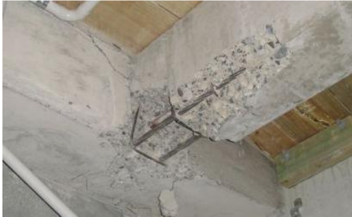
Exposed pre-stressing strands from inter-span rib into damaged insitu concrete edge beam
