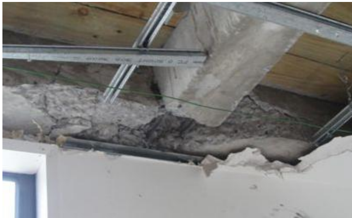
Severe spalling of insitu concrete edge beam along 'un-bonded' section adjacent to panels
