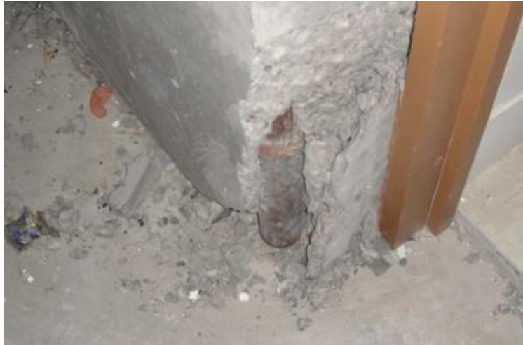
Spalling of concrete around vertical reinforcement couplers at end region of panel.
