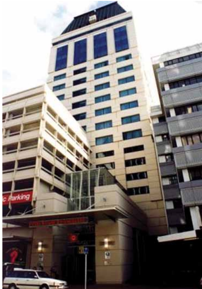
Figure 7.1: Hotel Grand Chancellor Building pre-September 2010 earthquake (source: C Lund & Son Ltd website)
