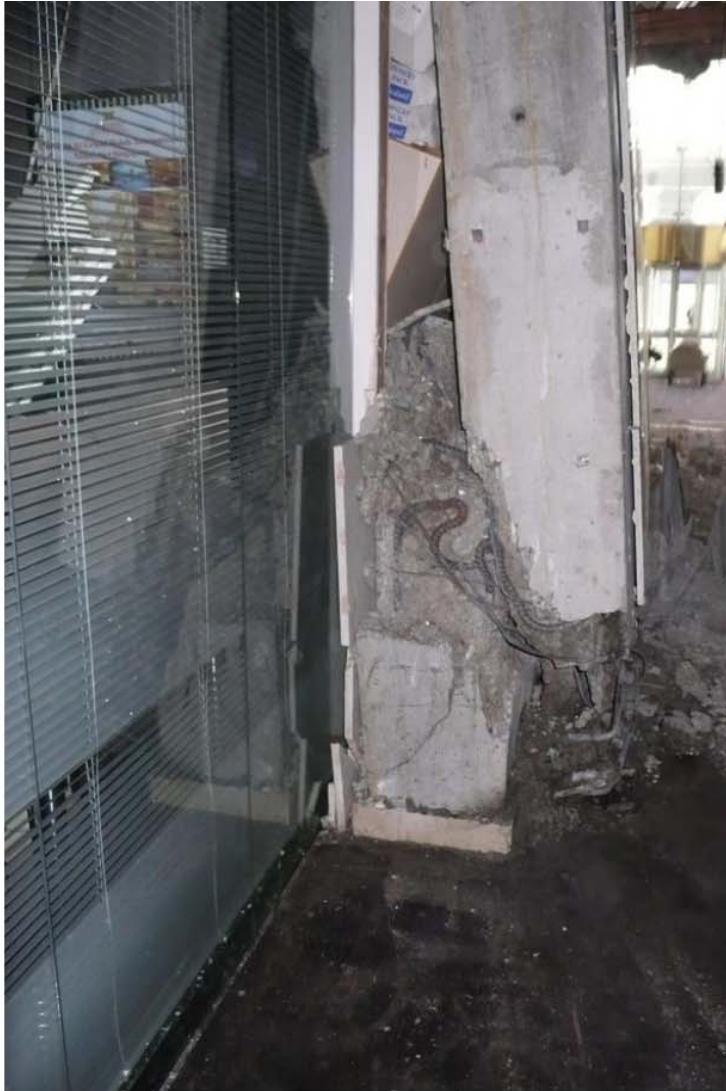
Photo 9 - Shearwall D5-6 Failure - End View
