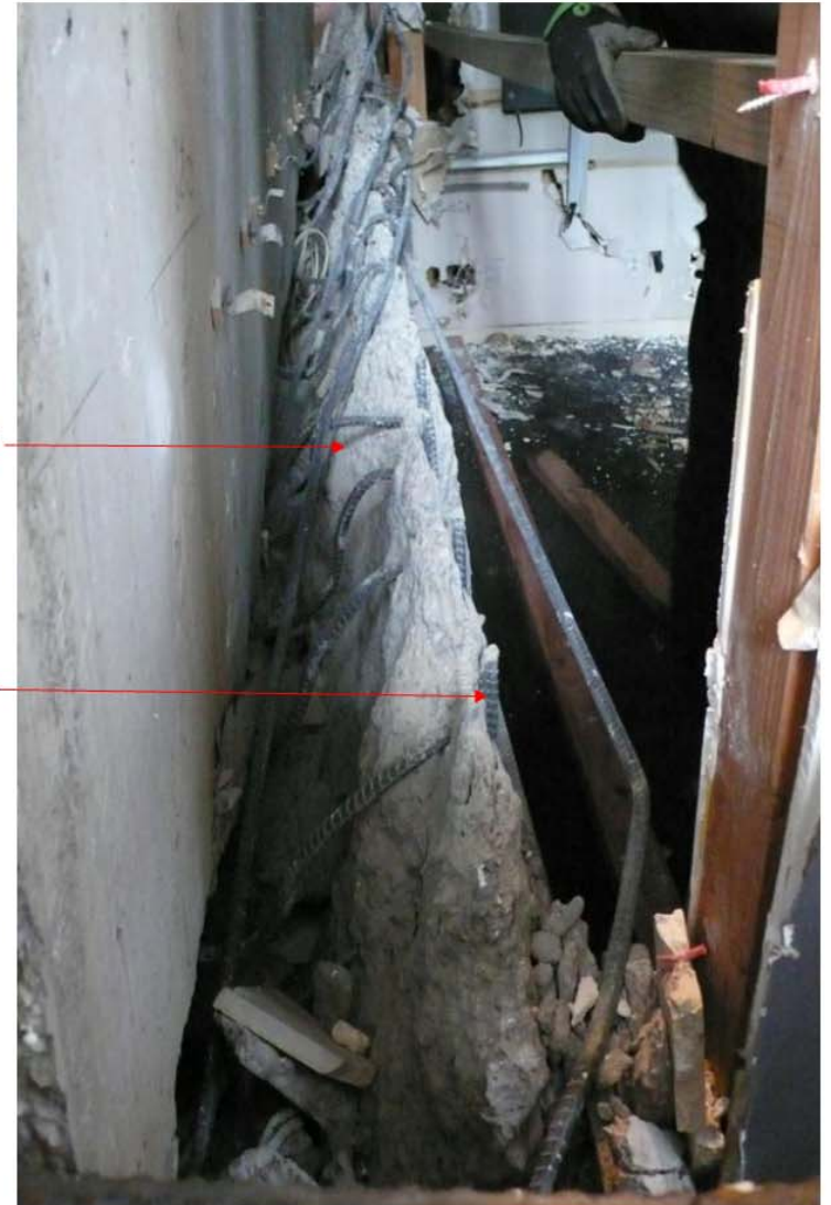
Photo 10 - Shearwall D5-6 Failure - Close-up
