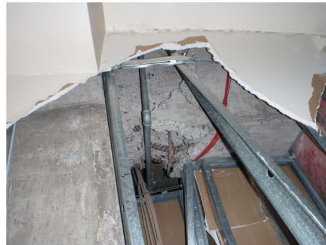
Photo 18 - Hinging in grid D tower beams
