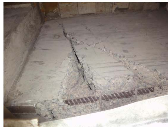
Photo 19 - Hinging in grid D tower beams
