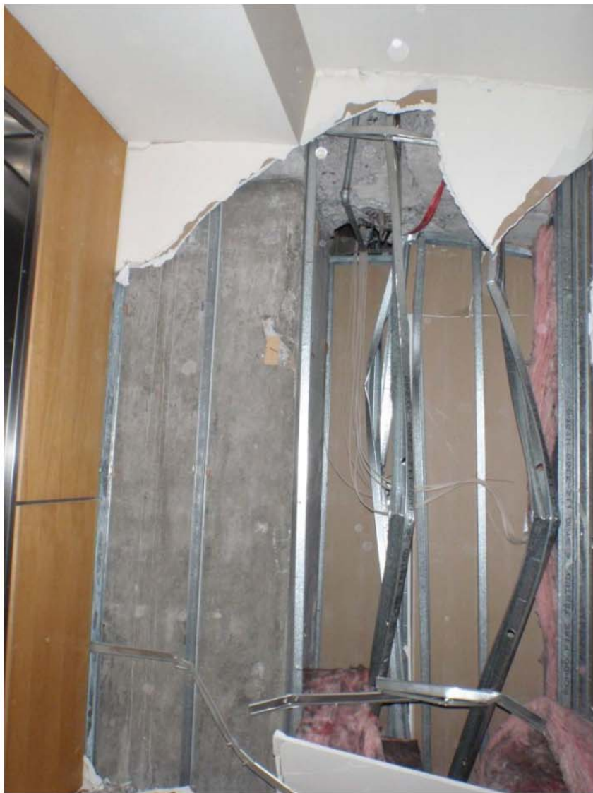
Photo 17 - Hinging in grid D tower beams
