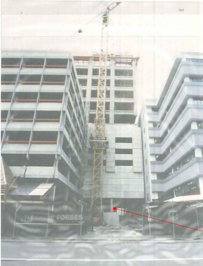
Photo 1 - Southern Elevation - During Construction
