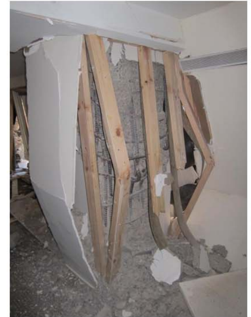
Photo 21 - Crushed columns at level 10, lines 5 & 6
