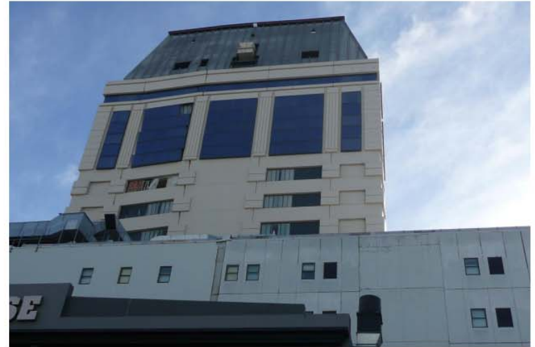
Photo 4 - Eastern Elevation - Post February
