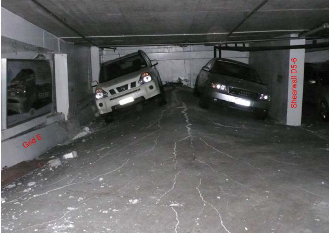
Photo 13 - Folded slab at level 2
