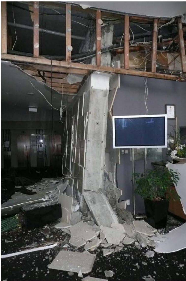
Photo 6 - Shearwall D5-6 - Base Failure
