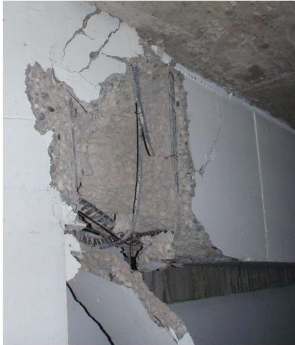
Photo 14 - Hingeing in grid E beams 6-7
