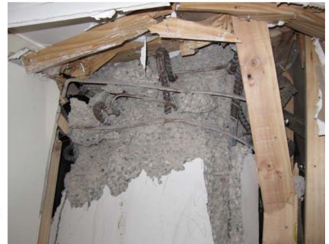
Photo 22 - Crushed columns at level 10, lines 5 & 6
