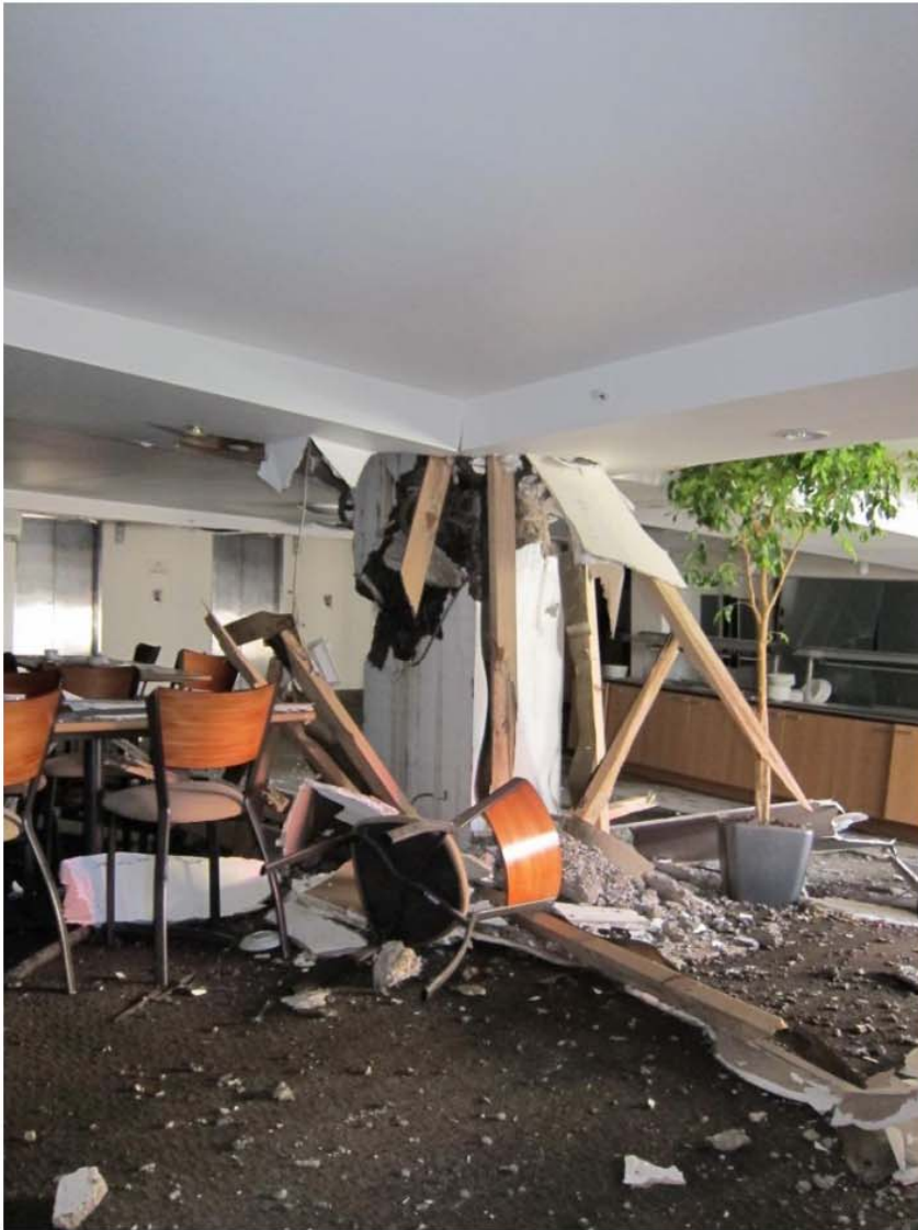
Photo 20 - Crushed columns at level 10, lines 5 & 6
