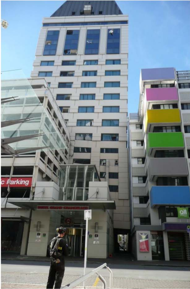
Photo 3 - Southern Elevation - Post February
