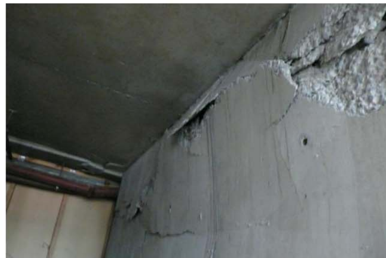
Photo 8 - Shearwall D5-6 - Hingeing at top of ground floor
