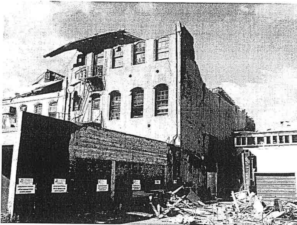
Photo 2: Northwest corner of building showing only remaining 3rd floor walls and roof.
