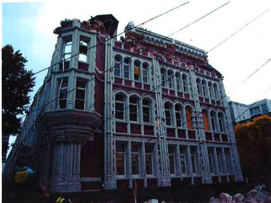
Figure 2: South facade. Note parapet since removed
