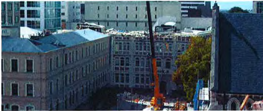
Figure 1: View of roof/fourth floor from above
