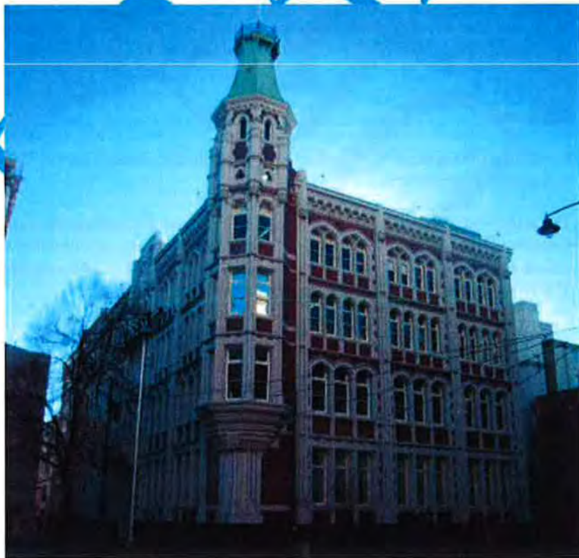
Figure 1-1 View of Building from Worcester St
