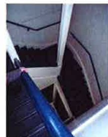
Original Northern Stair
