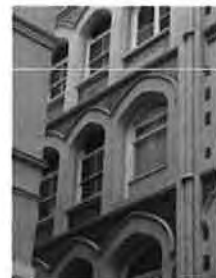
Service Bay Second Floor Windows
