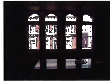
Articulated windows to South Elevation
