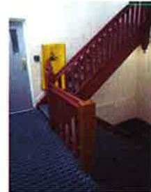
Third Floor Stair Landing. Change to more modern Southern Stair
