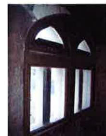
Original Pigeon House windows
