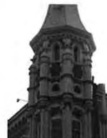
Roof Top Windows
