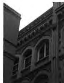
Service Bay Third Floor Windows with remnant section of parapet
