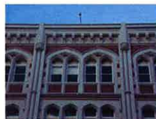
Third Floor Windows
