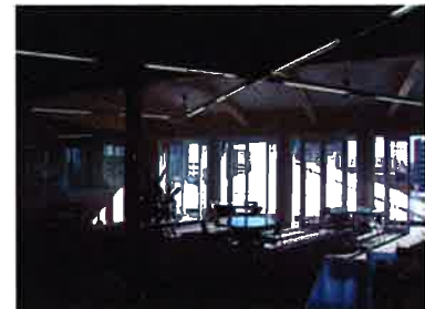
Original Ceiling and Column in Cafeteria
