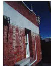
North Elevation showing brick and concrete cladding
