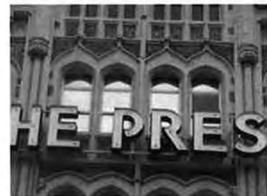
Entry Bay Third Floor Windows
