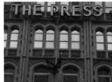
Entry Bay Second Floor Windows
