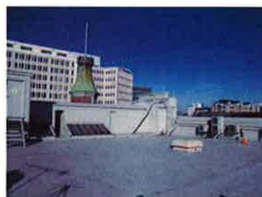
Southern Stair & Pigeon House
