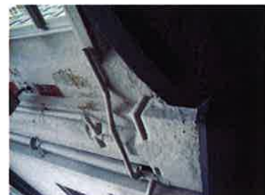
Painted modern penetrations
