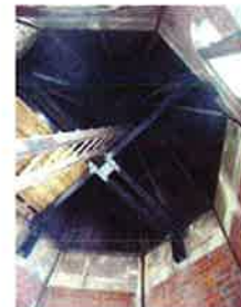
Inside Roof Tower showing steel and timber structure
