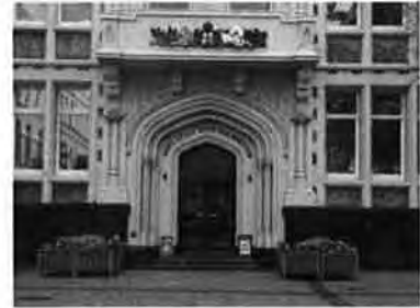
Entry Doors and Projecting Hood
