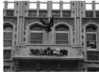
Entry Bay First Floor Window
