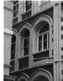
Service Bay First Floor Windows
