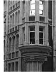
First and Second Floor Windows
