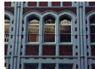
First Floor windows
