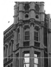
Second and Third Floor Windows
