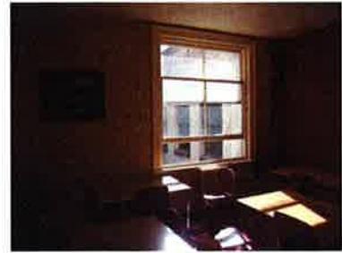
Large glazed timber windows to Eastern Light well
