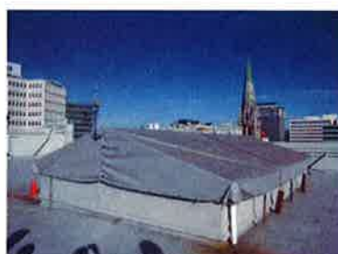
Skylight to Cafeteria
