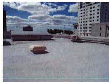
Roof looking North
