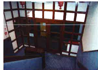
Southern Stair Lobby Fire Separation
