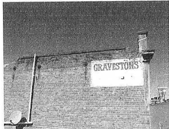
Figure 2: Damage to brickwork.
