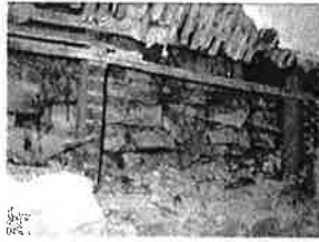
wall construction viewed from inside
