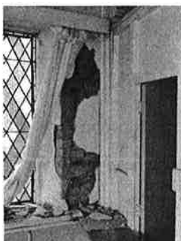
Annex north wall spalling plaster around window
