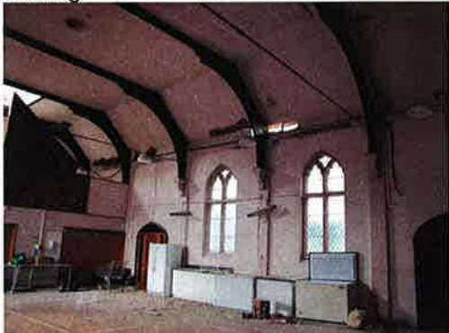
East wall of hall
