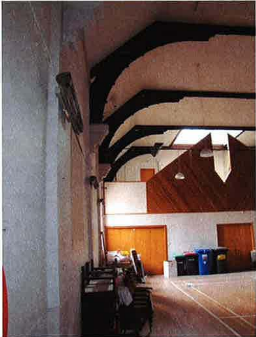
West wall of hall
