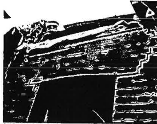
Dislodged bricks to north end of fire escape
