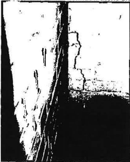
Vertical crack to upper level SE corner of building
