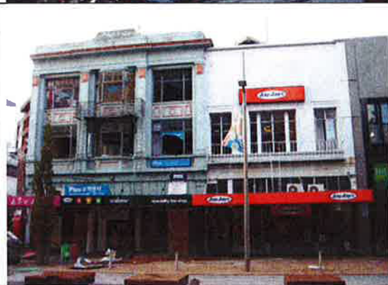
3 – Adjacent building to south east appears to have utilised the side wall of 242 High Street as a party wall
