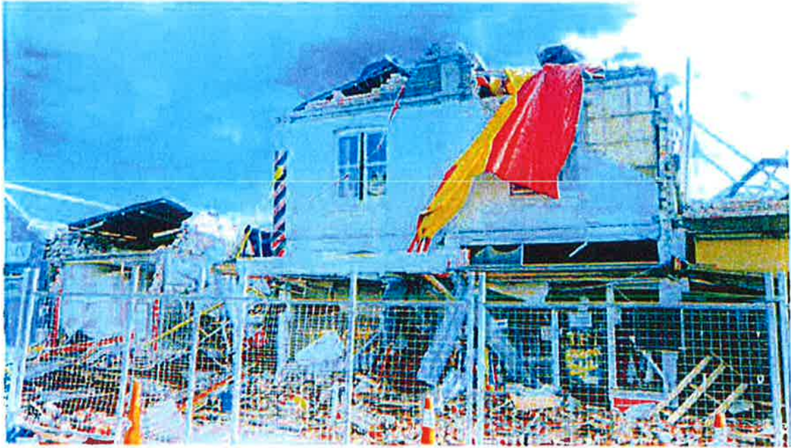
Photo 3 : After the Feb 22, 2011 quake.
