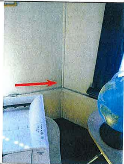
Photo 15. Plaster cracking
