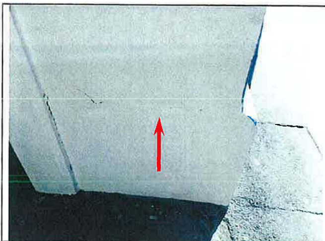
Photo 5. Plaster cracking
