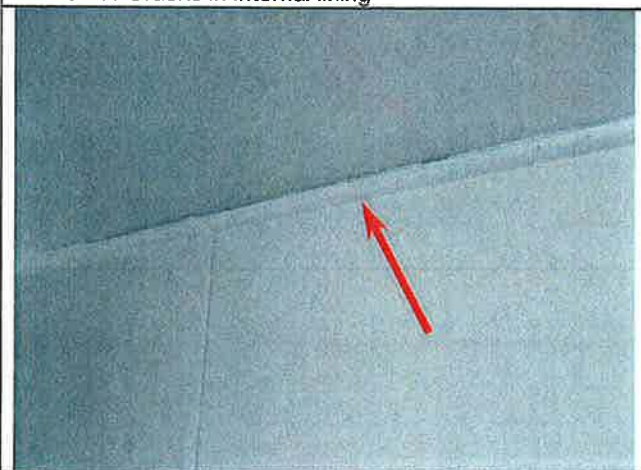
Photo 19. Plaster cracking
