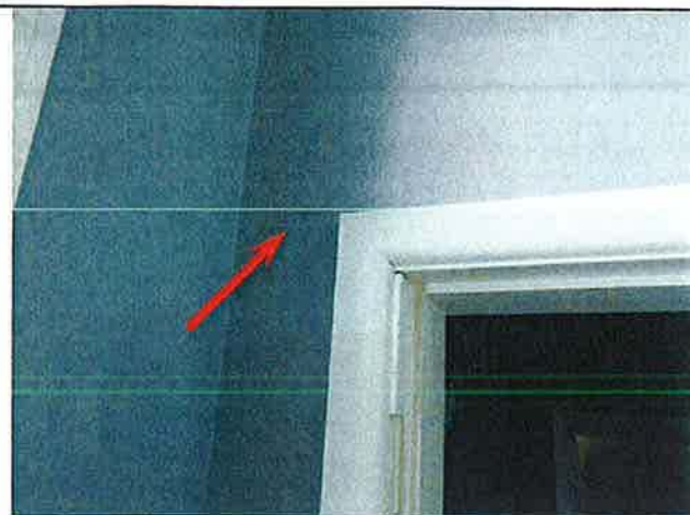
Photo 6. Plaster cracking
