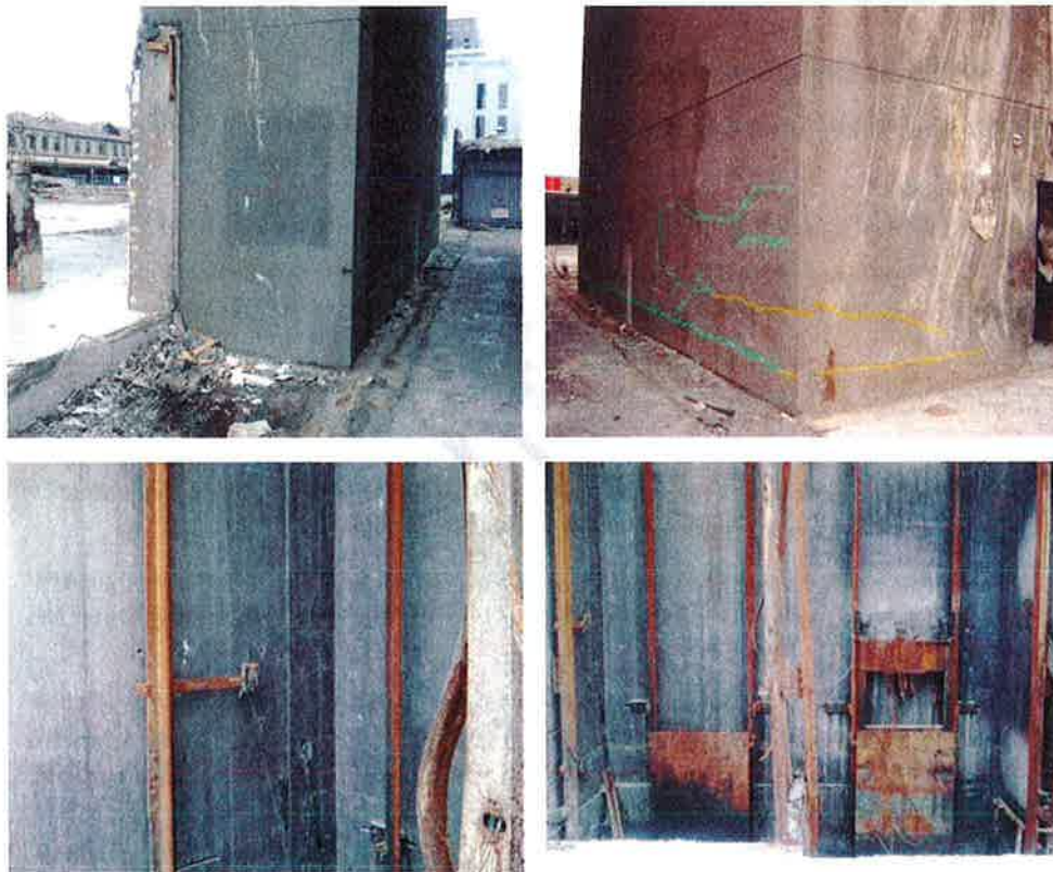
Figure 34 - North Core cracking (clockwise from top left) (a) No obvious cracking on Line D/E wall; (b) Horizontal flexural cracking on west and north west face of Line 5 wall and north end of Line C wall at Line C/5; (c) Fine two-way diagonal cracking on the inside faces of Level 1 to 2 Line 5; (d) and D walls in North Core.
