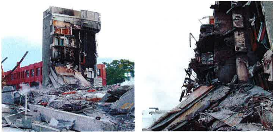
Figure 84 – View of North Core showing Level 4 slab lying diagonally on top of Level 3 slab. This indicates that the Level 3 and 4 slabs lost their vertical support on Line 3 prior to breaking away from the North Core.
