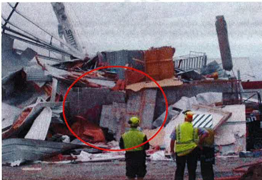
Figure 121 - West wall shortly after collapse. The corner Grid 1/A column is still standing and the wall panels have broken free in panel sections in places. The edges of the panel section are square consistent with the design drawings. Diagonal fracture of the masonry infill that has fallen outwards from level 2 is highlighted. This indicates that the infill masonry above Level 2 fully developed its shear capacity prior to the collapse and therefore affected the response of the structure to the Aftershock.
