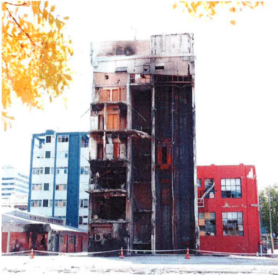
Figure 93 - All debris removed leaving the Level I slab on grade and remnants of the North Core.
