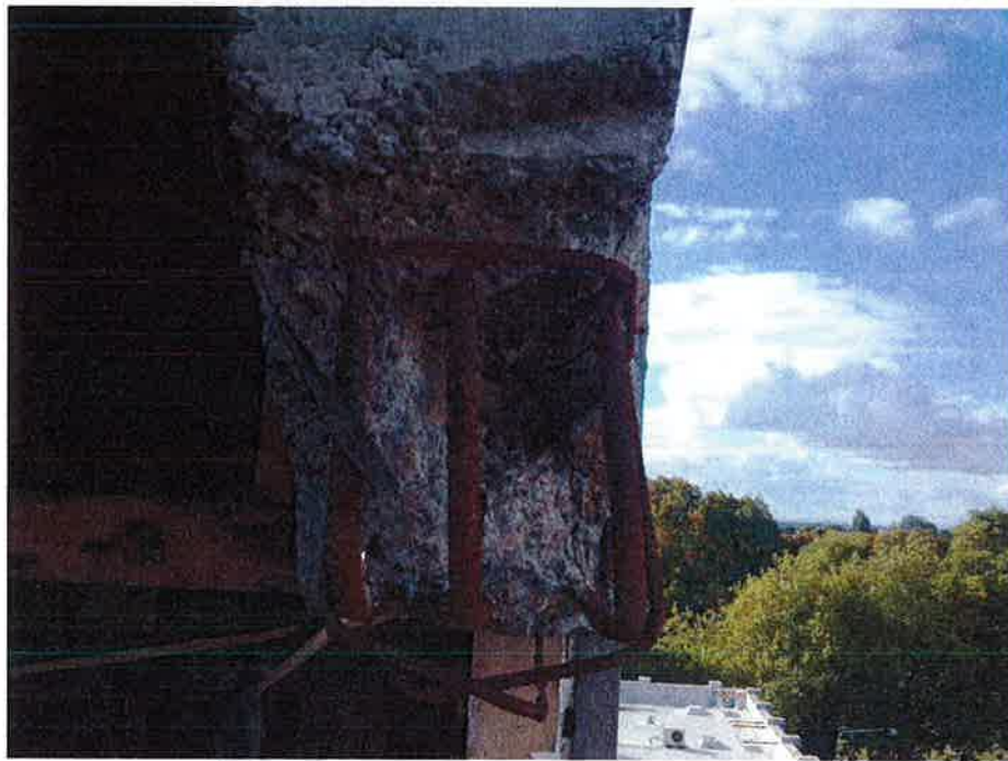
Figure 105 - Lift Well Wing Wall D/E: Column D/E 4 Connection (DENG Dwg S14); 3 x 20 to 24 mm diameter holes can be seen where reinforcing bars from column have pulled out. The drawing shows that 4-H20 bars were required to be bent in to the wall.
