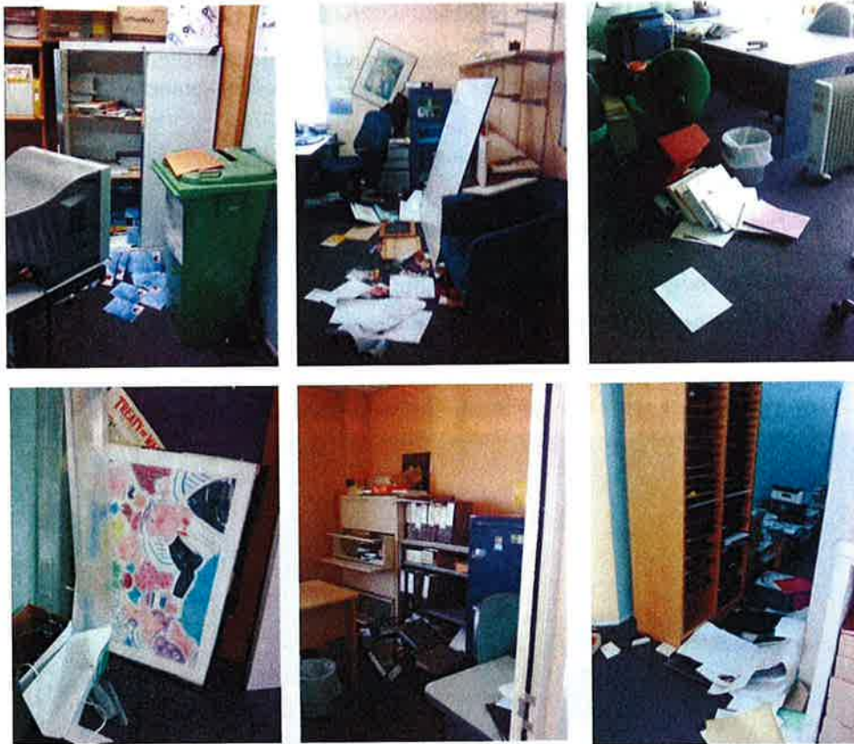
Figure 20 - Damage after 26 December, 2010 aftershock on Level 6 of CTV Building (clockwise from top left) a) Cabinet door had opened but hadn't fallen over though not attached to the wall (Line 3/B-C); b) As it was except that the filing cabinet had been stood back up (Line 2/A-B); c) Oil heater had been righted. Two filing cabinets had fallen to the floor; (Line 1/B-C) d) The cubby-hole unit had not emptied of papers in the earthquake on 4 th September. However in December it had fallen against the corridor wall towards Cashel Street. It had been righted before the photo was taken. (Line 2/B-C) e) The shelves and filing cabinets had gone down, but had been righted before the photo was taken (Line 4/A-B). f) The painting had fallen from the wall. (Line 1/A-B).
