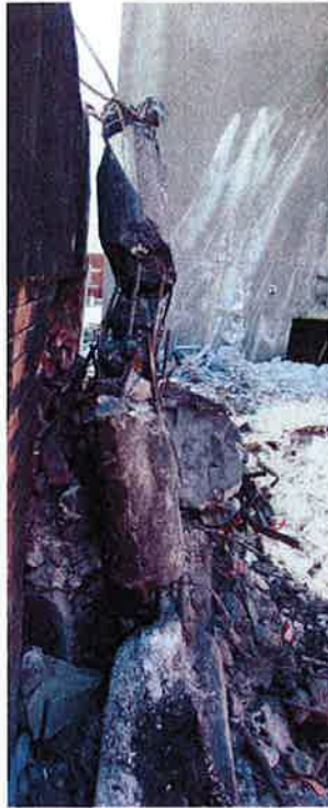
Figure 32 - Line 4 / B column with precast log beam in foreground and shell beam at rear. The column appears to have broken its back on a precast concrete Spandrel Panel and sustained head damage during the collapse.
