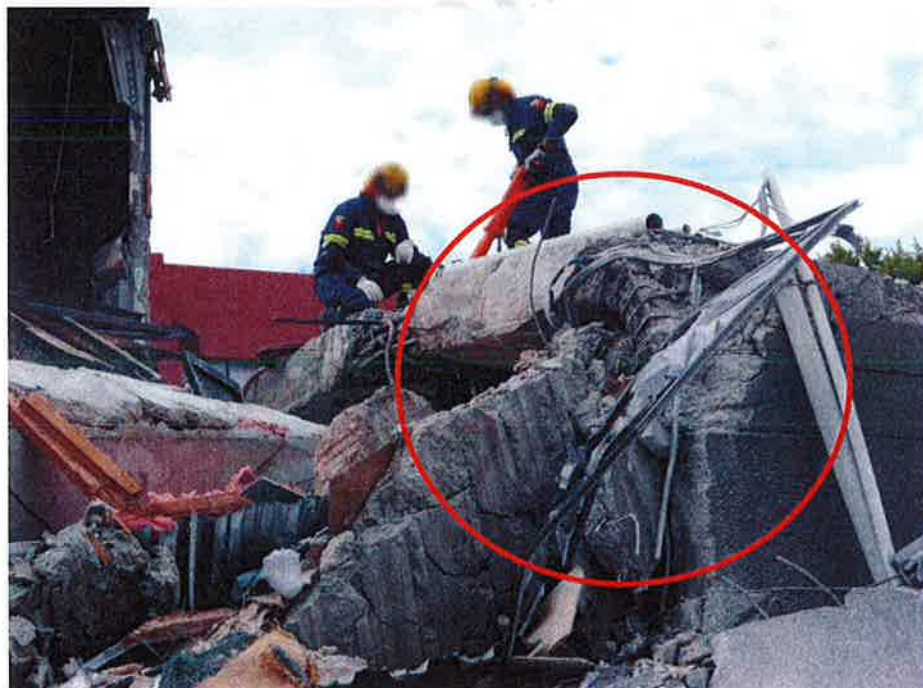
Figure 81 – Upper portion of South Wall being prepared for removal. A portion of slab can be seen highlighted in the foreground in contact with the South Wall on this side at Level 2. It may have forced the wall to pivot against it, preventing it breaking over at its base at Level 1.
