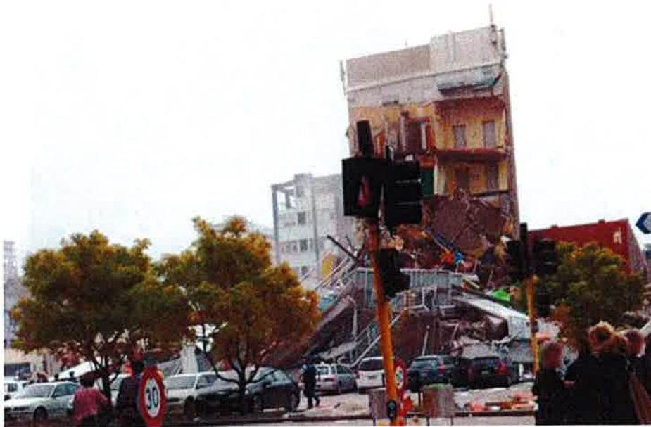
Figure 23 - Cashel St. south face with North Core tower in background immediately after collapse and prior to the fire starting. The cars in the car park on the south face were largely undamaged. The white escape stair that was attached to the South Wall can be seen still attached to the wall as it lays almost horizontal on top of the collapse building.
