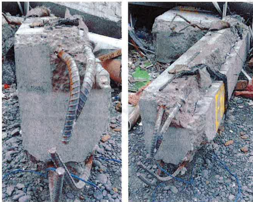
Figure 97 - Item E18 Pre-cast edge beam north-west corner (DENG B22 Dwg S18 (from left to right) (a) Smooth form finish at attachment to column 4A (DENG Detail 1 Dwg S19); (b) No starters (reinforcing bars) from pre-cast beam into slab to prevent the profiled metal deck slab pulling away (DENG Section 4 Dwg S15). If roughened these joints may have slowed down development of progressive collapse.
