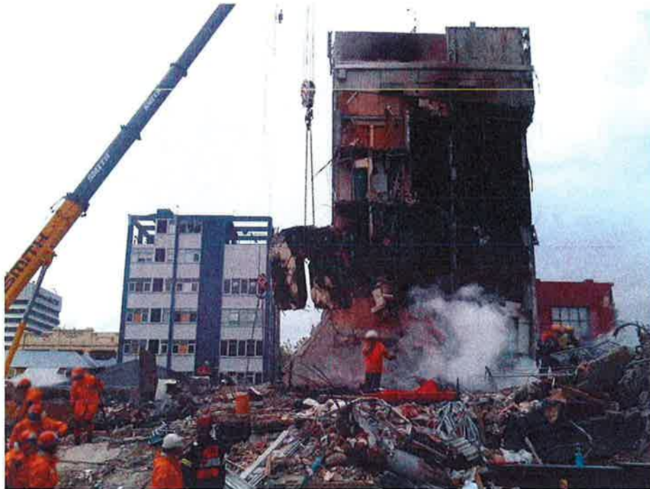
Figure 80 - Portion of Line 1 South Wall being lifted out by crane.. The Level 6 slab in front of North Core has been removed for safety reasons.
