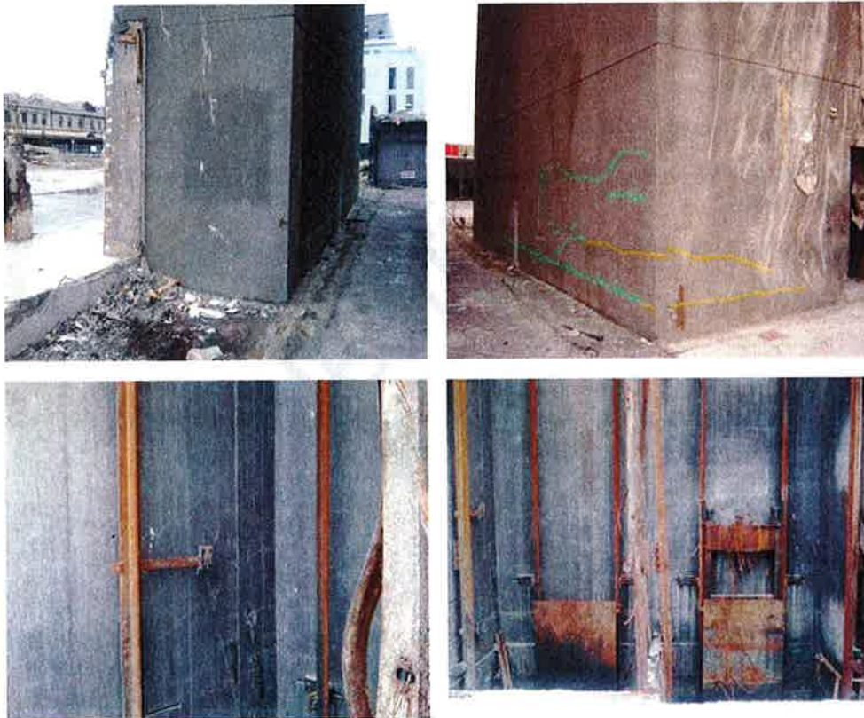
Figure 102 - North Core cracking (clockwise from top left) (a) No obvious cracking on Line D/E wall; (b) Horizontal flexural cracking on west and north west face of Line 5 wall and north end of Line C wall at Line C/5; (c) Fine two-way diagonal cracking on the inside faces of Level 1 to 2 Line 5; (d) and D walls in North Core.
