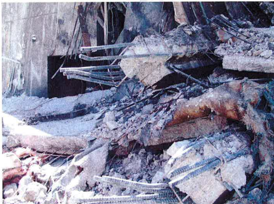
Figure 88 - Line 3 beams lying rotated southwards
