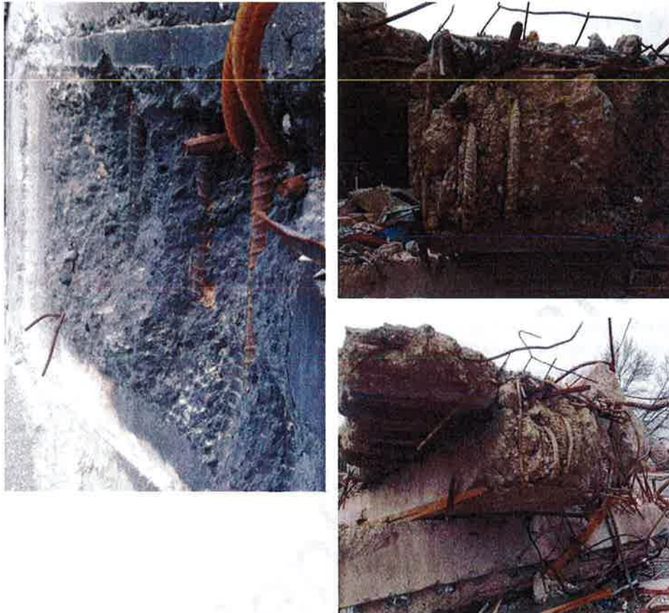
Figure 94 - Precast shell beam (Item E14) from northern face Grid 4, west side of North Core (DENG B23 Dwg S18). (clockwise from top right) (a) to (b) Fractured slab outstand remnant at east end from which slab concrete cores were extracted. The bottom H24 bars from shell beam have been turned back into the concrete infill rather than embedded in shear wall as specified (DENG Detail 5 Dwg S19). Notice the bar imprint on wall at the connection seen in (c) at Level 4 and at Level 3.. This meant that these beams would not have performed as intended.
