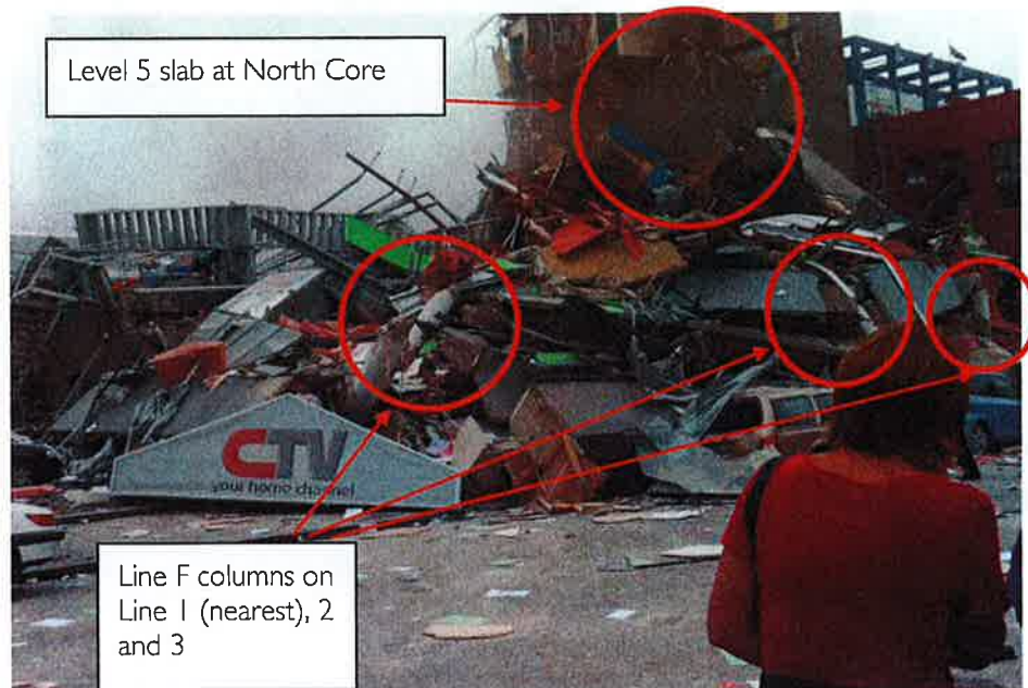
Figure 66 - Corner of Cashel and Madras Streets looking towards North Core. Fractured columns and fallen Spandrel Panels are visible (MSN photo).
