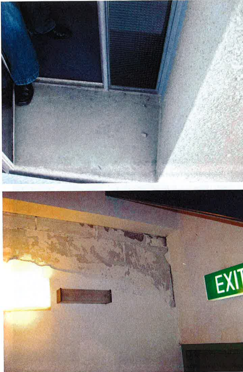
Figure 16 - (Top to bottom) (a) Fine cracking in floor at junction with South Wall; (b) Spalling of plaster finishes on internal masonry in-fill wall on Line 4 in front of stair well.
