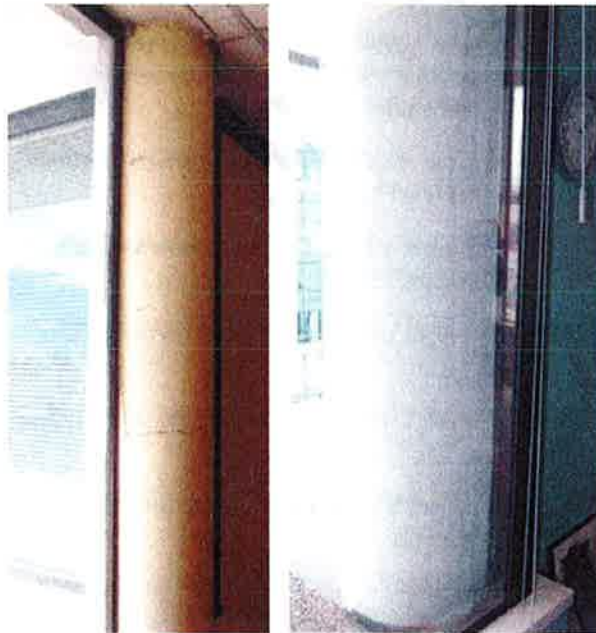
Figure 15 - Level 6 400mm diameter columns (Left to right) a) Column 4 D/E outside lift; b) Column on Line 1/A-B with hairline horizontal cracking.
