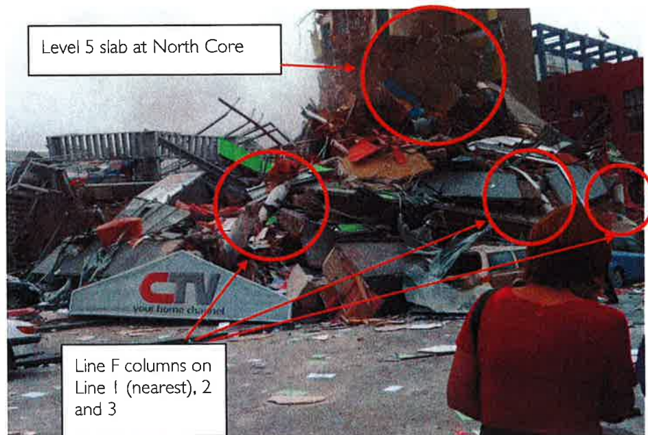
Figure 24 - Corner of Cashel and Madras Streets looking towards North Core. Fractured columns and fallen Spandrel Panels are visible (MSN photo).
