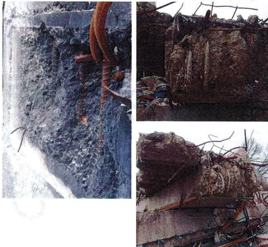
Figure 36 - Precast shell beam (Item E14) from northern face Grid 4, west side of North Core (DENG B23 Dwg S18). (clockwise from top right) (a) to (b) Fractured slab outstand remnant at east end from which slab concrete cores were extracted. The bottom H24 bars from shell beam have been turned back into the concrete infill rather than embedded in shear wall as specified (DENG Detail 5 Dwg S19). Notice the bar imprint on wall at the connection seen in (c) at Level 4 and at Level 3.. This meant that these beams would not have performed as intended.
