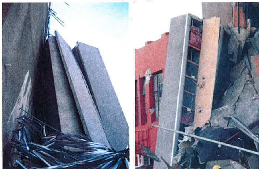
Figure 73 - Line 4 / B-C Spandrel Panels against tower wall, showing (left to right) a) View from north face; b) View from west showing timber framing for wall linings.
