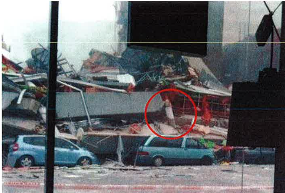
Figure 68 – View from looking west across Madras Street. A Line F/3 column is highlighted showing conical fracture in the painted portion above unpainted portion which had been enclosed by Spandrel Panels.
