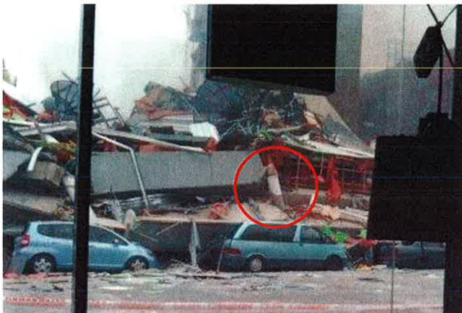
Figure 25 – View from looking west across Madras Street. A Line F/3 column is highlighted showing conical fracture in the painted portion above unpainted portion which had been enclosed by Spandrel Panels.
