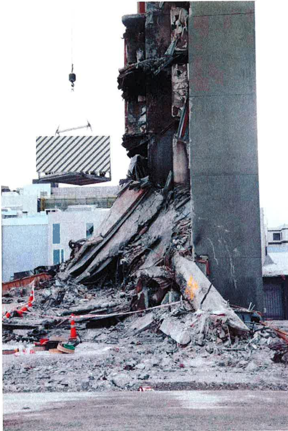
Figure 26 - North Core with Level 4 and 3 slabs laying diagonally against it.
