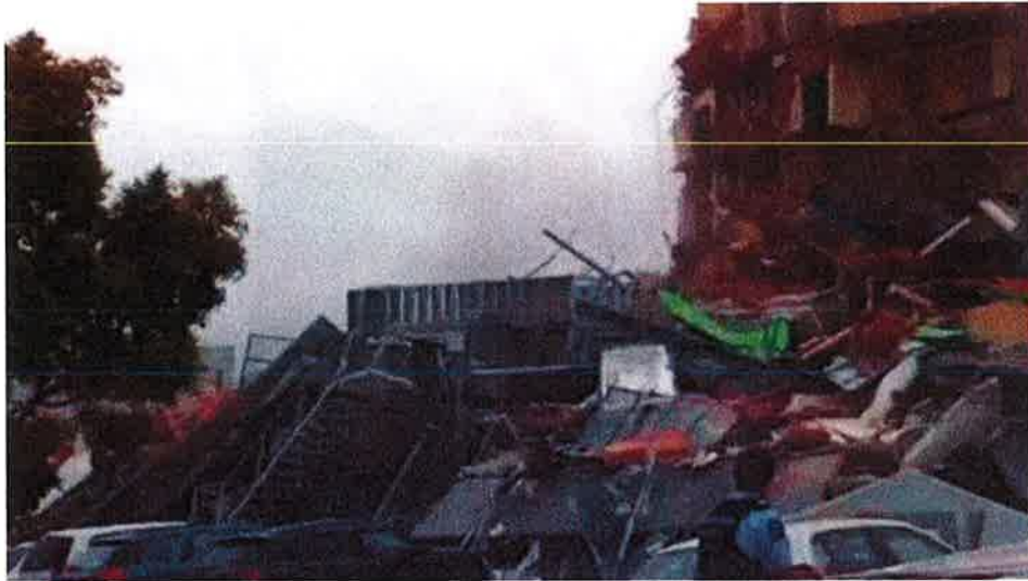
Figure 64 – View southeast corner of the CTV Building looking northwest. The South Wall collapsed onto the top of the debris from Level 2 can be seen, identifiable by the white fire escape stair still attached to it.
