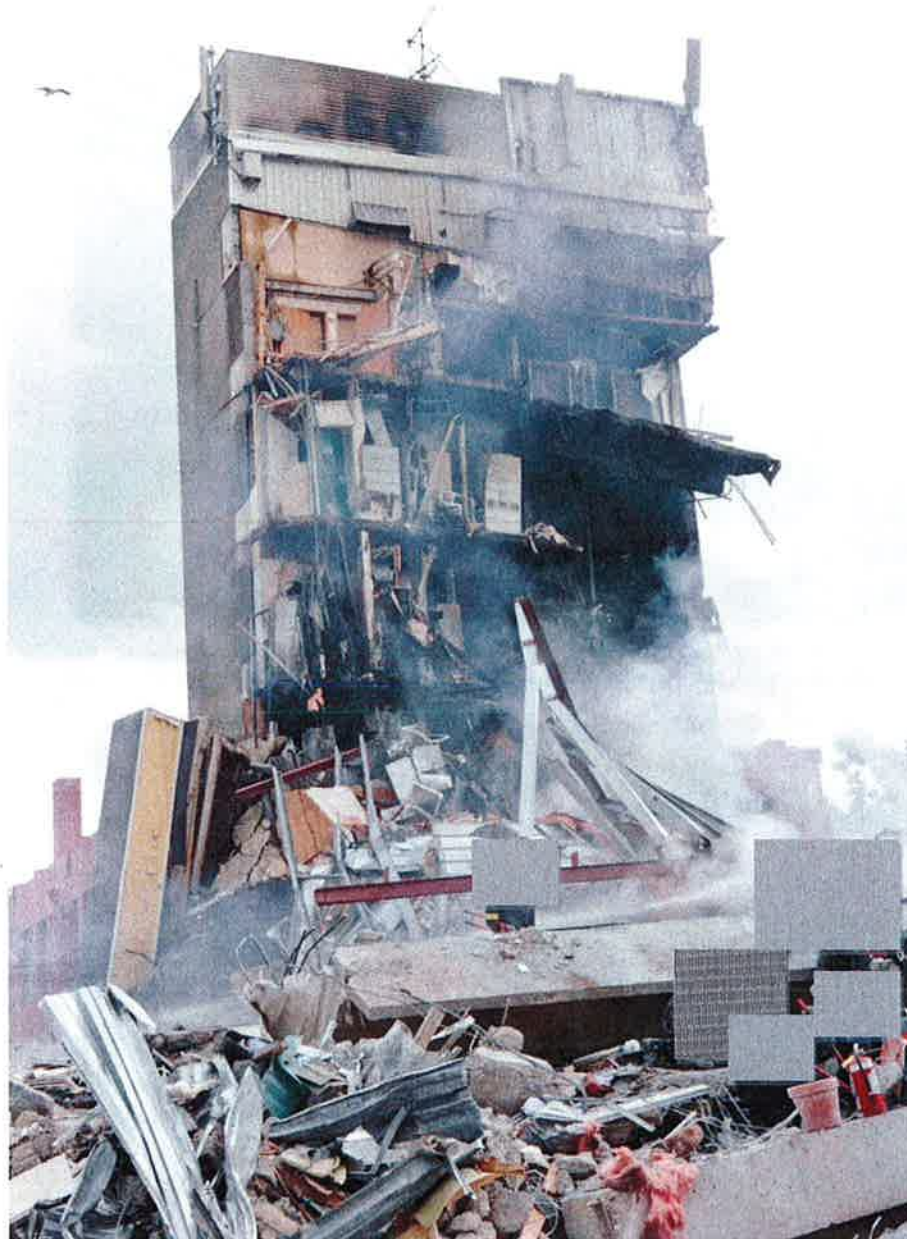
Figure 71 - Spandrel Panels and beams at Cashel Street Line 1 and on Line 4 in background standing vertical. Roof steelwork debris is visible.
