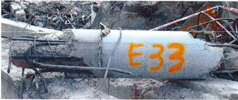
Figure 78 - Perimeter 400 mm diameter column with spalled base and bar lapping zone at left unpainted portion that would have been located at Spandrel Panel infill areas.
