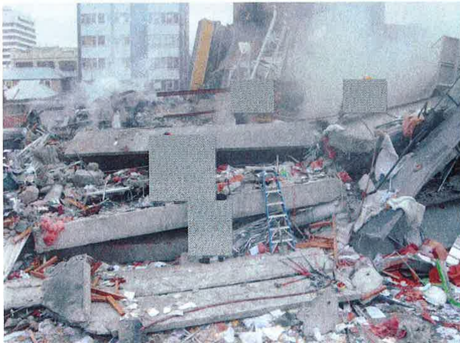
Figure 27 - Concrete Spandrel Panels, perimeter beams and columns on Cashel Street face (Line 1 / B-D).
