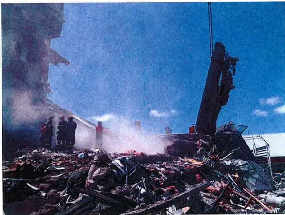
Figure 77 – Precast concrete beam being lifted from the debris near the South Wall.
