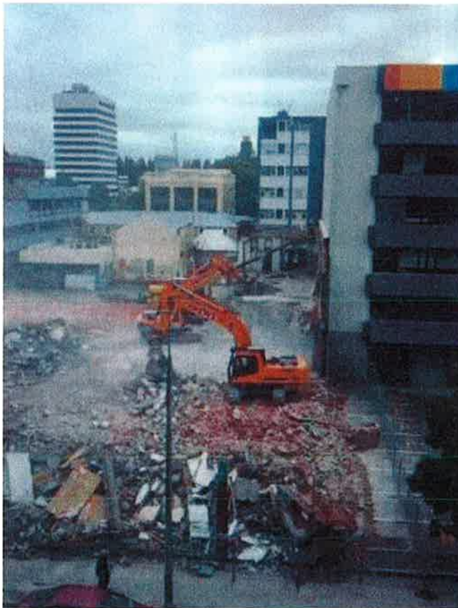
Figure 21 - Heavy machinery demolishing the building adjacent to the CTV Building after the 4 September Earthquake. The boundary wall is still in place covering the Line A infill masonry wall of the CTV Building.
