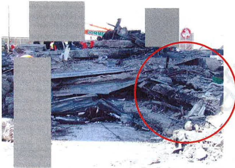
Figure 31 - Line 2 beams highlighted laying rotated northwards. This indicates that the Line 2 columns collapsed prior to the slabs breaking away from the Line 1 South Wall and frame.
