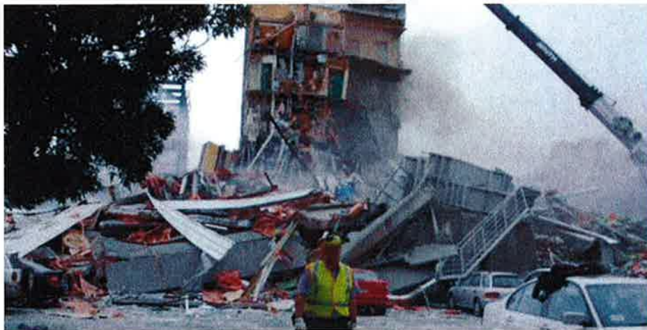
Figure 63 - Western end of south face (Line 1). Collapsed Line shear wall with escape stair to the right.
