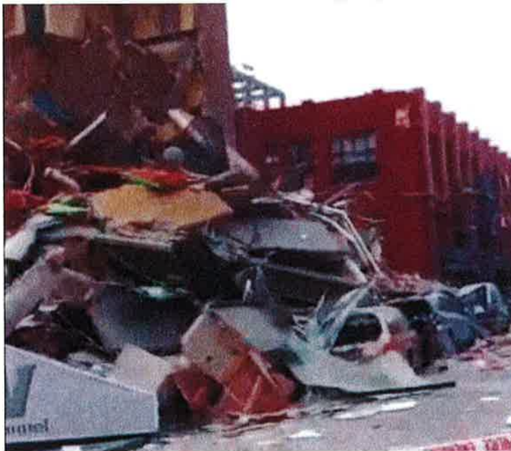
Figure 67 – View from southeast corner of CTV Building along Madras Street. This shows Line F Spandrel Panels fallen onto cars parked in the street indicating a tilt to the east during collapse.
