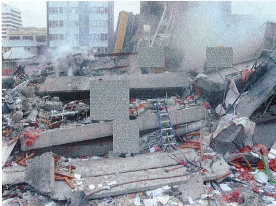
Figure 72 - Concrete Spandrel Panels, perimeter beams and columns on Cashel Street face (Line I / B-D).
