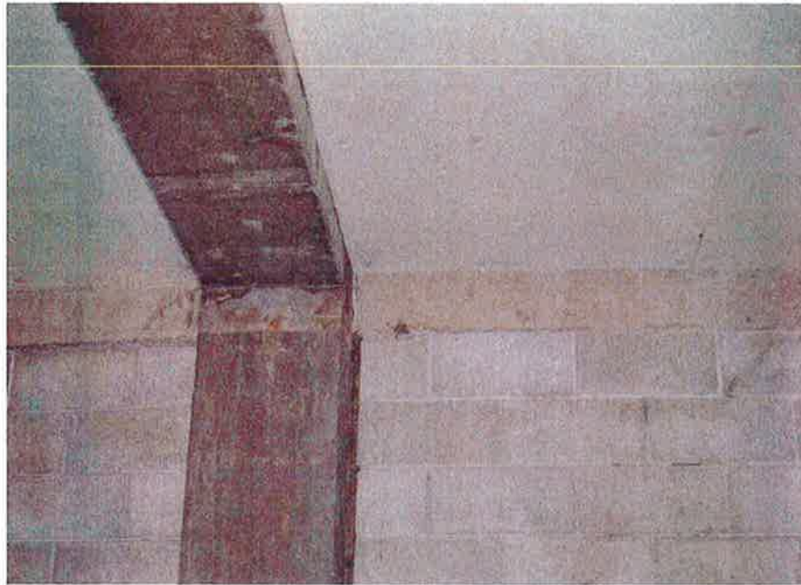
Figure 118 - Line A infill masonry wall adjacent to column with no obvious cracking after the 4 September earthquake. Flexible sealant is visible between masonry and column.
