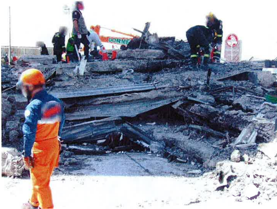
Figure 87 - Line 2 beams lying rotated northwards.
