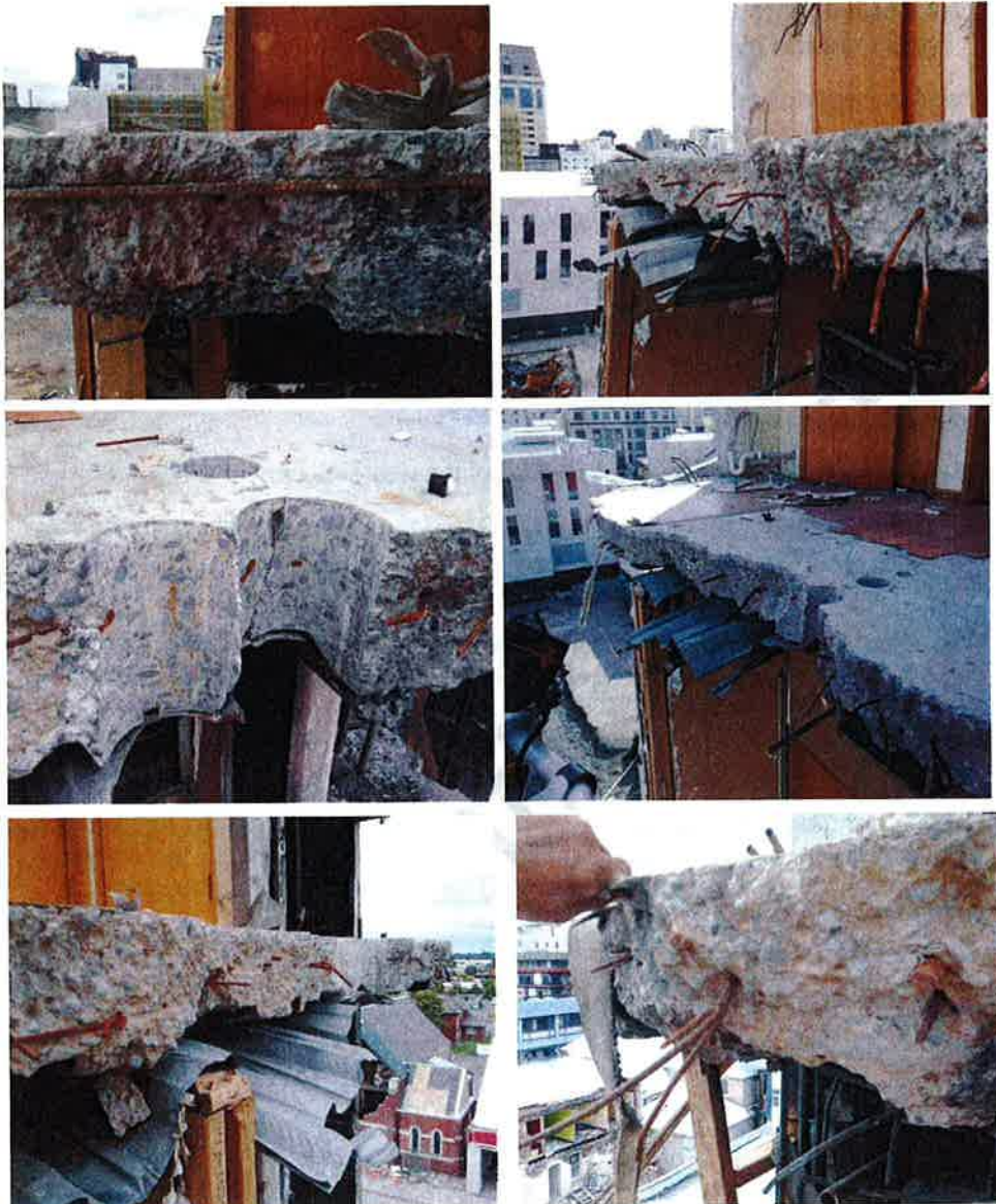
Figure 103 - Line 4 Core Wall Slab Remnant at Level 6 amenity area (clockwise from top left) (a) Slab edge on stairwell wall looking west with H12 saddle bar exposed and ends of mesh below it; (b) Vertical concrete fracture surface with reinforcing mesh fractured; (c) Slab looking west with cores cut in floor for amenities; (d) Fractured mesh angled downwards; (e) Fractured slab edge looking east. Torn metal decking aligned approximately with concrete fracture edge; mesh at varying height within slab; (f) Cores for amenities at fracture edge can be seen and are a small proportion of the total fracture surface length.
