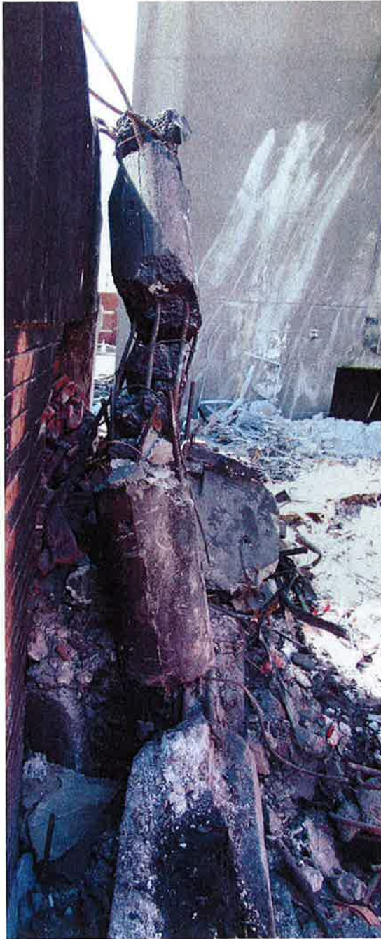
Figure 90 - Line 4 / B column with B22 precast log beam in foreground and B23 shell beam at rear. No hinging is apparent at the base of the column compared to the perimeter column Item E33.
