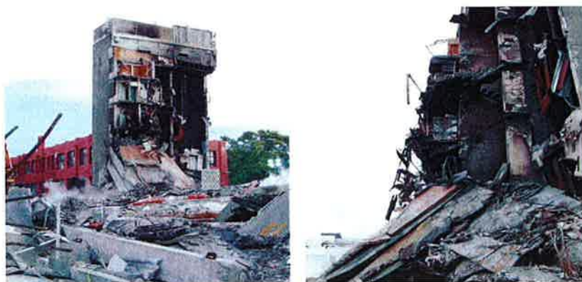
Figure 30 – View of North Core showing Level 4 slab lying diagonally on top of Level 3 slab. This indicates that the Level 3 and 4 slabs lost their vertical support on Line 3 prior to breaking away from the North Core.
