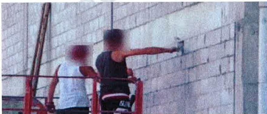
Figure 117 – Workers (including Eyewitness 16) hammering face of top course block away on west wall near Line A / 1 corner column. This indicates hollow blocks occurred in the top course and no separation joints on the outer face of the masonry.
