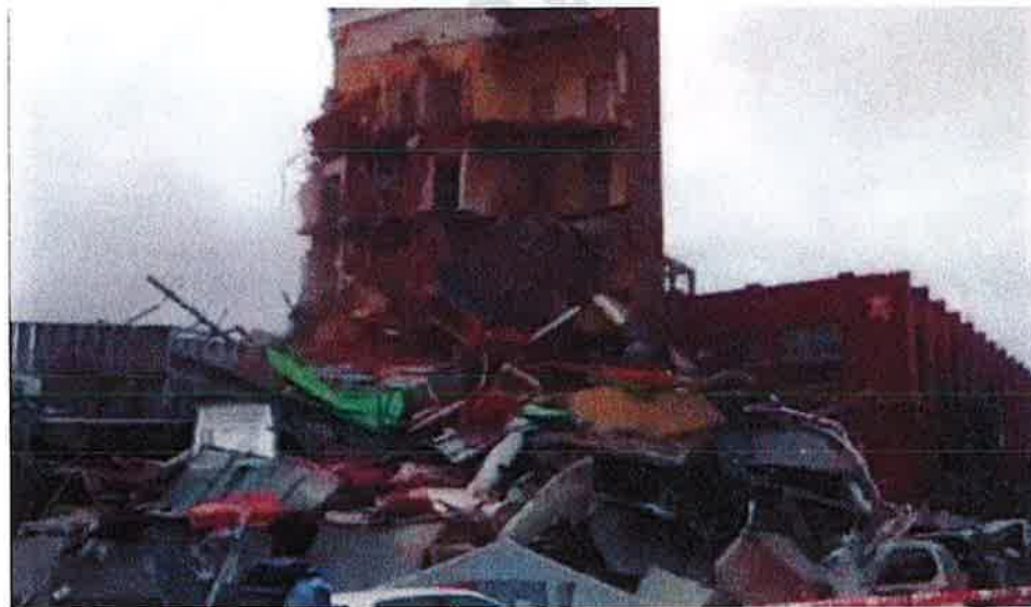
Figure 65 Madras St with precast Spandrel Panels fallen onto cars.
