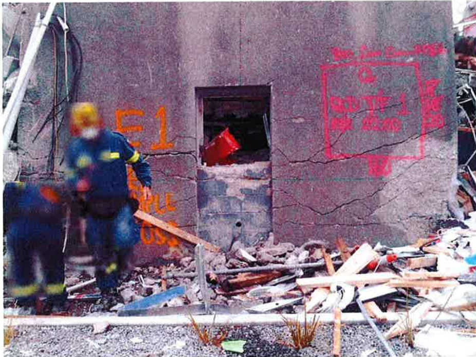
Figure 82 - Line 1 South Wall at Level 1 showing masonry in-fill at door opening, in-plane flexural fan-like cracking and spalling of concrete at right (east) end. A portion of profile slab can be seen end on through the opening
