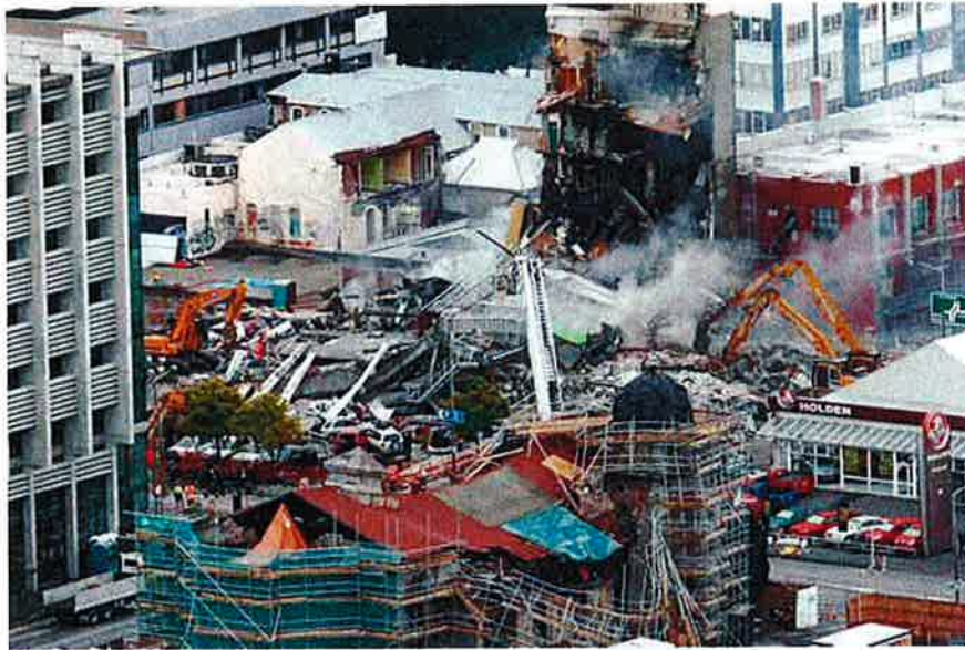
Figure 69 - Aerial view from southeast with debris being removed by heavy machinery. Fire has blackened the North Core. The Samoan church is damaged in the foreground (Dominion Post).
