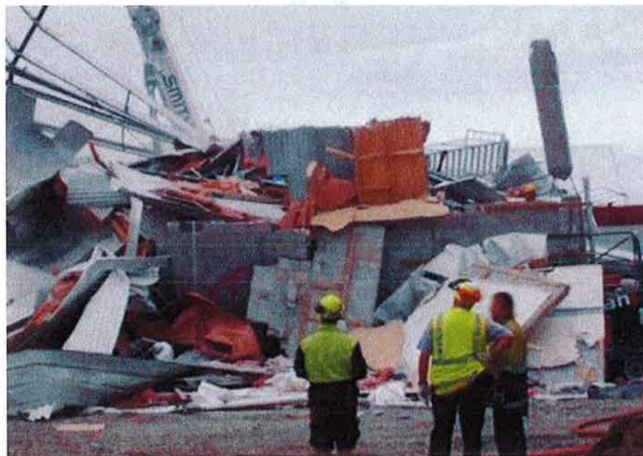
Figure 61 - Southwest corner (Grid A/1) with corner column still standing. Collapsed work platform under wall panels can be seen at the right on which Eyewitness 16 was working.
