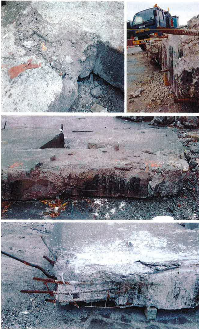
Figure 101 - Line 1 South Wall Level 5 to Level 6 (Item E5) (clockwise from top left) (a) Crumbly concrete at door edge of west pier able to be dislodged by boot; (b) Smooth and charred construction joint on top west surface looking east; (c) Charred construction joint above west pier. Door sill on left; (d); Top east corner with fractured top 3-H24 bars. Floor 664 mesh exposed.
