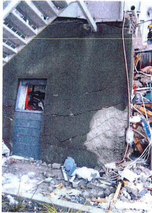
Figure 33 - Fan-like flexural cracking on the South Wall in conjunction with compressive spalling of the concrete at the wall east end. This indicates that the South Wall suffered flexural damage prior to the collapse of the floor slabs.
