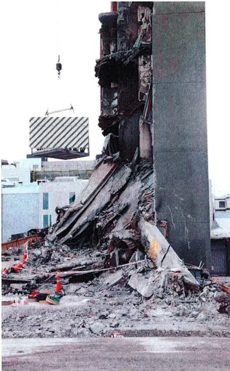
Figure 130 - North Core slabs leaning against the North Core showing that their collapse occurred after collapse of the Line 3 frame
