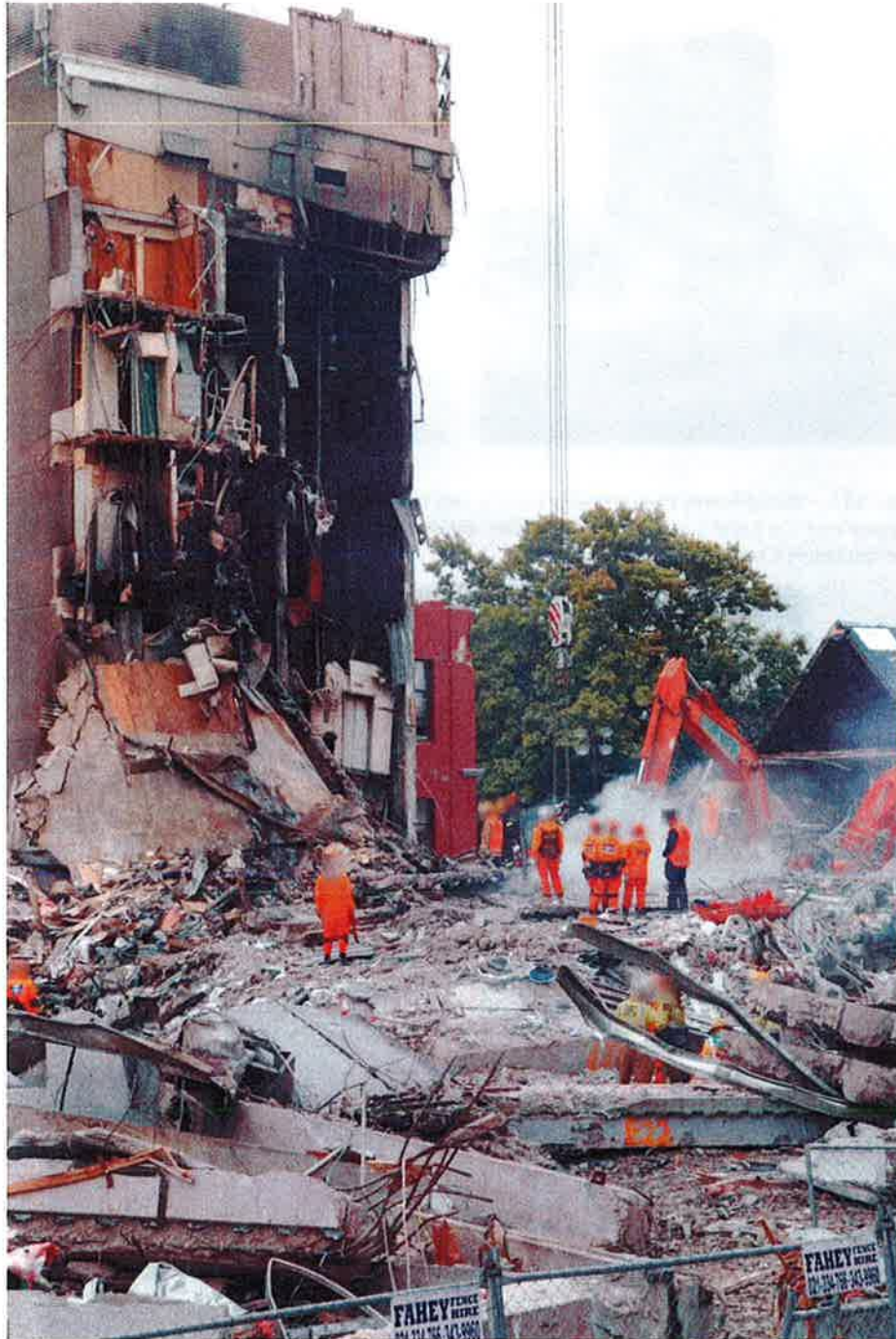
Figure 86 – View from southwest of North Core. The Level 4 slab can be seen lying diagonally against the North Core.
