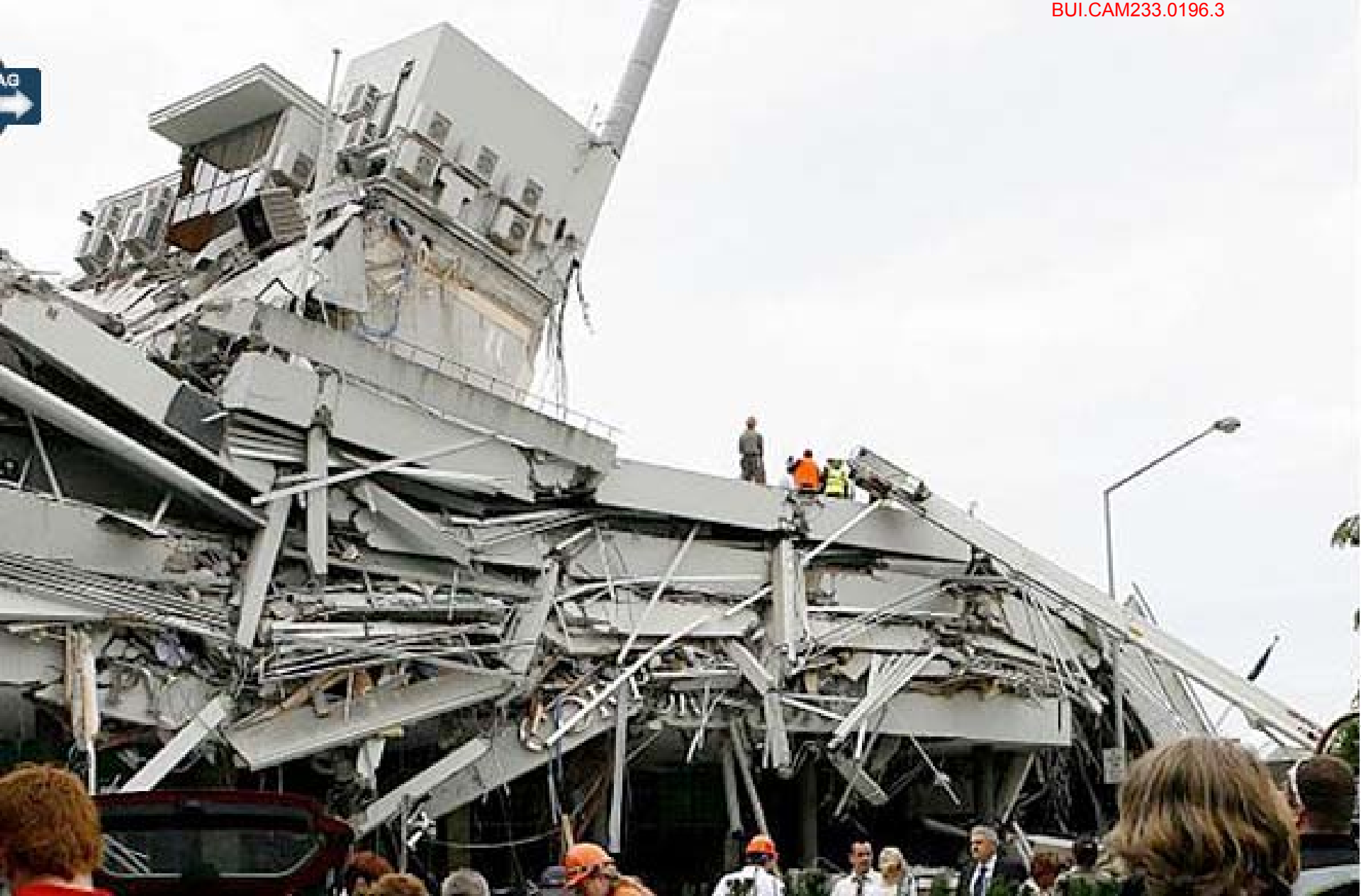
PGC BUILDING AFTER EQ
