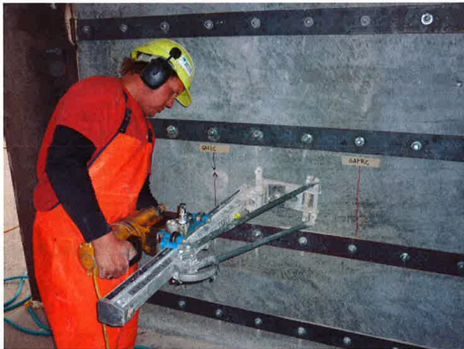
Figure 1 Drilling concrete core from Gallery Apartments
