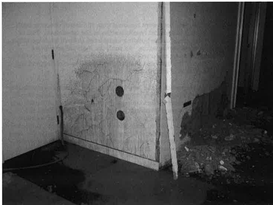
Figure 7 Core location on Wall element
