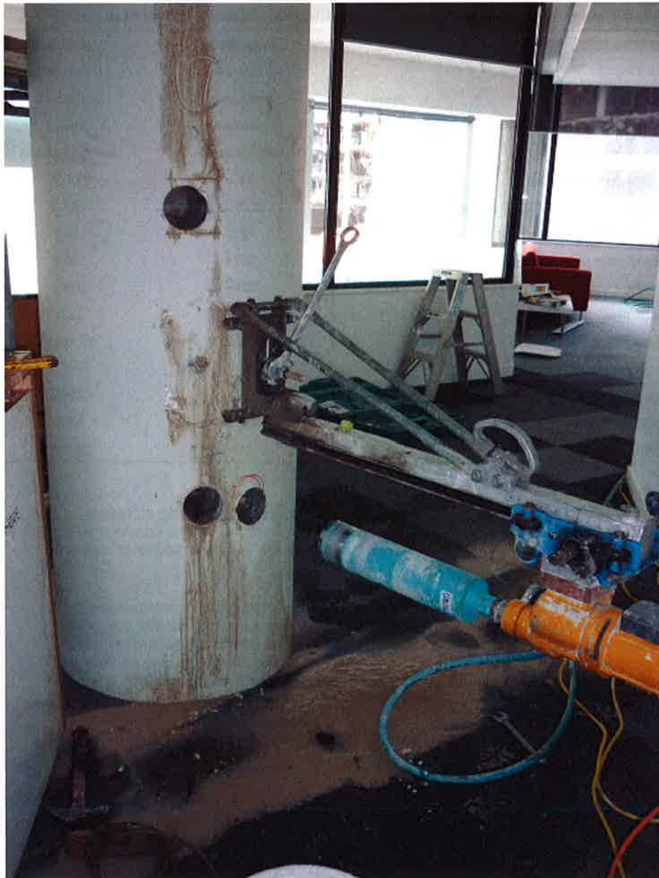
Figure 5 Core Drilling in concrete column
