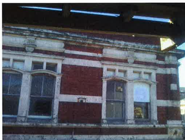
Figure 3 - 1st Floor Mollett Street Façade 15th September 2010
