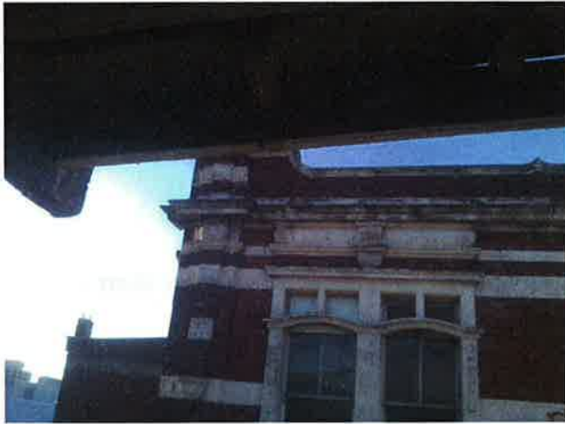
Figure 1 - 1st Floor Mollett Street Façade, 15th Sept 2010
