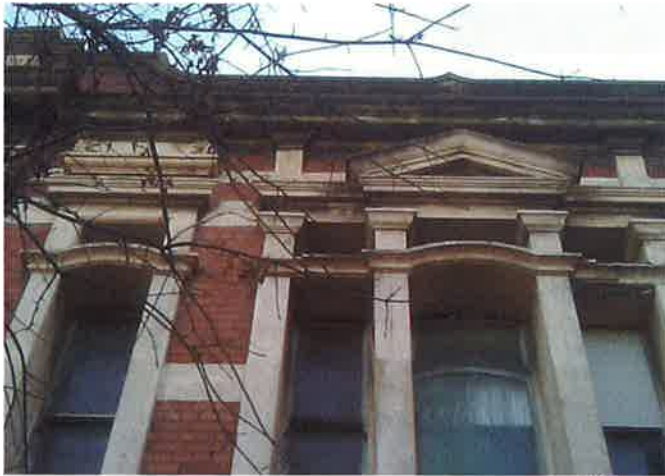
Figure 5 - 1st Floor Colombo Street Façade, 15 th September 2010
