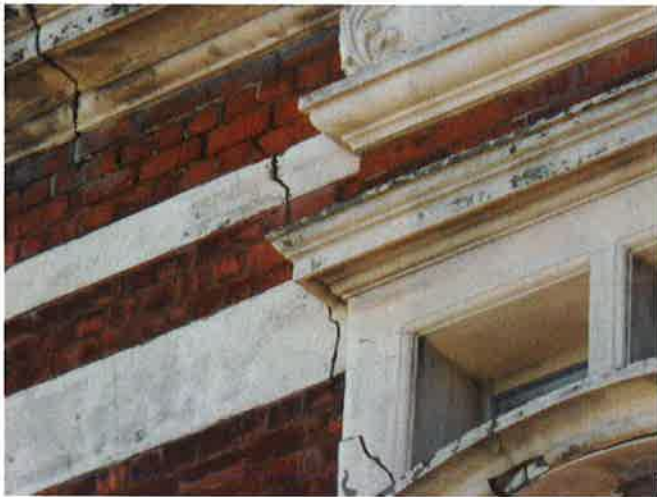
Figure 11 - 603 Mollett Street facade, 9th September 2010
