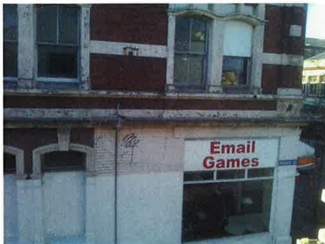
Figure 2 - 1st Floor Mollett Street Façade 15th September 2010
