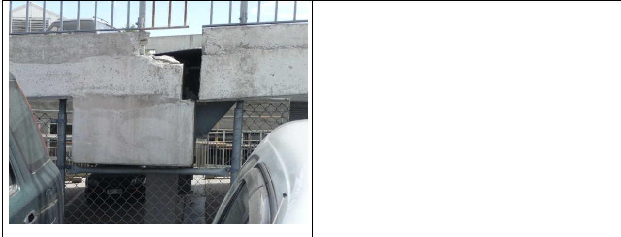
Figure 6: Parking garage on St Asaph St and Antigua St, Christchurch [Photos by M. Bruneau]; (a) Redundancy provided by multiple EBF bays; (b) Evidence of EBF link yielding; (c) Fractured link at lower level EBF; (d) Evidence of inelastic deformations at top level EBF; (e) Close-up view of same; (f) Displacement at expansion joint, top ramp.
