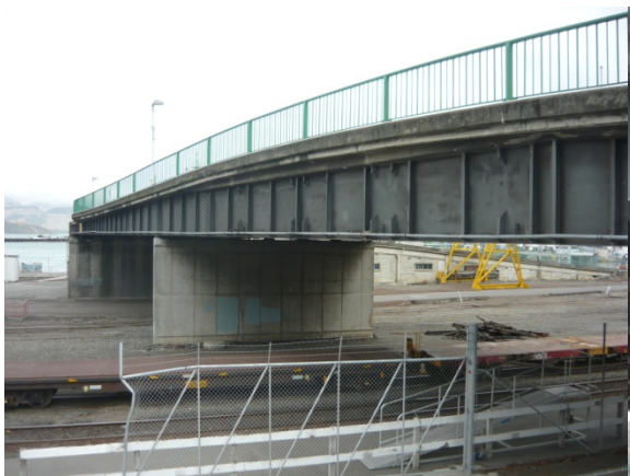
Figure 25 – Lyttleton Port Bridge (a) Plate Girder (b) Abutment Spalling (MacRae)
