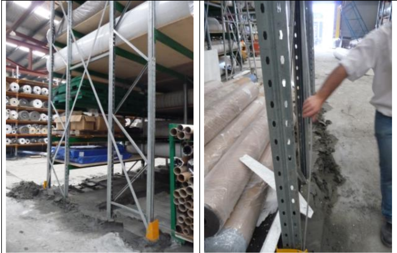
Figure 16: Industrial storage racks that survived, with evidence of soil liquefaction [Photos by M. Bruneau]; (a) Global view; (b) Close –up of buckled brace.
