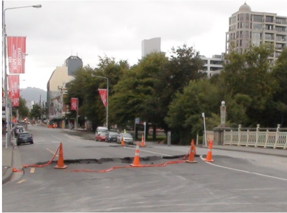
Figure 23 – Colombo Street bridge (a) Slumping of riverbank close to bridge; (b) Buckling of fascia arches; (c) Slumping of abutments at end of bridge; (d) Undamaged straight riveted girders. (Leon)
