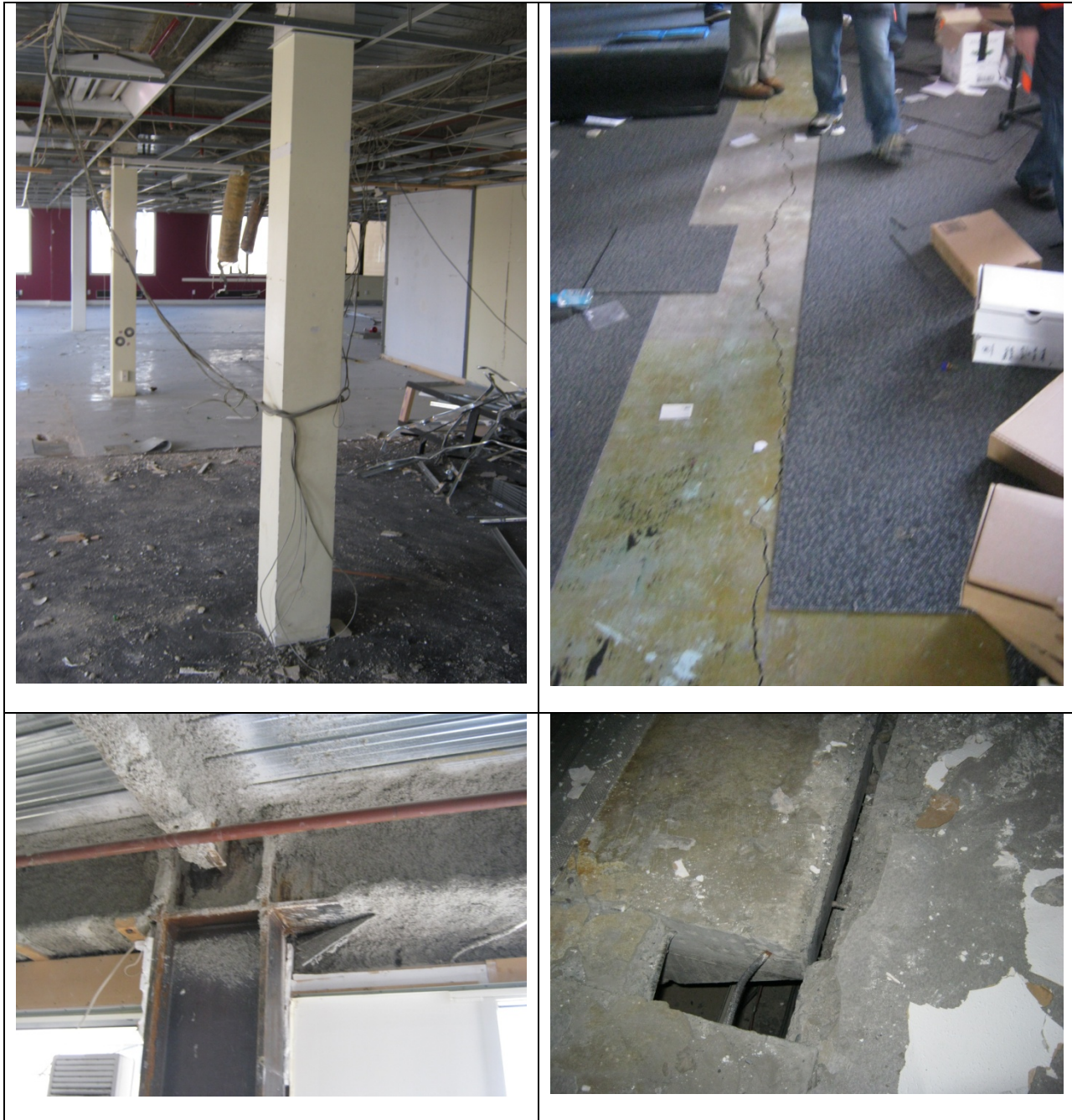
Figure 10: Seven storey PMRF building [Photos by C Clifton]: (a) Internal view of partially stripped floor; (b) Crack in ground floor slab where perimeter (to the right of the crack) has moved downwards relative to the core; (c) Typical beam to column connection with fire protection partially removed for inspection; (d) Gap opening in stair at landing due to lateral movement (stairs had independent structural support).
