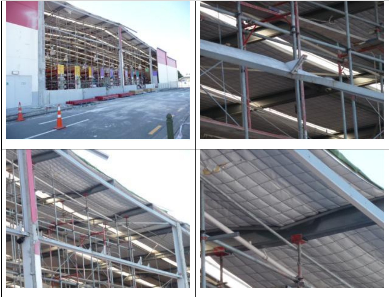
Figure 18: Failure of tilt-up panel connections [Photos by M. Bruneau]; (a) Global view; (b) Close –up view of fractures connection; (c) Global view of buckled beams; (d) Local view of one such beam.
