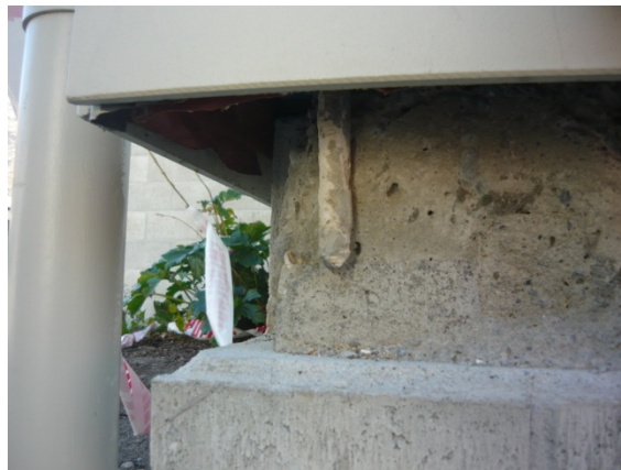
(a) Overall View from the South (b) Baseplate bolt at SE corner of the building Figure 20. Heathcote Valley Primary School Steel Moment Frame building (Photos: MacRae)
