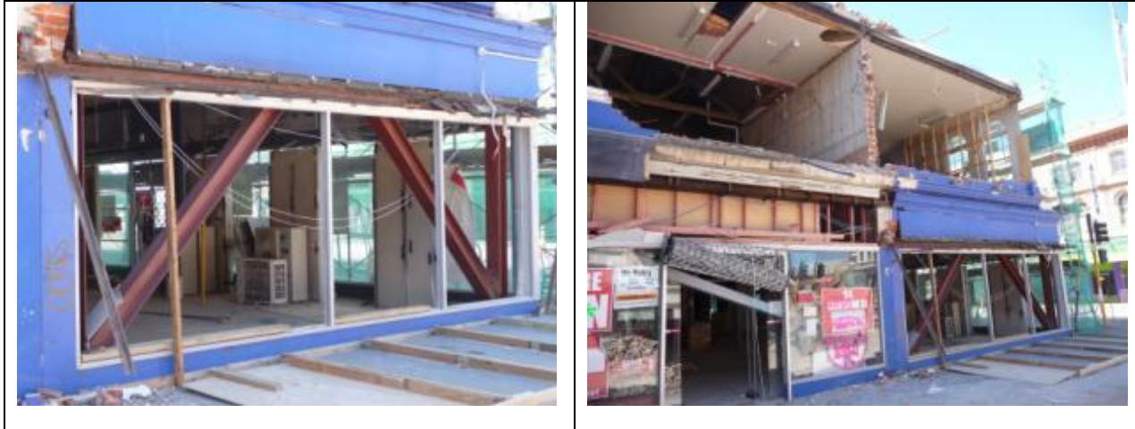
Figure 12: Braced frame as a retrofit to unreinforced masonry building [Photos by M. Bruneau and C Clifton]: (a) Close-up view; (b) Global view.
