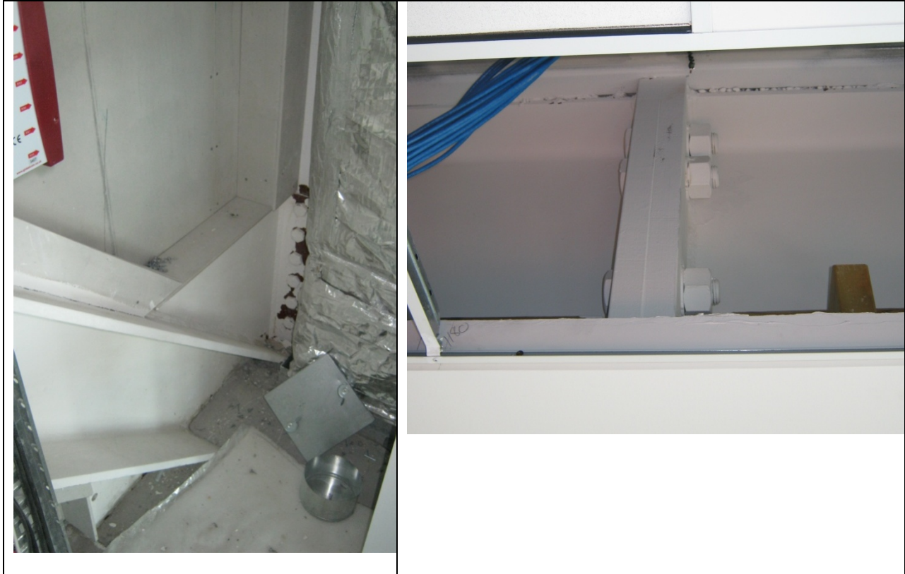
Figure 7: Connections in Club Tower Building, Christchurch [Photos by G C Clifton]; (a) Brace/beam/column connection showing out-of-plane yielding in endplate but no inelastic demand in gusset plate; (b) Flush moment endplate splice connection
