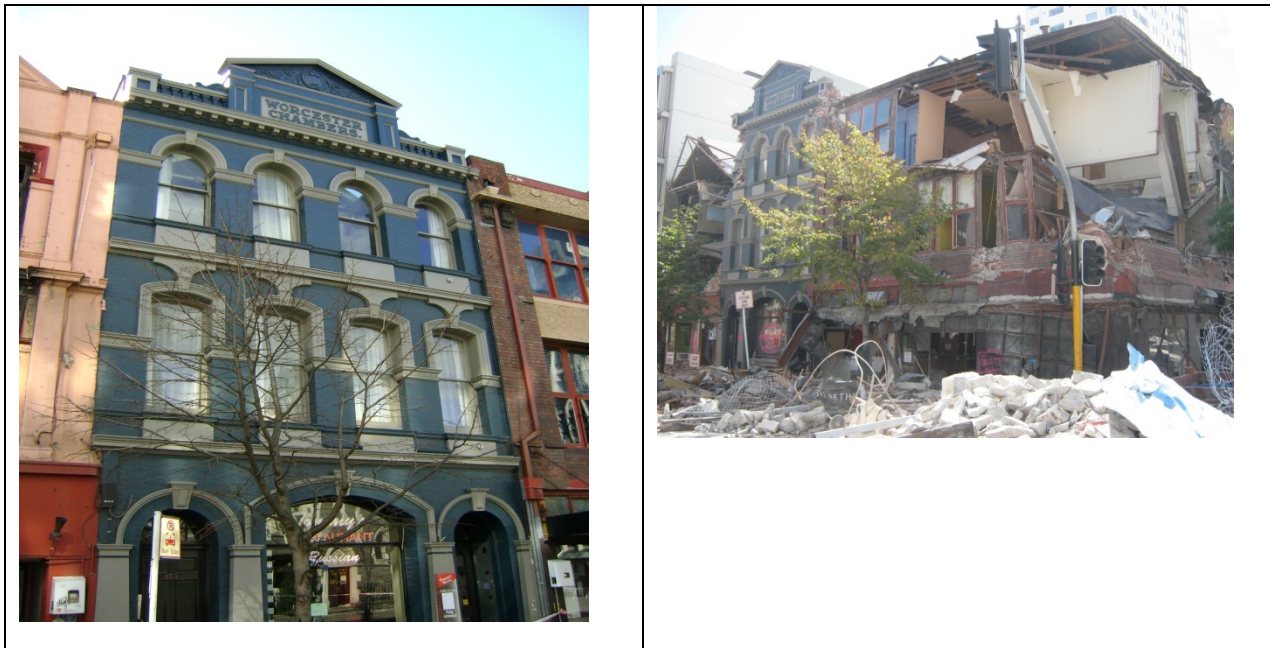
Figure 13: Strengthened URM buildings[Photos by C Clifton]: (a) is following the September 2010 event and (b) following the February 2011 event, taken from a slightly different view-point.
