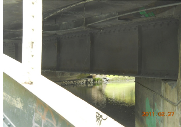
Figure 23 – Colombo Street bridge (a) Slumping of riverbank close to bridge; (b) Buckling of fascia arches; (c) Slumping of abutments at end of bridge; (d) Undamaged straight riveted girders. (Leon)
