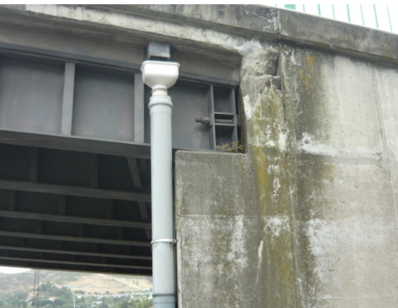
Figure 25 – Lyttleton Port Bridge (a) Plate Girder (b) Abutment Spalling (MacRae)
