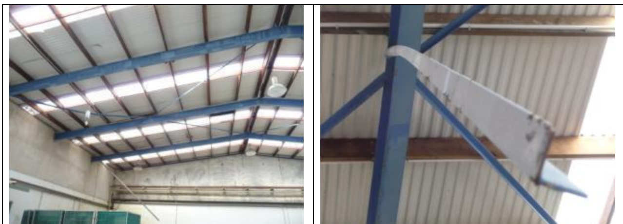
Figure 17: Industrial facility roof bracing [Photos by M. Bruneau]; (a) Global view, showing buckled brace
