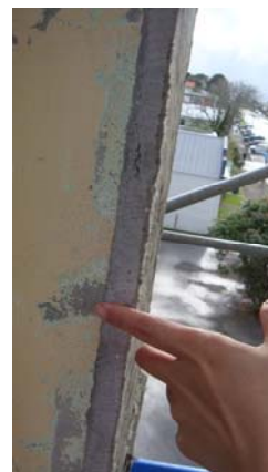
(b) Fibre reinforced shotcrete applied to the exterior surface of a chimney
