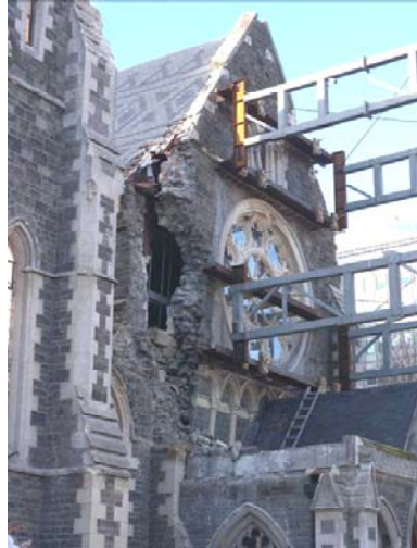
(a) unstable front wall
