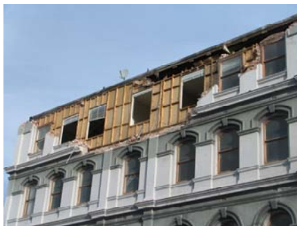
(a) Wall damage at 140 Linchfield Street
