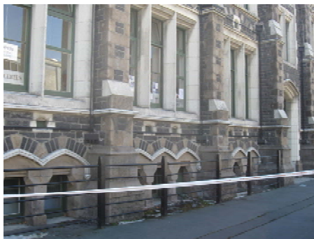
(a) External post-tensioning used in the Christchurch Arts Centre (photo taken after 22 February 2011 earthquake)
