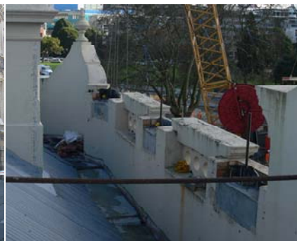
(b) Internal post-tensioning bars used in the Birdcage hotel, Auckland
