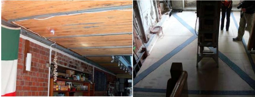
(a) Steel sections added to stiffen and secure the floor diaphragm
