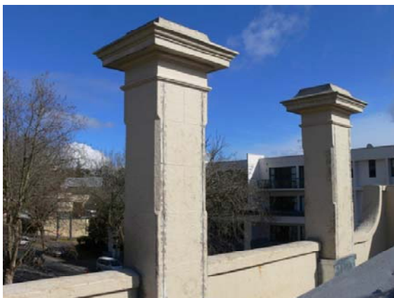
(a) Vertical Near Surface Mounted (NSM) Fibre Reinforced Polymer (FRP) strip strengthening of chimneys
