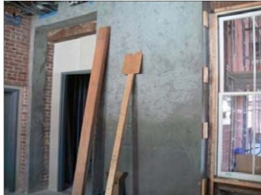
(a) Internally applied shotcrete to a URM building located in San Francisco
