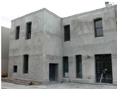
(a) Shotcrete applied to a former URM building
