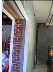
(b) Shotcrete applied to a URM building located in San Francisco
