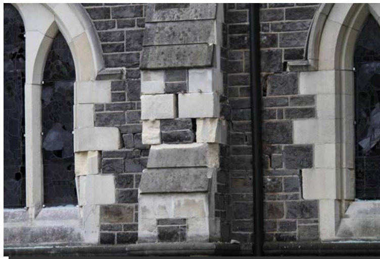
Figure 3.34 Christchurch Anglican Cathedral - diagonal cracks in the south façade piers
