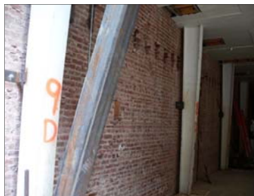
(b) Steel moment frames used in a multi storey URM building in San Francisco
