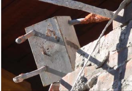
(a) Poor installation of adhesive anchors
