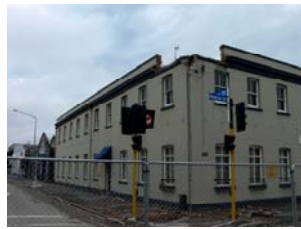
(b) Exterior view of failed parapet at corner
