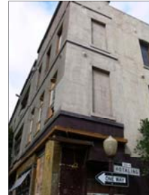
(c) Externally applied shotcrete to a URM building located in San Francisco
