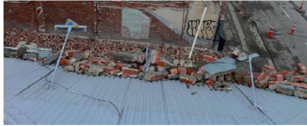
(a) Roof level view of failed parapet restraint
