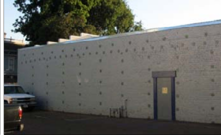
(b) Addition of internal strong-backs and extensive anchorage of masonry, San Louis Obispo
