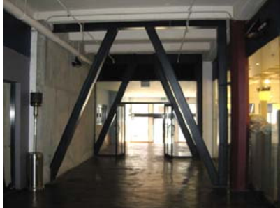
(a) Eccentric bracing in a walkway
