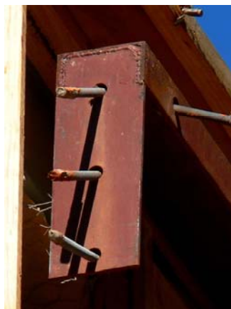
(a) Failure of a steel fixing due to anchor withdrawal
