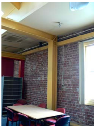
(a) Post-earthquake condition of a URM building having an internal steel frame retrofit
