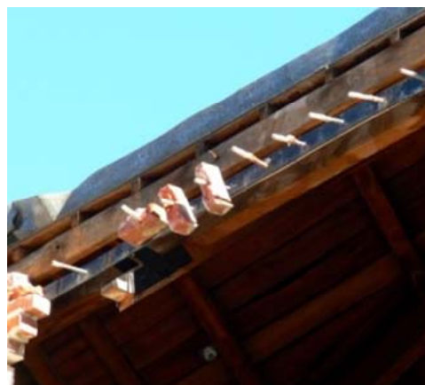
(b) Failure of a steel fixing due to both anchor withdrawal and brick detachment
