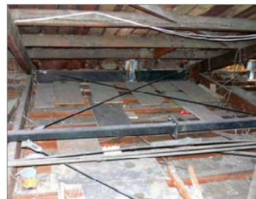
(b) Roof diaphragm improvement using steel braces
