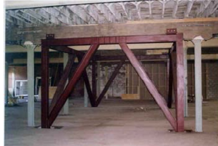
(b) Eccentrically braced core
