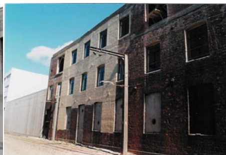
(b) Surface bonded FRP applied to the exterior of a URM wall
