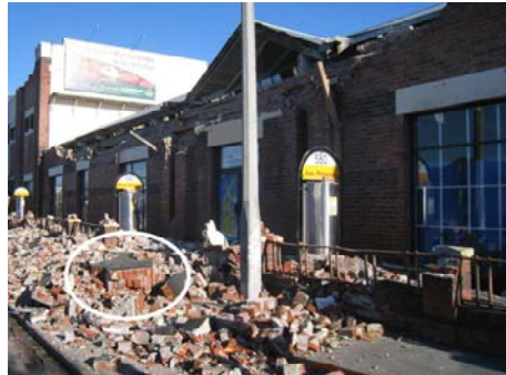
(a) Solid section of masonry gable
