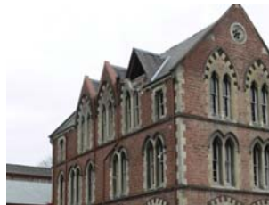
(c) Montreal-Armagh street corner
