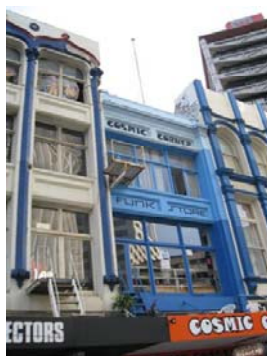
(a) Building overview
