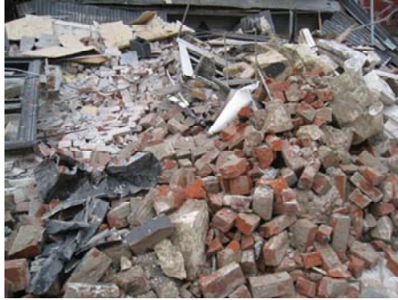
(a) Masonry rubble showing 'clean' bricks
