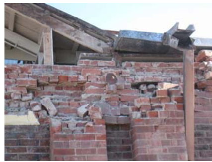
(b) Wall anchor still intact (see also Figure 6a).
