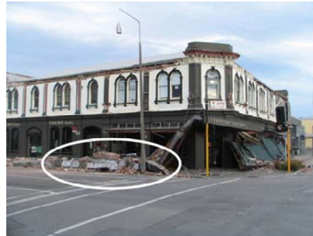
(b) Solid section of parapet
