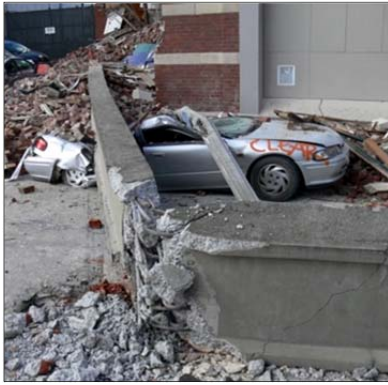
(a) Collapse of concrete capping beam used to replace the original masonry parapet
