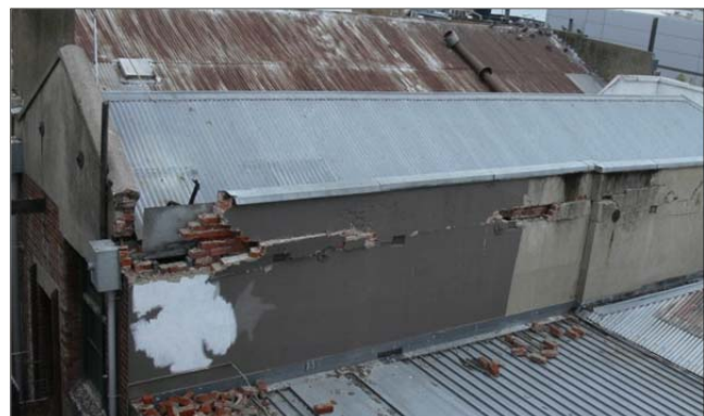
(b) Heavy damage to parapet
