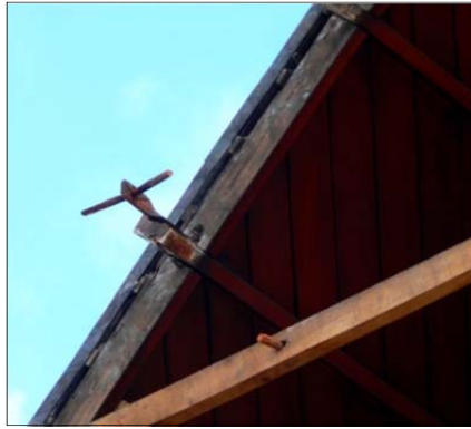
(a) Restraint used at the time of construction
