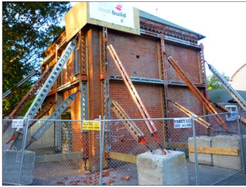
(a) Extensive steel temporary shoring of a URM building following 4 Sept. 2010 Darfield earthquake, (building located outside CBD)
