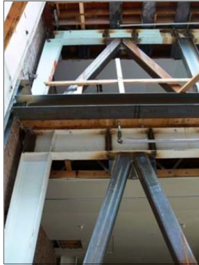
(a) Steel k-brace frames used in a multi storey URM building in San Francisco
