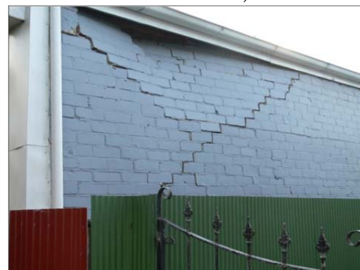
(f) Two-way bending out-of-plane wall failure
