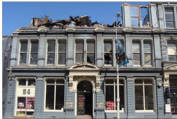
(d) Complete collapse of top storey due to weak piers, 84 Lichfield Street
