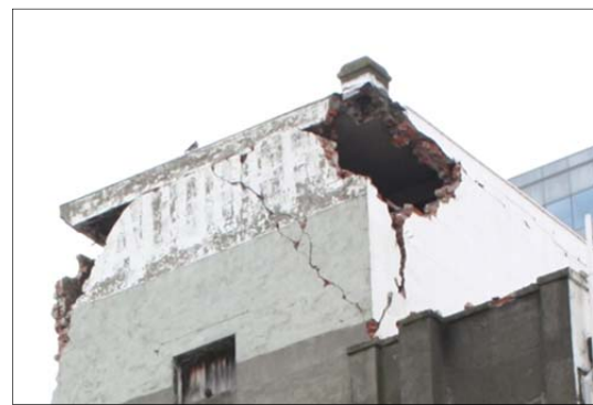
(b) Corner failure
