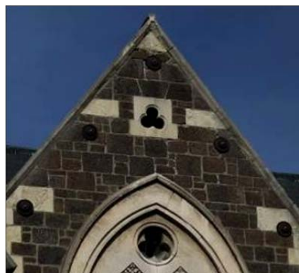
(c) Example of through tie anchorage
