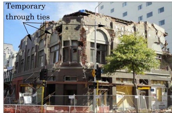
(b) Temporary securing work on a URM building following 4 Sept. 2010 Darfield earthquake, corner of Gloucester and Manchester Street
