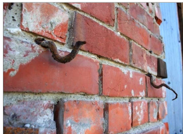
(b) Metal cavity ties in poor rusted condition
