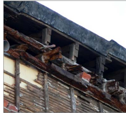
(b) Example of poor roof diaphragm condition
