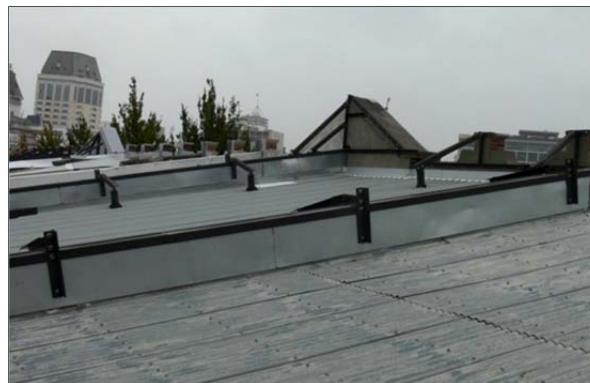
(e) Steel angels 'confining' the parapet and securing it back to the roof via rigid braces
