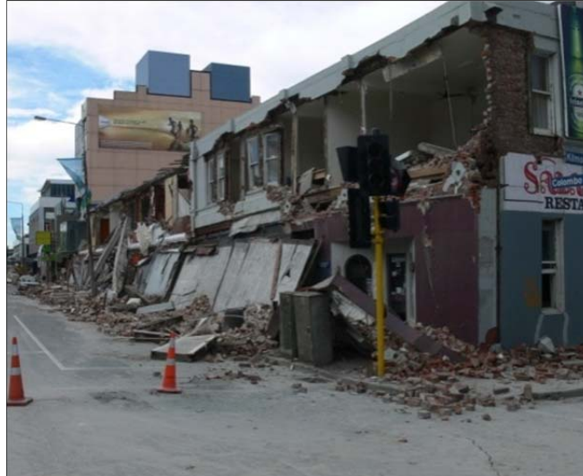
Figure 3.6 Collapse of awnings due to falling debris, at the corner of Colombo and Kilmore Streets looking north-east
