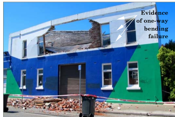
(d) One-way out-of-plane bending wall failure below a concrete ring beam (building located outside CBD)
