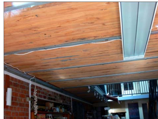
(d) Floor diaphragm improvement using overlays and steel framing
