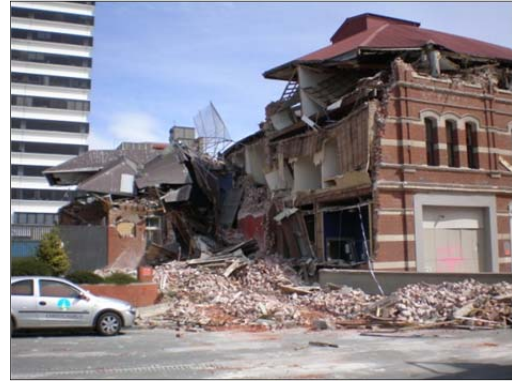
(b) Partially collapsed building poses a near certain risk to building occupants and to public space, 194 Gloucester Street
