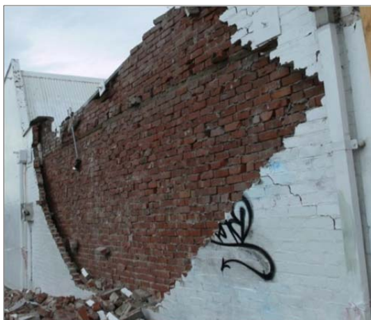
(a) Out-of-plane failure of a single leaf veneer
