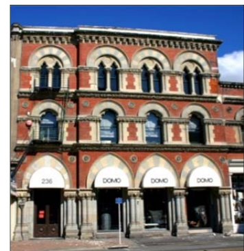
(c) Perforated masonry frame, 236 Tuam Street
