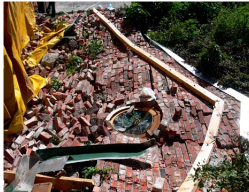
(d) Gable collapse due to inadequate connections
