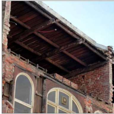
(a) Example of fair roof diaphragm condition
