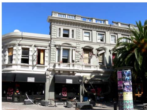
(c) Damage classification - Heavy Damage level – C (120 Manchester Street)
