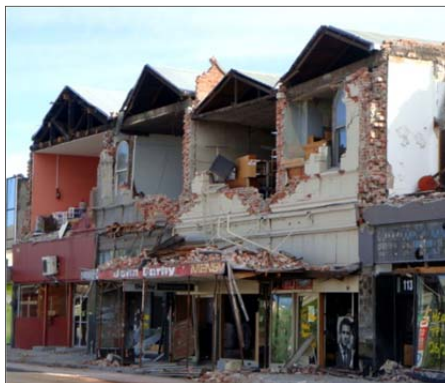
(c) Out-of-plane collapse of parapet and facade, 105 -109 Manchester Street
