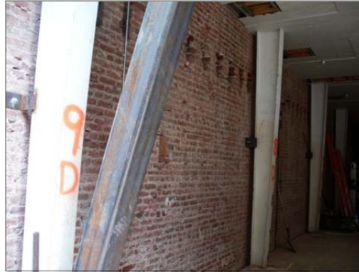
(b) Steel moment frames used in a multi storey URM building in San Francisco
