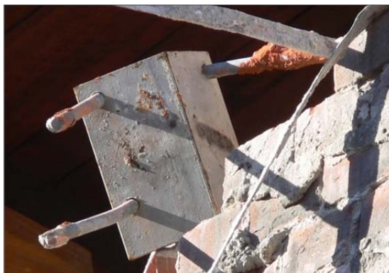
(a) Poor installation of adhesive anchors
