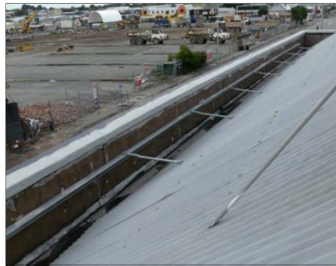
(d) Parapet restraint using rigid steel braces connected to a continuous steel section
