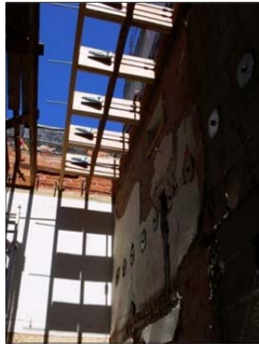
(a) Extensive addition of wall-to-diaphragm anchorage, San Louis Obispo
