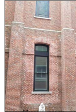
(c) Reduction of window opening to increase in-plane wall capacity
