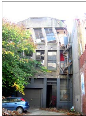
(c) Weak piers, pier rocking, 82 Lichfield Street
