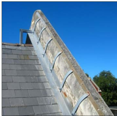
(c) Well restrained parapet
