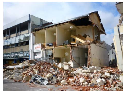
(d) Damage classification - Destroyed Damage level – D (202 Hereford Street)
