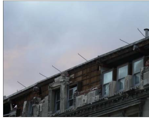
(b) Thin and flexible restraint rods failed to restrain the parapet
