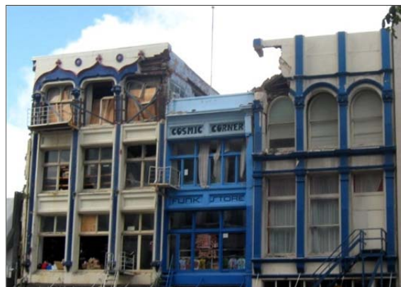
Figure 3.13 Example of building pounding causing in-plane failure, High Street
