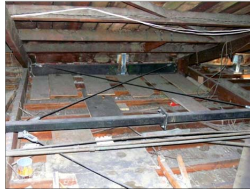
(b) Roof diaphragm improvement using steel braces
