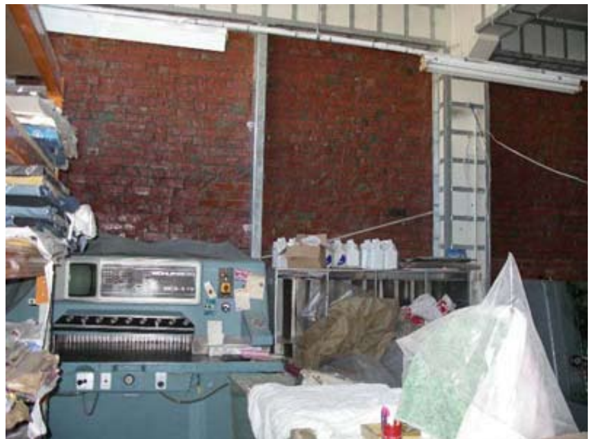
Finished wall with strengthening.
