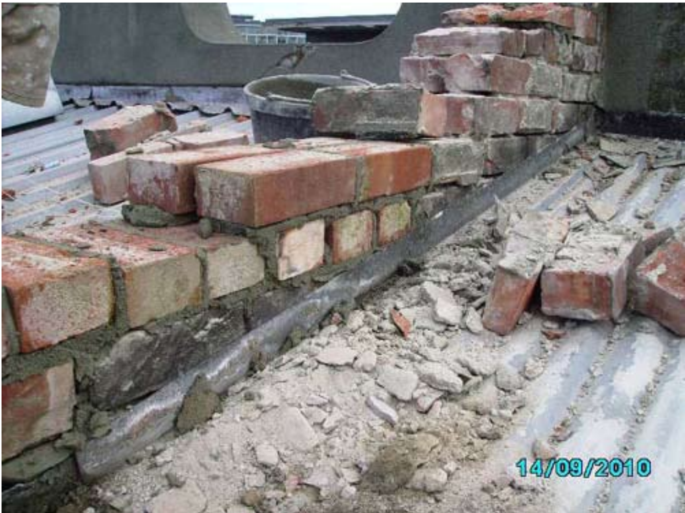
Party wall at roof level before strengthening
