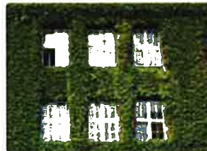
Above: A green wall reduces off site stormwater runoff and contributes to building insulation.
