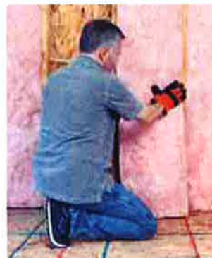
Left: Insulation installed during construction
