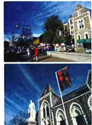
Above: Significant heritage buildings where repairs are underway - The Arts Centre, Worcester Boulevard and Canterbury Museum, Rolleston Avenue.
