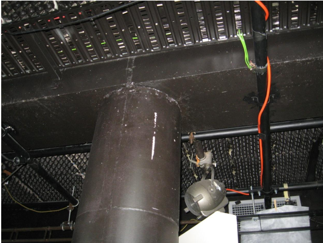
Photo 7 Internal beam column joint under first floor – no evidence of damage.
