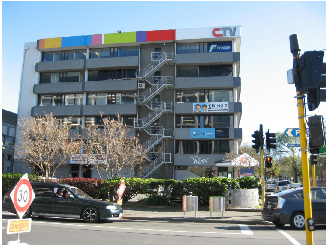
Photo 1 South Elevation of Building
