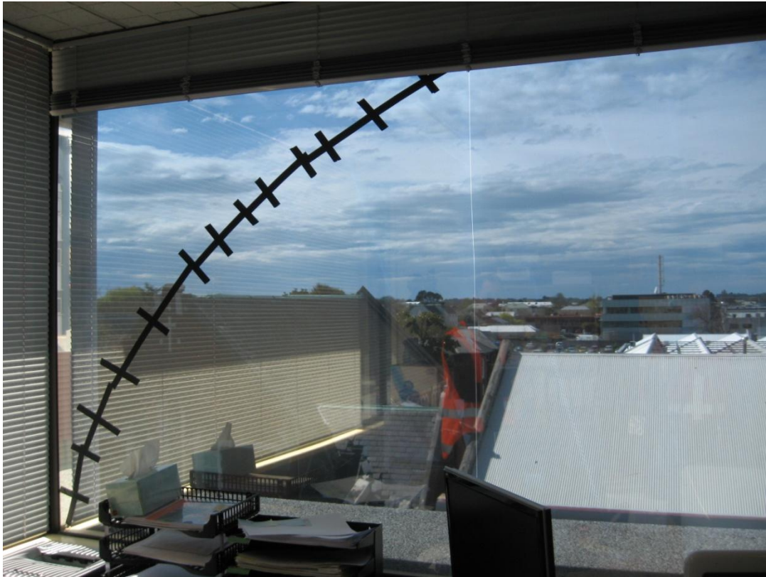
Photo 15 Broken window.
