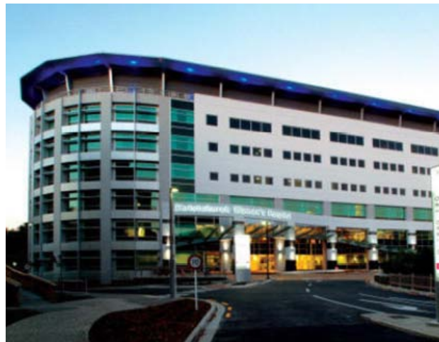
Figure 2: Christchurch Women's Hospital sits on Lead Rubber base isolators.
