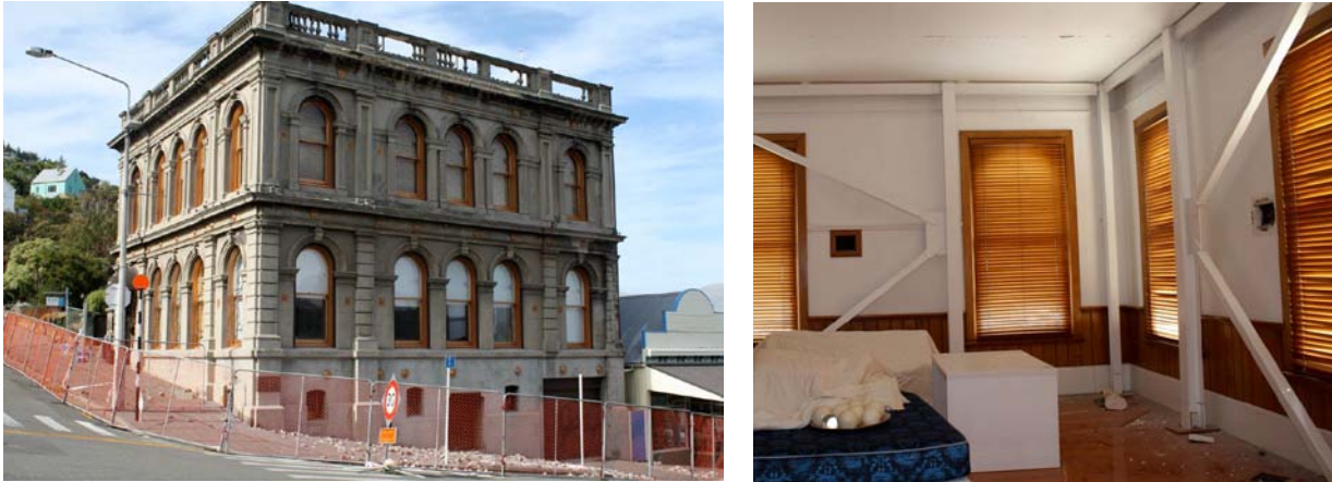
Figure 4: The Lyttelton Fire Station building suffered only minor damage as it has been strengthened with an internal steel frame (Photos Win Clark)
