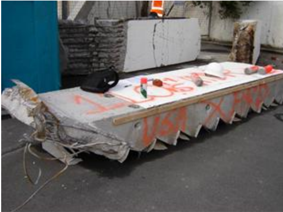
Figure 18 - Unit 3 with upper landing; Unit 1 to left behind; Unit 2 to right behind
