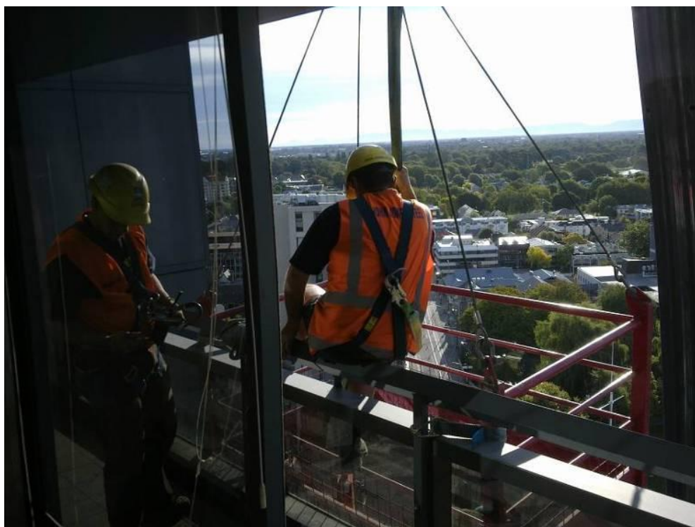
Figure 5 –Crane access into building
