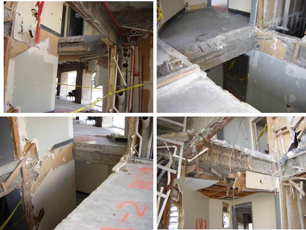
Figure 14 – Level 2 to 3 Stairwell in the access area used for remnant retrieval
