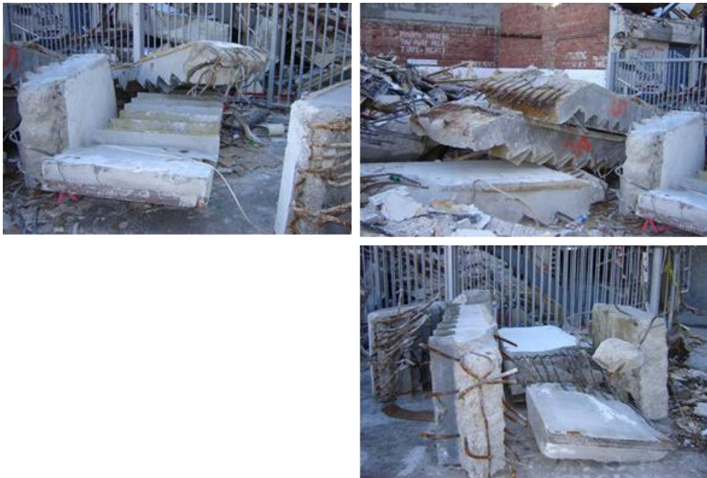
Figure 34 – Other stair remnants.
