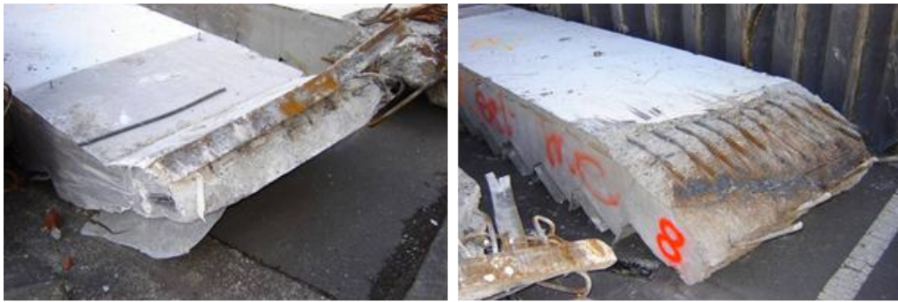
Figure 23 - Unit 8 (left to right): (a) 300 mm long upper landing with 45 degree shear crack and damaged seating angle. Fractured D20 bar remnants in end face; (b) Gas cut mid-height landing b.
