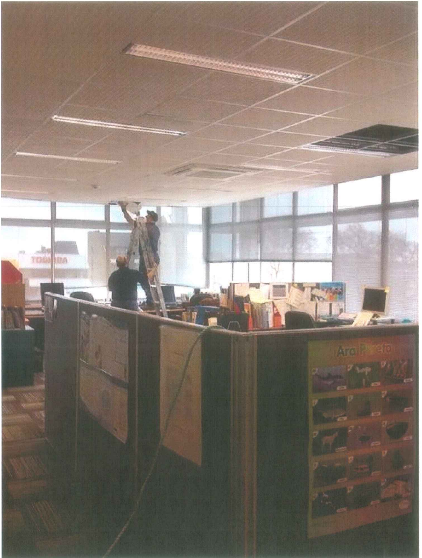
Pac BLDG Sept 2010.
