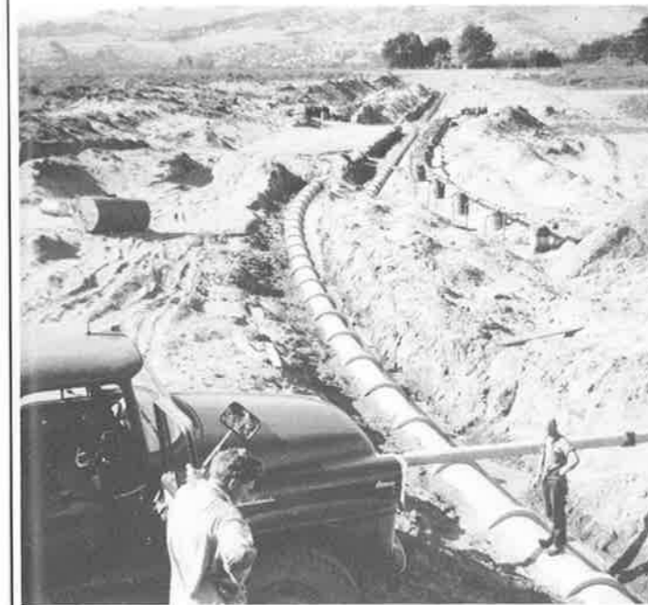
Above and right: Construction, in 1966, of the Number 15 rising main from the Number 15 pumping station in Woolston to the sewage treatment works in Bromley.
