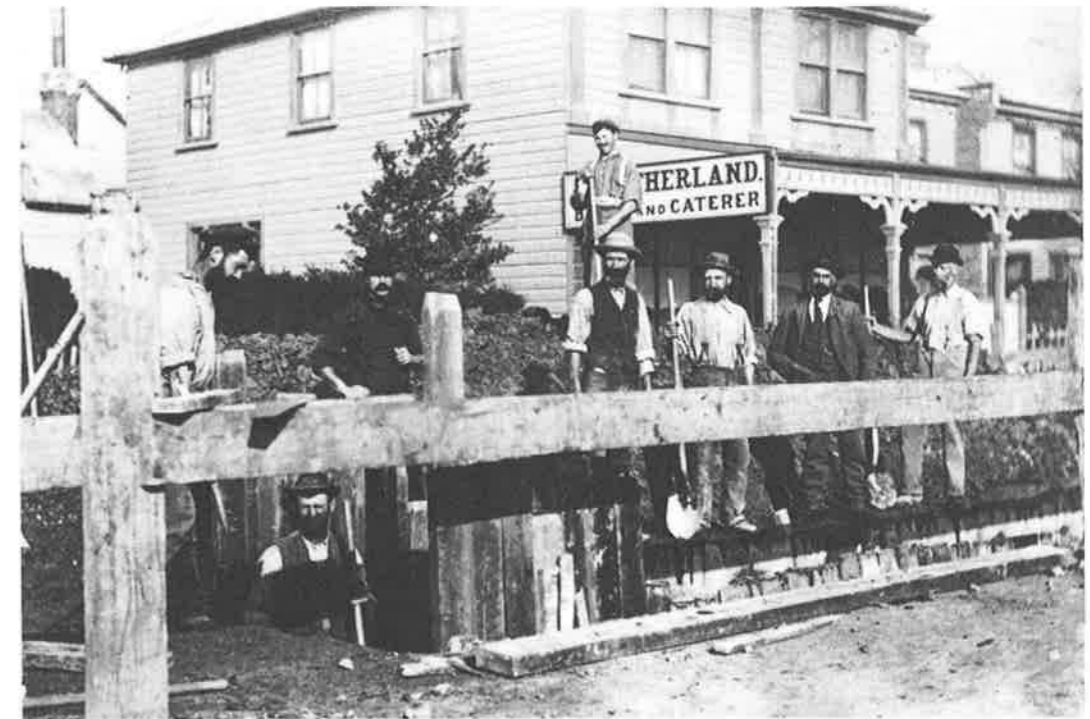
Sewer construction at the east end of Tuam Street, c. 1905. Drainage Board
