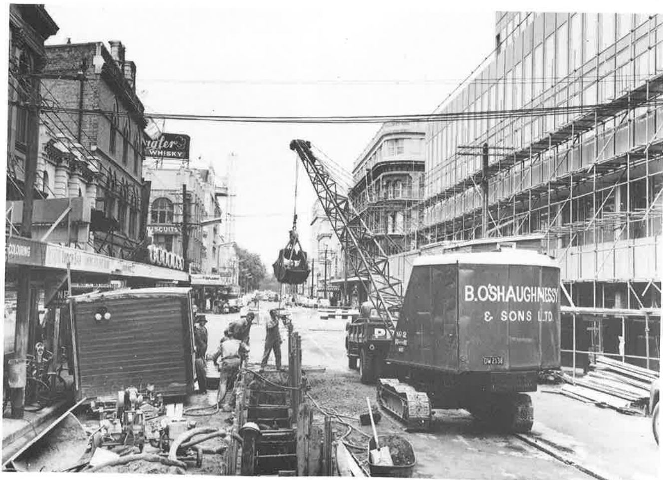
Right: A Drainage Board gang constructing a street sewer. The date of the photograph is uncertain, but is probably some time in the 1950s or early 1960s. Below: The central area relief sewer under construction along Hereford Street, 1966.
