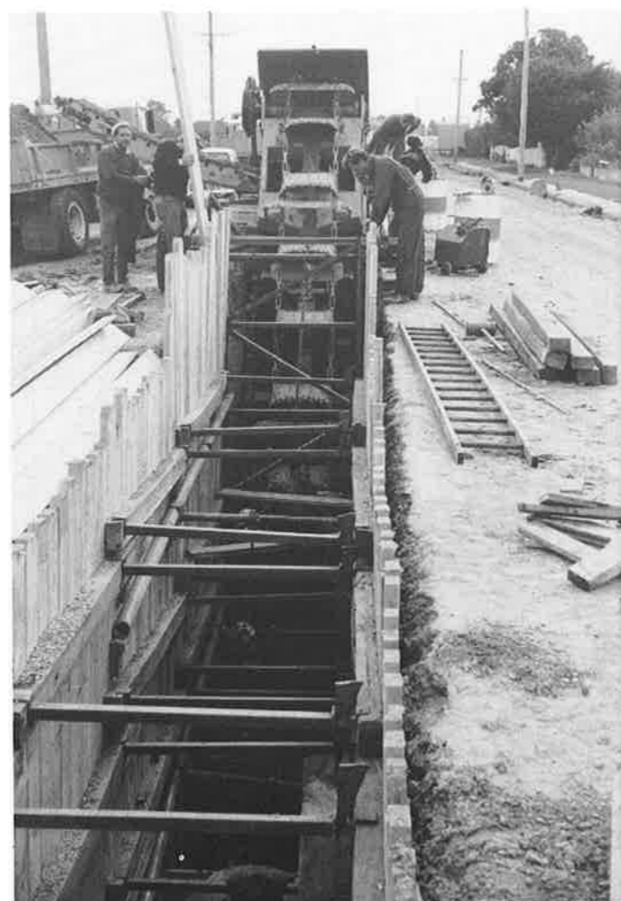
Sewer reticulation, Maces Road, 1969. Drainage Board
