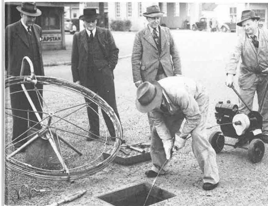
Left: Using a flexible rod to clear a blocked sewer. Below: The Board's inspectors, at the rear of the old Hereford Street offices, about to leave on their rounds to inspect household drainage and plumbing. The photograph was probably taken in the 1940s or 1950s.
