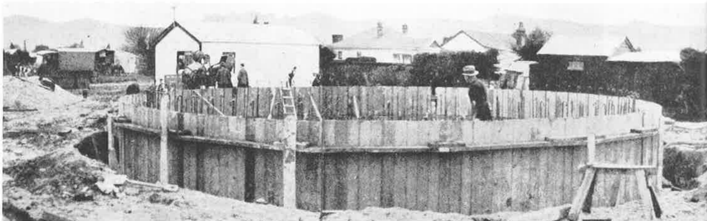
A sewage pumping station under construction in 1925. It is not clear which one this is of the several pumping stations under construction in that year. Weekly Press
