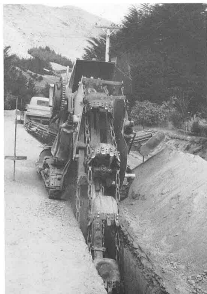
Sewer reticulation, Avoca Valley. Drainage Board
