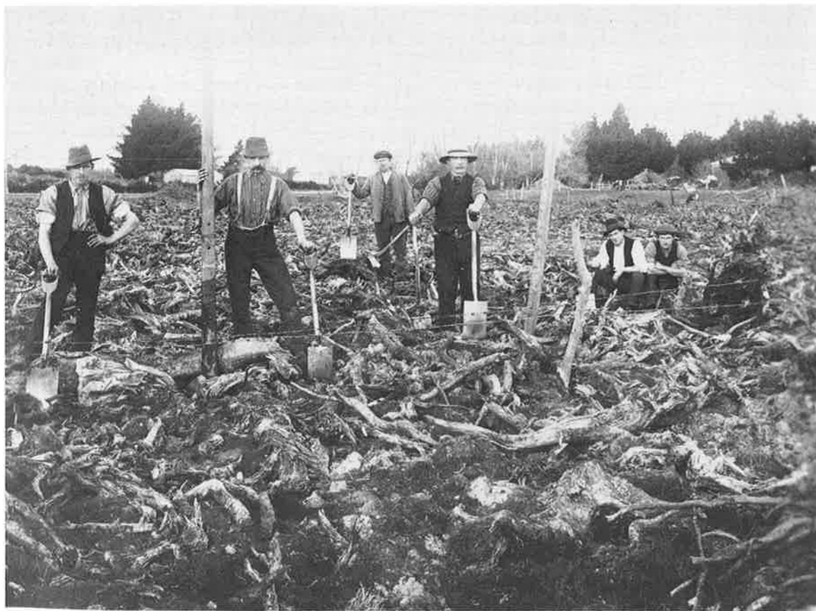
The difficult ground conditions encountered over much of Christchurch are evident in these 1918 photographs of land that was once covered by swamp forest.
