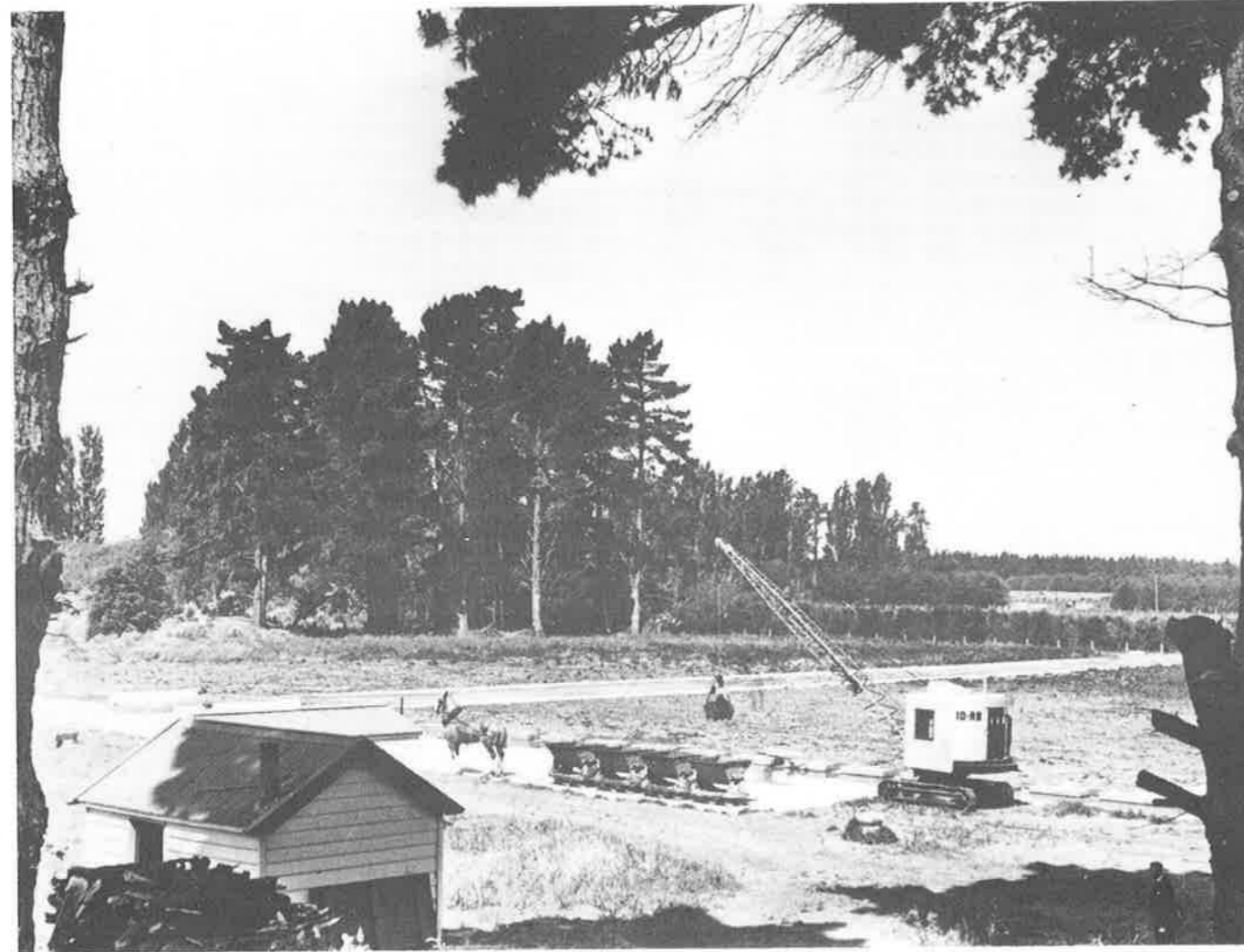
The last years of the old sewage farm. Above: Clearing out the septic tanks at the farm in 1945. Left: The sewage farm in 1957, just before construction of the new treatment works began. Both photos: Drainage Board
