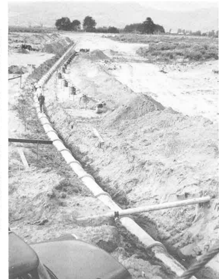
Above and right: Construction, in 1966, of the Number 15 rising main from the Number 15 pumping station in Woolston to the sewage treatment works in Bromley.
