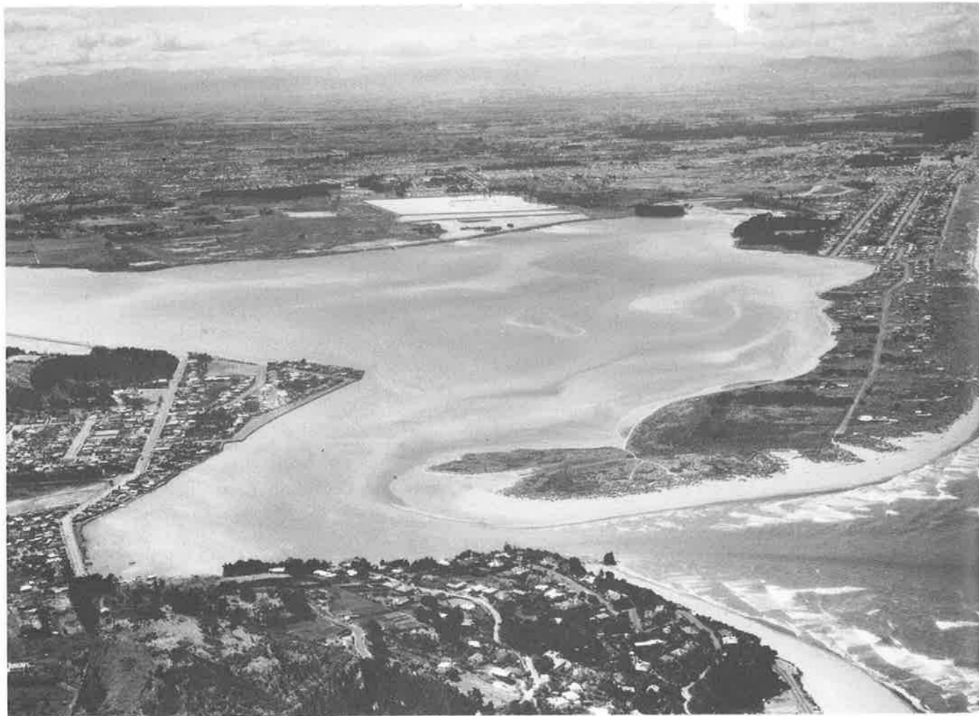
An aerial view of the Estuary, 1964, looking over its mouth to the oxidation ponds of the then-new treatment works at Bromley. Drainage Board
