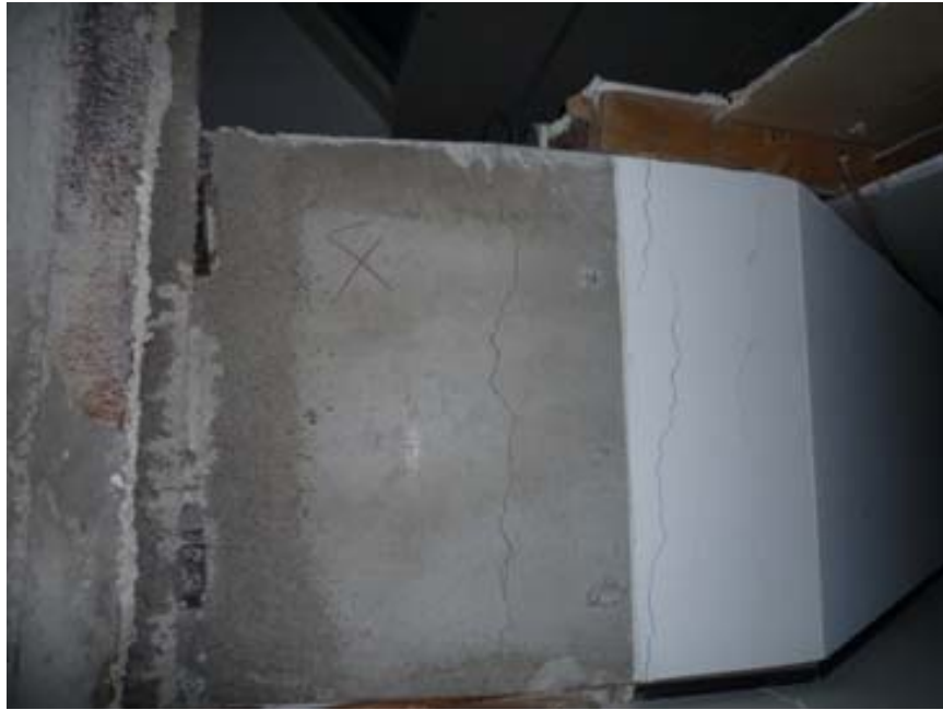
Figure A2.6.7: Level 16, South West Lobby, Looking up at Underside of North-West Unit Showing Cracking
