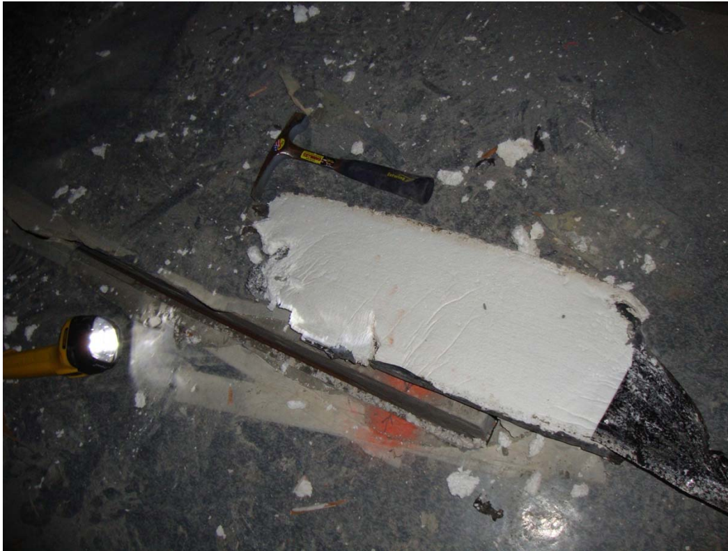
Figure A2.6.3: Level 16, North-East Landing, South-East Unit, Seismic Gap with 20 mm Polystyrene Sheet Infill Removed
