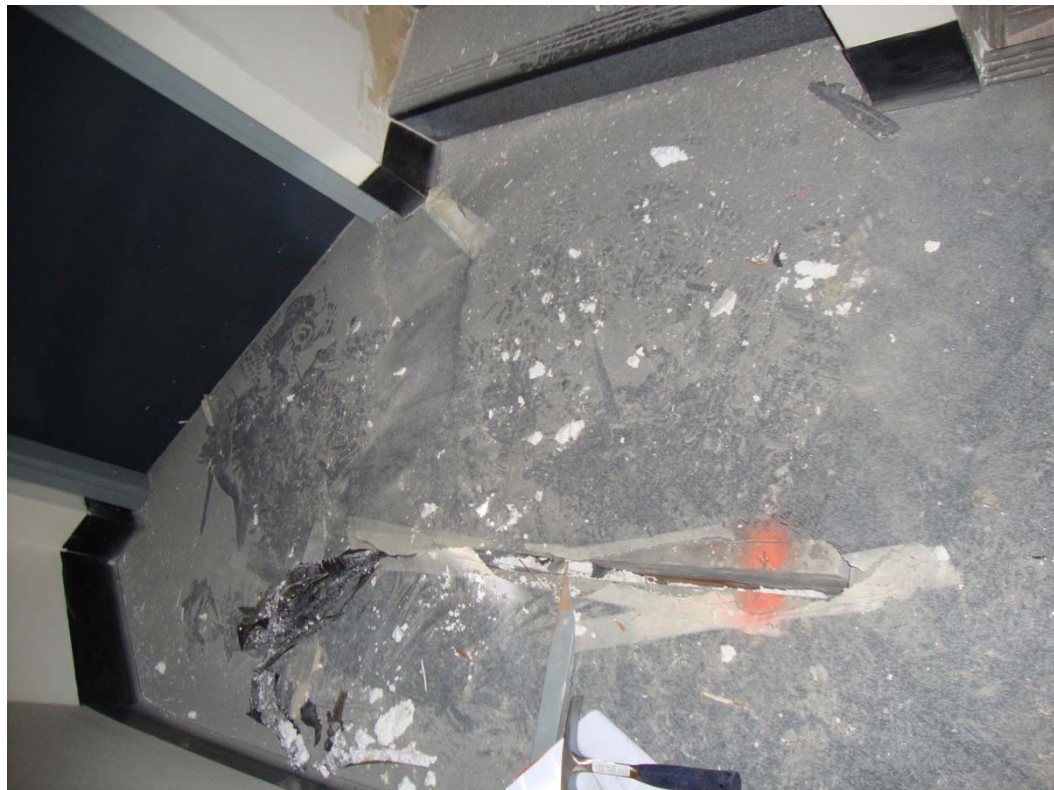
Figure A2.6.2: Level 16, North-East Landing, South-East Unit, Seismic Gap with 20 mm Polystyrene Sheet Infill
