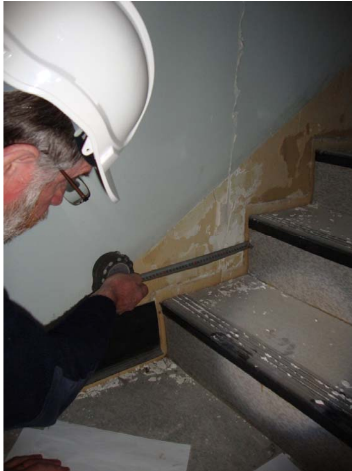
Figure A2.6.5: Level 16 : North-West Unit, South-West Landing – Relative Movement between Stair and North-West Wall (19 mm horizontally, 30 mm vertically)
