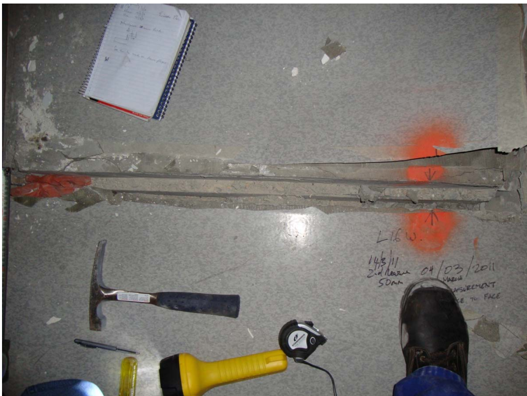
Figure A2.6.4: Level 16, South-West Lobby, North-West Unit, Seismic Gap with Stepped Landing
