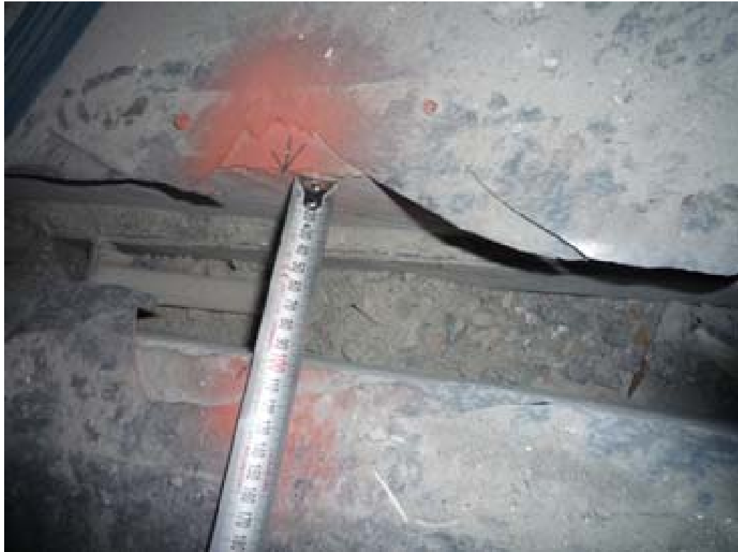
Figure A2.6.1: Level 15 North-West Unit, South-West Landing, Gap with 23 mm Removed off Unit
